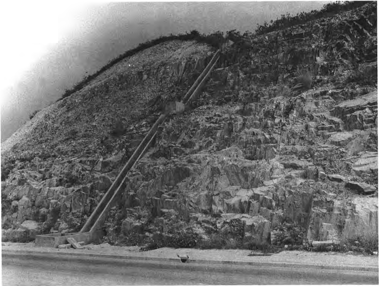
Plate 14. Rock Cut Slope in Coarse Tuff of the Repulse Bay Formation. Completely weathered material is evident at the top of the cut face. Weathering is more strongly developed to the left of the drainage channel. Vertical, closely spaced jointing with subsidiary horizontal joints give the outcrop a blocky appearance.
