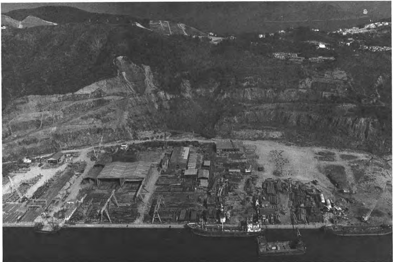
Plate 12. Aerial View of the Reclamation and Cut Slopes of Northeast Junk Bay. (GCO/OAP 1984/10039).
