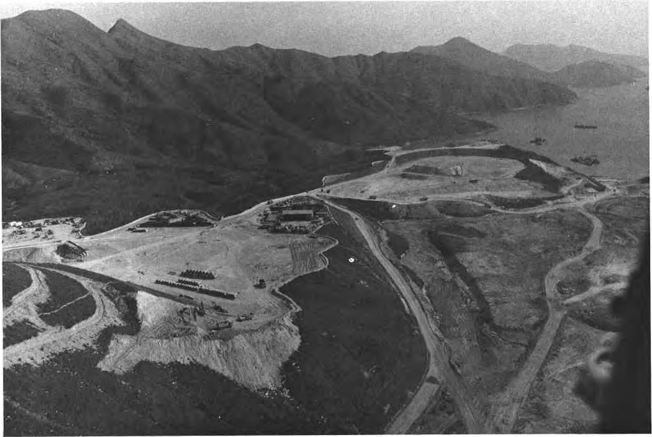
Plate 11. Aerial View of the Cut Platforms East of the Junk Bay Controlled Tip. The material extracted during the formation of the cut platforms is used to surround the layers of waste in the controlled tip. (GCO/OAP 1984/10044).
