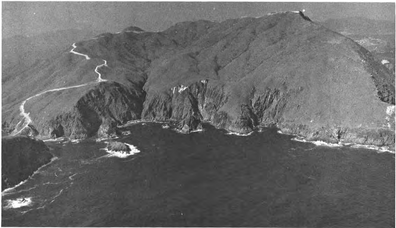
Plate 5. Aerial View of the Southern Coast of Tung Lung Island. Moderately sloping sideslopes are being subjected to basal undercutting by wave action. The resulting cliffs are prone to rockfalls and landslip activity that may extend up the sideslopes. (GCO/OAP 1984/9993).
