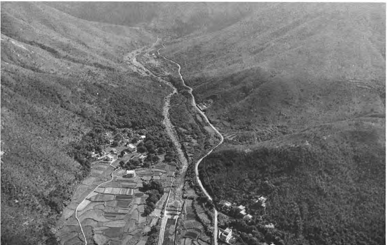
Plate 12. Oblique Aerial Photograph Looking South Towards Tung Chung Hang. Note the failure of insitu terrain on the western side of the Wong Lung Hang Road in the centre of the photograph (GCO/OAP 1981/4573).
