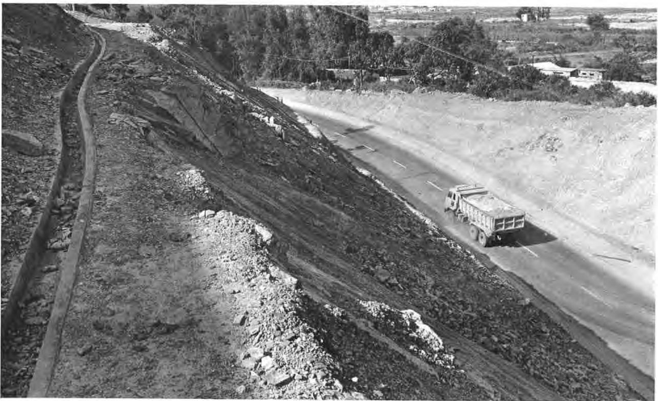
Plate 12. Shallow Cleavage and Joint-controlled Wedge and Planar Failures in a Large Cutting on the Lin Ma Hang Road to the North of Muk Wu. The cutting was constructed in steeply inclined phyllites of the Lok Ma Chau Formation.
