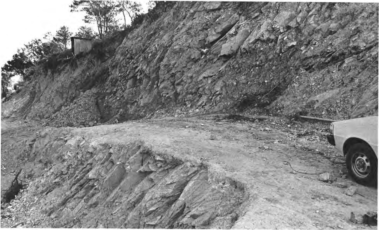
Plate 11. Phyllites of the Lok Ma Chau Formation Exposed in a Cutting for the Extension of the Lo Wu Railway Station. The phyllites display intense, closely spaced cleavage which dips consistently northeast and results in the highly fractured nature of the rock mass.
