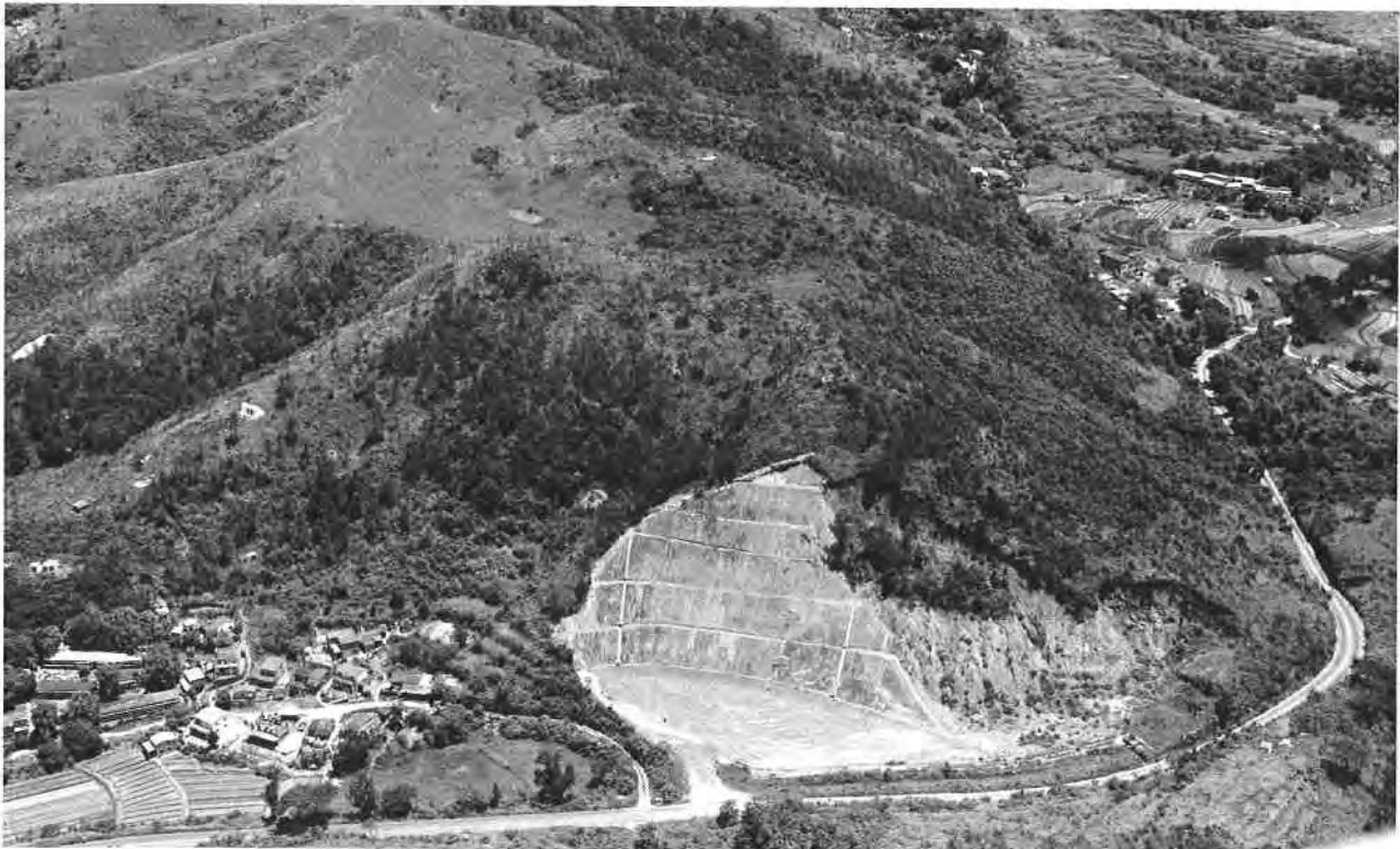
Plate 10. Large-scale Landslip in Weathered Volcanic Tuff of the Repulse Bay Formation. The cut slope lies to the north of the Sha Tau Kok Road at Au Ha at the Four Mile milestone (GCO/OAP 1981/5364).
