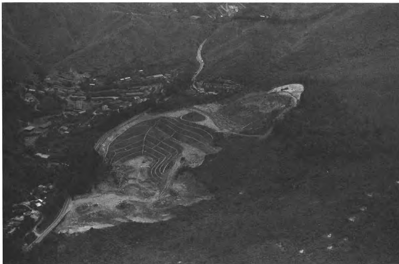
Plate 8. Oblique Aerial Photograph of the Eastern End of the Shek Kong Valley near Kadoorie Farm. A large landslip affects the upper part of the construction zone. A tension crack is evident in the chunamed cut slope at the upslope margin of the site. (GCO/OAP 1979/584).
