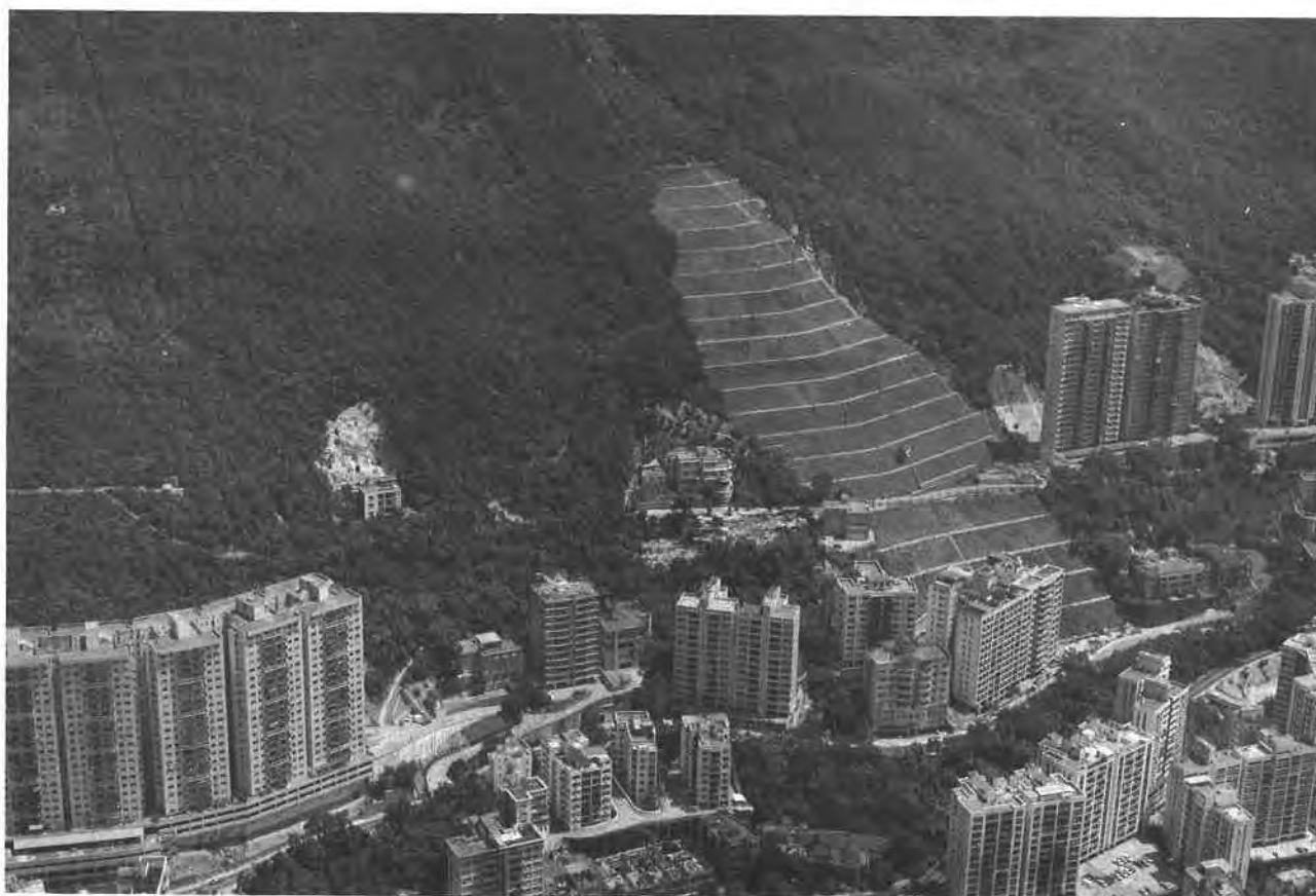
Plate 9. Oblique Aerial Photograph of the Po Shan Road Landslip after Remedial Works.
