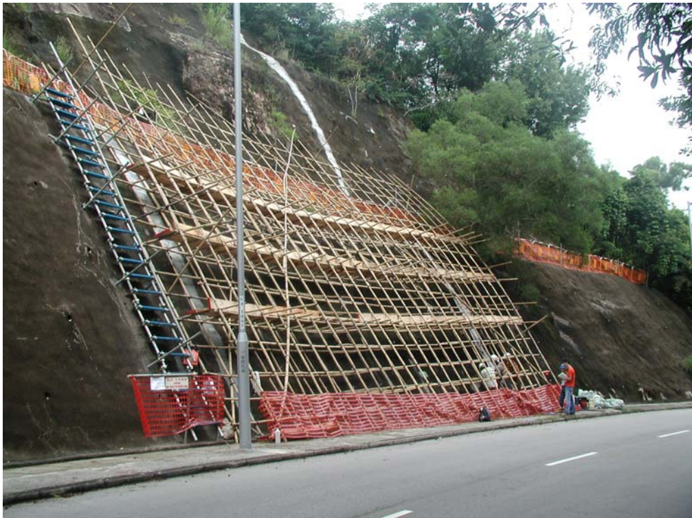
Plate 6 - View of Section of Slope No. 3NE-B/C82 Surveyed Using the Sympathetic Vibration Technique and Confirmatory Coring
