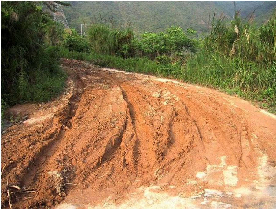
Plate 17 - View of the Landslide Debris Washed Down the Access Road by Subsequent Overland Flow (Photograph taken on 9 May 2003)
