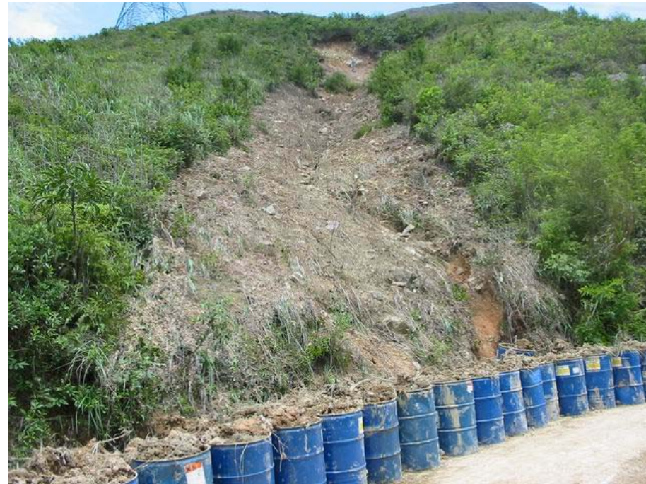
Plate 16 - View of the Debris Trail and Source Area from the Access Road (Note the incised gully on the right side. Photograph taken on 16 May 2003)
