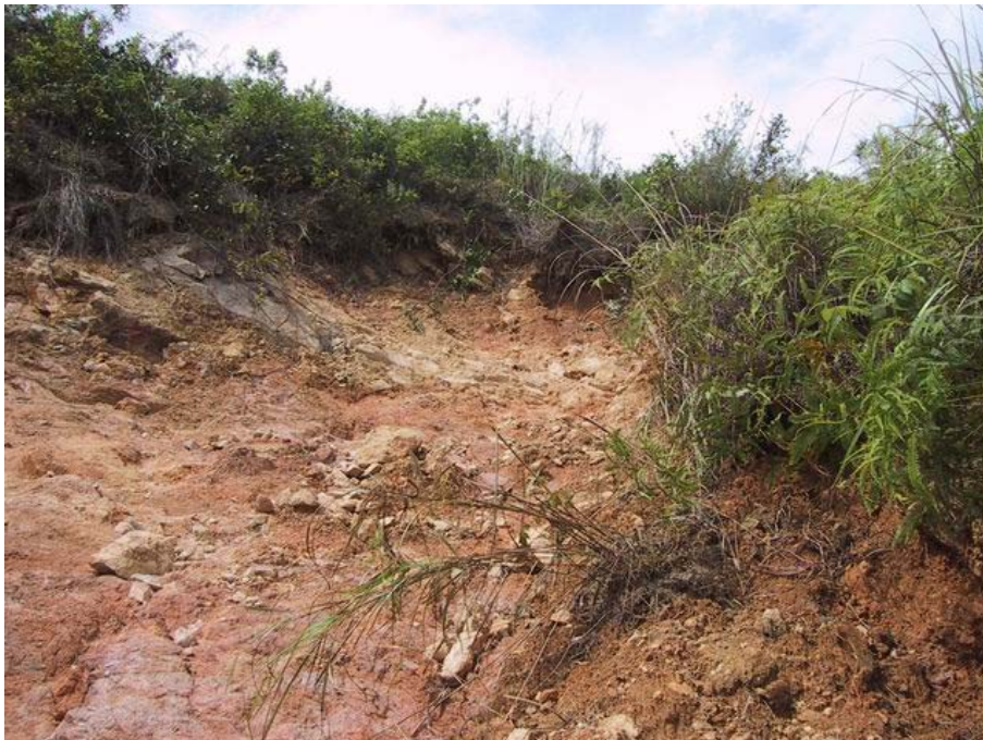
Plate 6 - View of the Eastern Portion of the Main Scarp (Note the persistent band of metamorphosed siltstone. Photograph taken on 16 May 2003)
