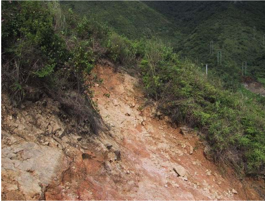
Plate 7 - View of the Eastern Flank of the Source Area (Note the relatively clean surface of rupture with overlying colluvium exposed at the scarp. Photograph taken on 16 May 2003)
