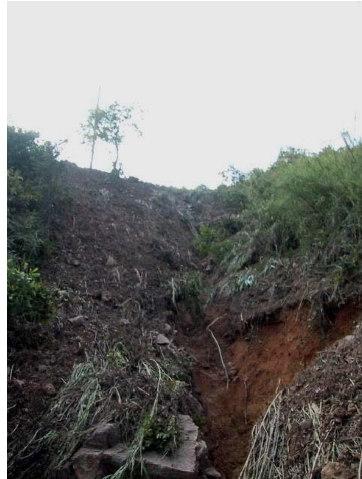
Plate 24 - View Looking Upslope from Chainage CH 82 (Note the minor failure of the eastern flank of the drainage line. Photograph taken on 9 May 2003)
