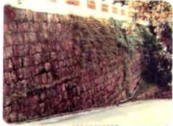
Plate 4 - Dry Packed Squared Rubble Wall with Horizontal Beams (11SW-A/R163)
