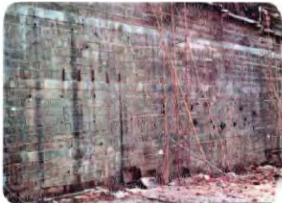
Plate 10 - Tied Face Wall with Horizontal Beams (11SW-A/R45)
