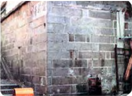
Plate 9 - Tied Face Wall (11SW-A/R74)
