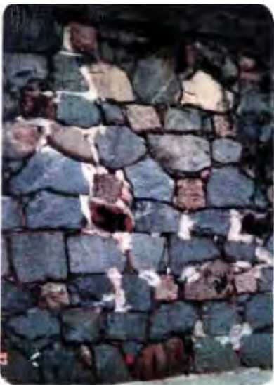
Plate 11 - Random Rubble Wall with Stone Ties
