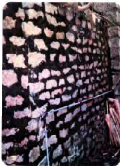
Plate 10 - Tied Face Wall with Horizontal Beams (11SW-A/R45)
