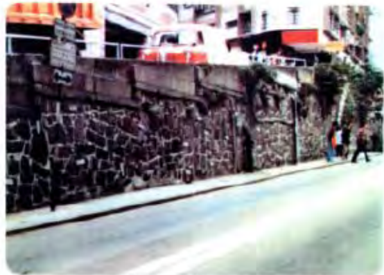
Plate 2 - Pointed Random Rubble Wall (11SW-A/R116)
