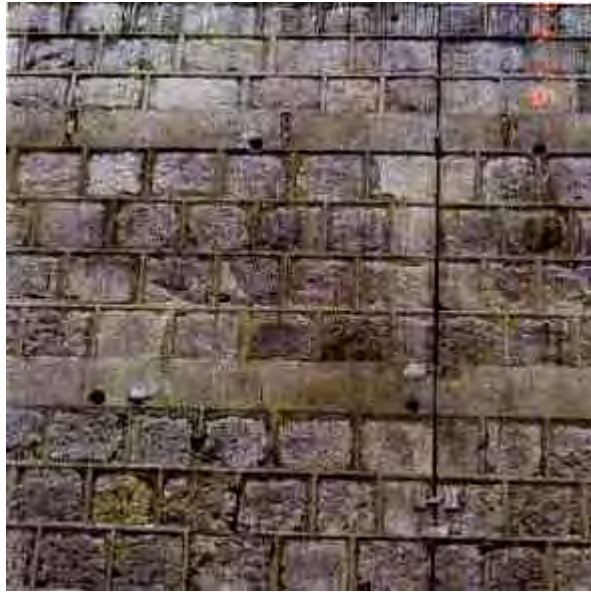
Plate 13 - Presence of Expansion Joints or Similar Construction Joints
