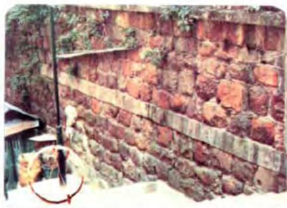
Plate 6 - Pointed Squared Rubble Wall with Horizontal Beams (11SW-A/R194)
