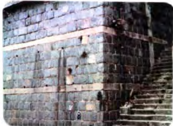
Plate 8 - Dressed Block Wall with Horizontal Beams (11SW-A/R423)
