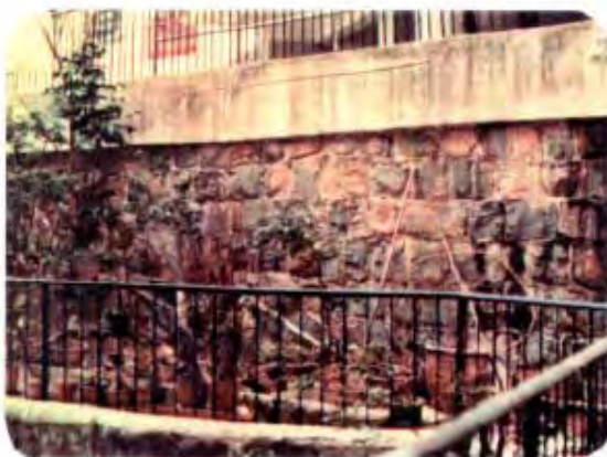
Plate 5 - Pointed Squared Rubble Wall (11SW-A/R295)
