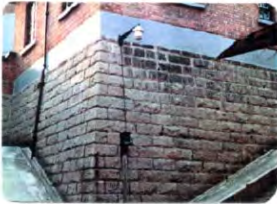
Plate 7 - Dressed Block Wall (11SW-A/R46)
