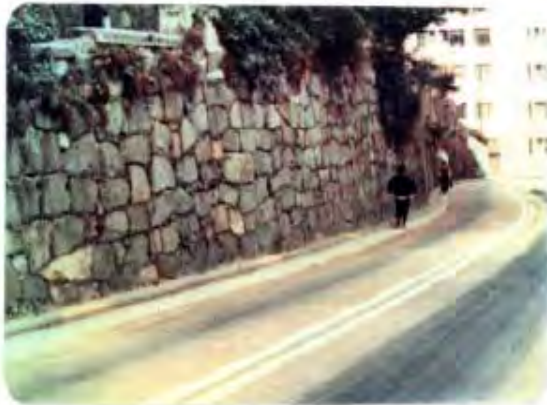
Plate 1 - Dry Packed Random Rubble Wall (11SW-A/R389)
