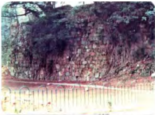
Plate 3 - Dry Packed Squared Rubble Wall (11SW-A/R109)
