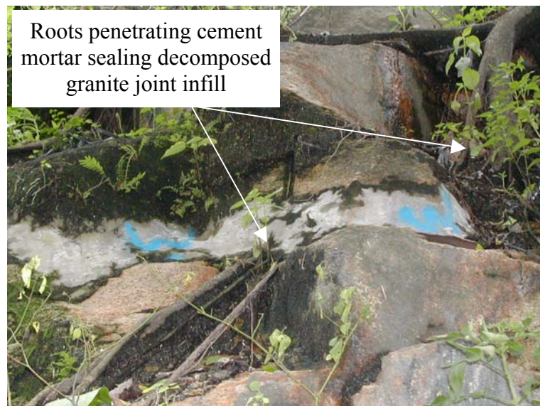
Plate 9 - Wide Sub-horizontal Joints Sealed with Cement Mortar to Prevent Erosion of Weak Weathered Granite Infill Material (Photograph taken on 17 June 2003)
