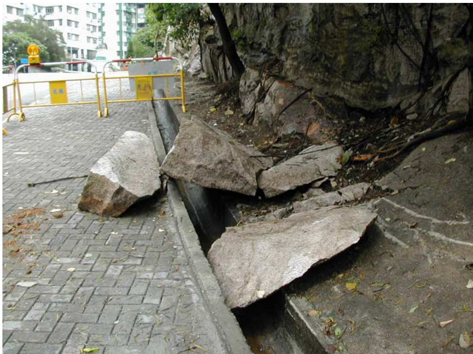
Plate 3 - View of the Detached Granite Blocks from the 6 June 2003 Rockfall (Photograph taken on 7 June 2003)
