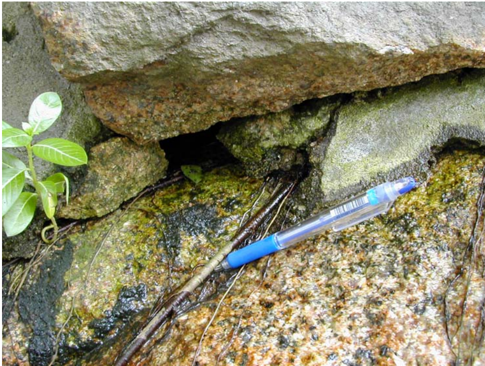
Plate 12 - Close-up View of Seepage at the Eastern Portion of the Rock Slope (Photograph taken on 17 June 2003)
