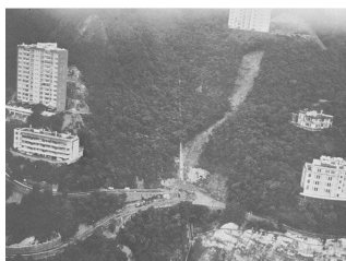
Plate (b) - Hillside failure at junction of Magazine Road and May Road
