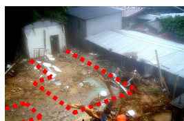
Plate (c) - Houses demolished by the debris flow
