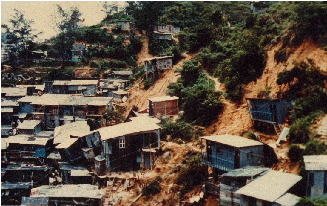
(a) Landslide covering a large area, where small cuttings and pockets of fill materials are present
