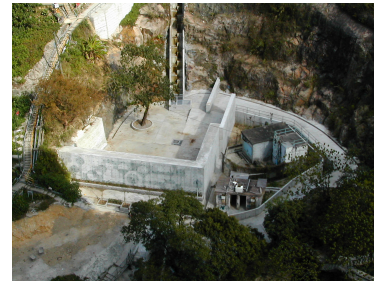
Plate (c) - Check dam constructed after the debris flow
