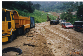
Plate (c) - debris deposited on the access road
