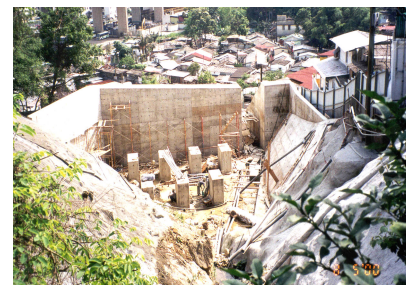
Plate (d) - Check dam constructed to protect the village from future debris flows
