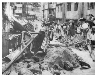
Plate (e) - Debris flow reaching North Point due to washout from Braemar Reservoir
