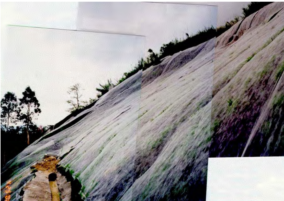
Plate 9 - View of Slope No. 6NE-B/C8 in April 2000 (Photograph taken by ESA Consulting Engineers Ltd on 25 April 2000)
