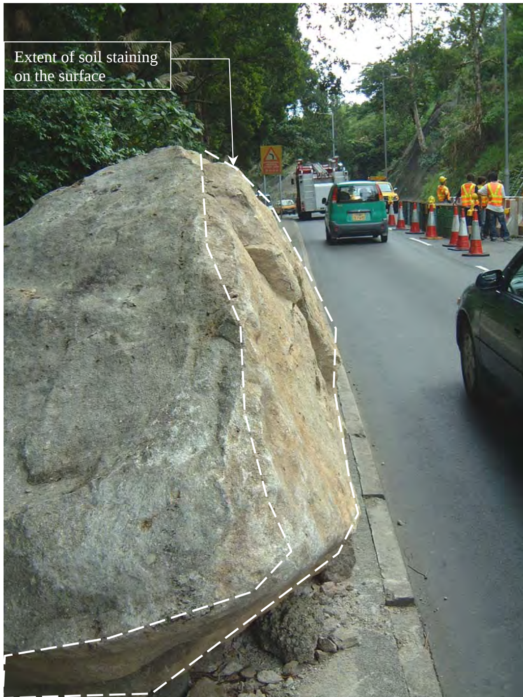
Plate A4 - Close-up View of the Fallen Boulder (Photograph taken on 16 May 2003)
