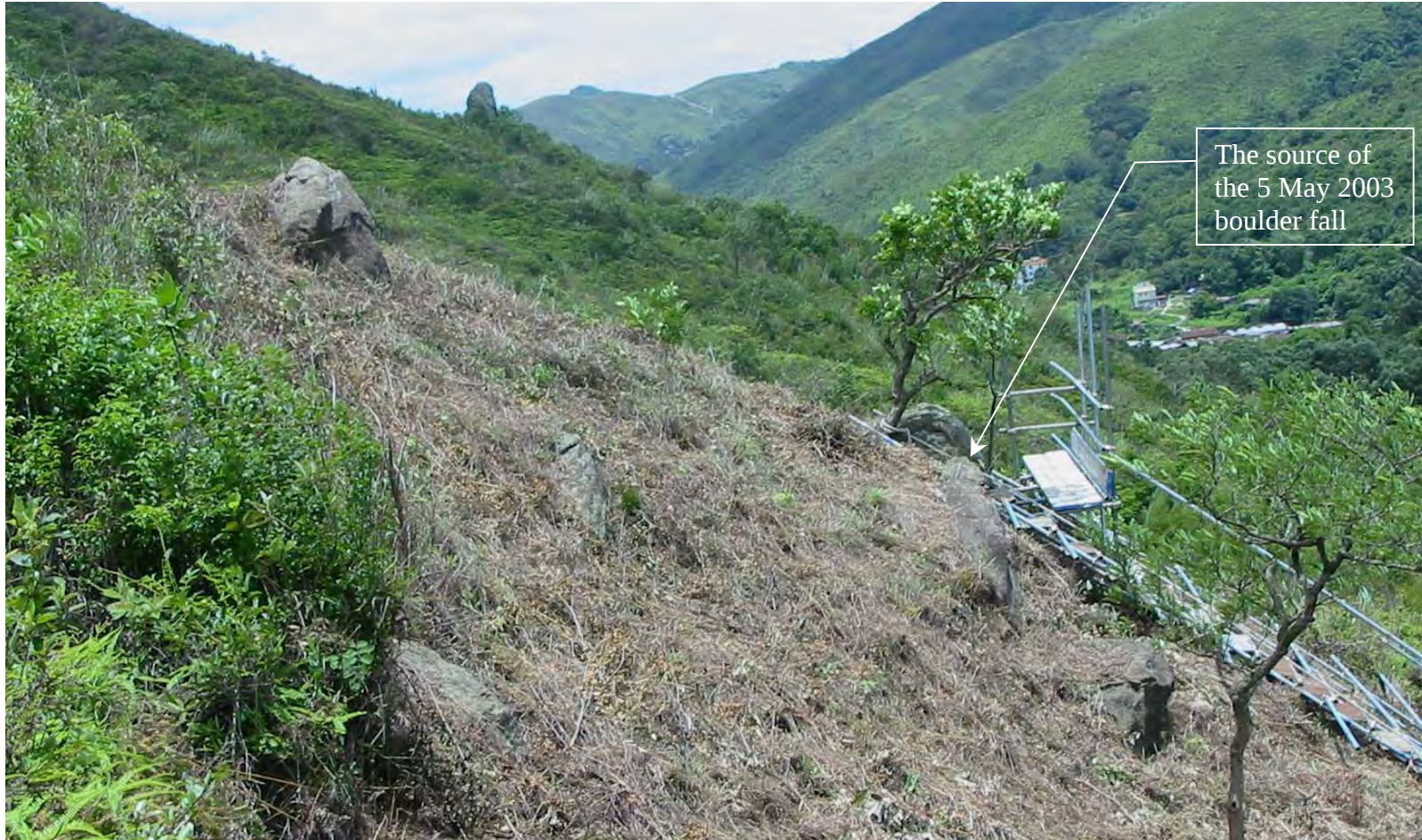
Plate A3 - Side View of the Natural Hillside above the Source of the 5 May 2003 Boulder Fall after Vegetation Clearance (Photograph taken on 16 May 2003)
