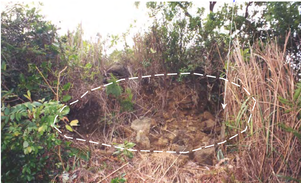
Plate A5 - View of the Source of the 5 May 2003 Boulder Fall (Photograph taken on 6 May 2003)
