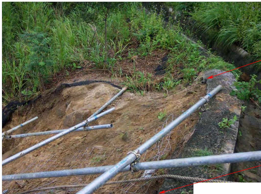
Plate 6 - View of Remnants of Erosion Control Mat around the Crest of the 5 May 2003 Landslide Site (Photograph taken on 14 June 2003)
