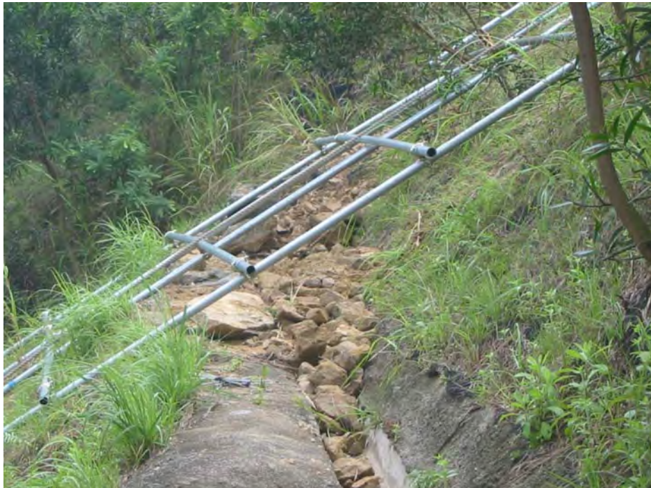
Plate 5 - View of the 1 m Wide Berm on Slope No. 6NE-B/C8 (Photograph taken on 6 May 2003)
