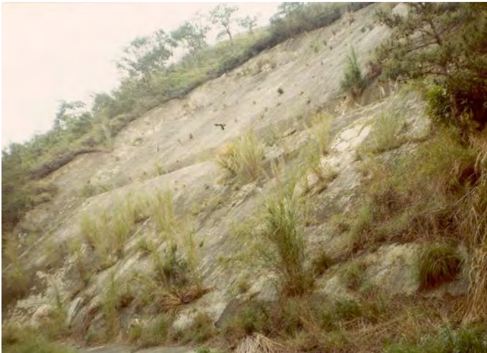
Plate 8 - General View of Slope No. 6NE-B/C8 in 1978 (Photograph taken by Binnie & Partners (Hong Kong) on 18 April 1978)
