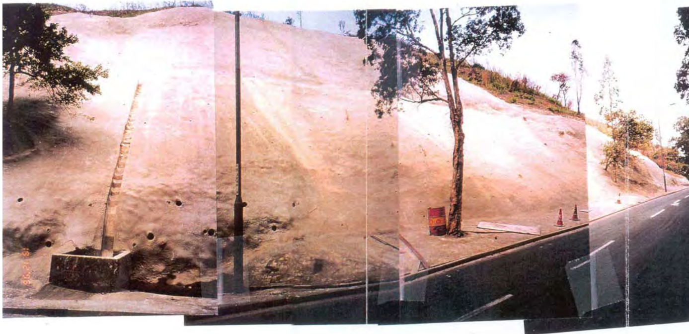
Plate 10 - View of Slope No. 6NE-B/C8 in December 1996 (Photograph taken by ESA Consulting Engineers Ltd on 19 December 1996)
