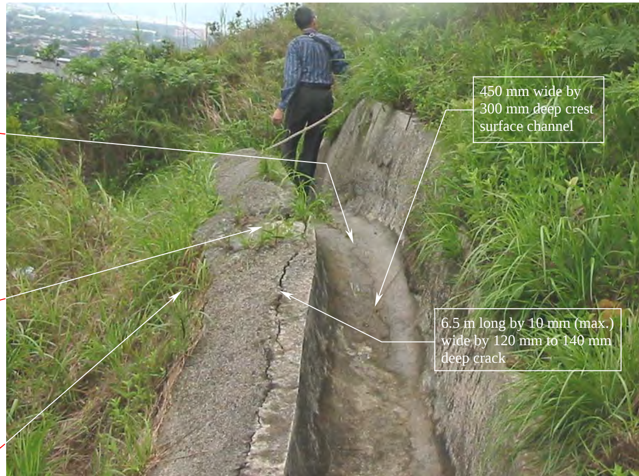
Plate 7 - View of the Surface Drainage Channel along the Crest of Slope No. 6NE-B/C8 (Photograph taken on 6 May 2003)
