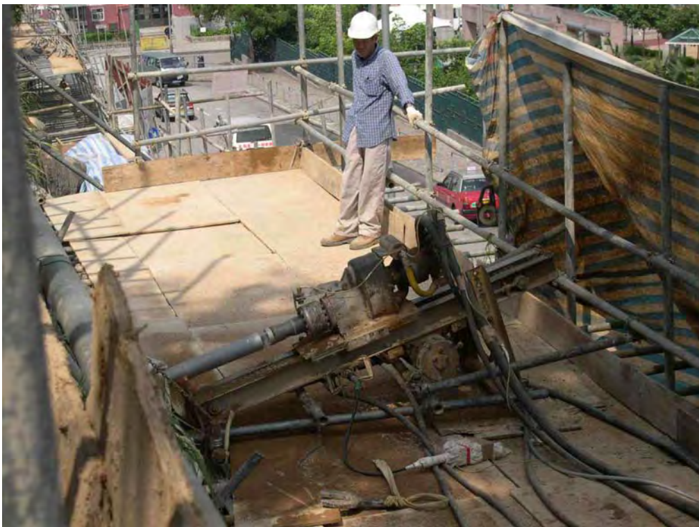
Plate 2 - Air-driven Rotary Percussive Down-the-hole Drilling Machine Used at the Site
