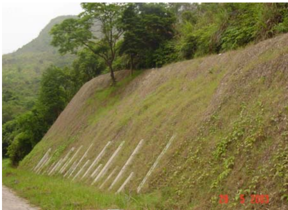
Overall view of slope treated with CMS-ML Green System
