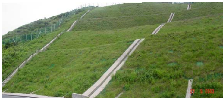
Overall view of slope applied with Multimat
