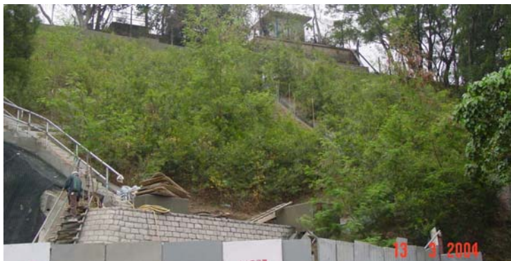
Overall view of slope applied with Enkamat
