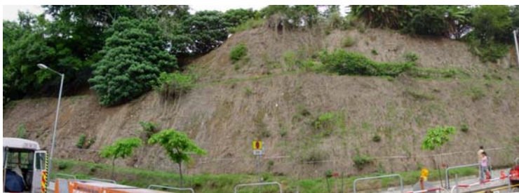
Overall view of slope treated with NFY Hydro-Mulching
