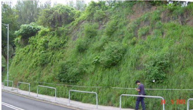
Overall view of slope treated with Eco-link
