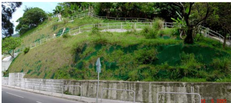
Overall view of slope applied with Miramat TM8
