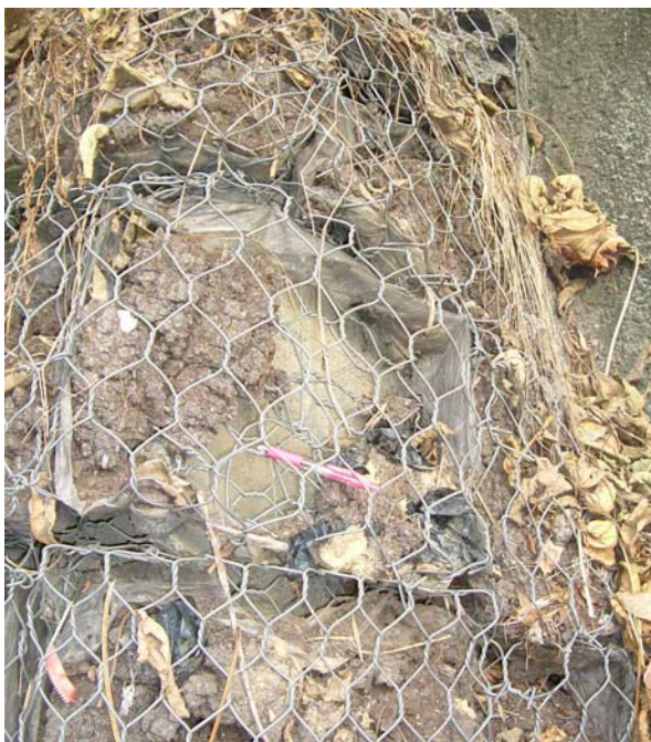
Plate 13 - Sign of Distress Observed on Slopes with NFY Mulching Panel
