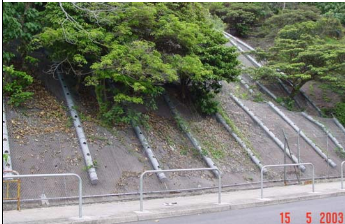
Overall view of slope treated with NFY Hydro Planter
