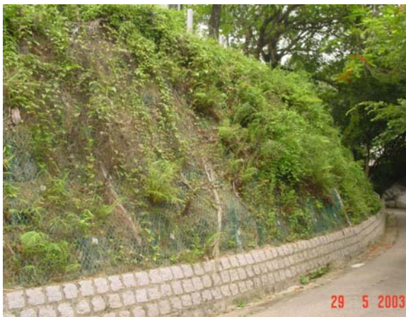
Overall view of slope applied with Enkamat and Steel Wire Mesh
