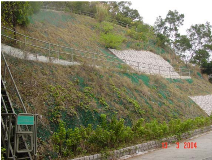
Overall view of slope applied with Miramat TM8 and Steel Wire Mesh
