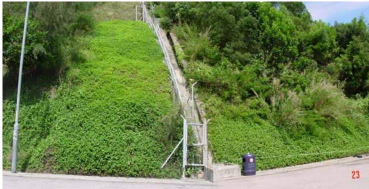
Overall view of slope treated with Toyo-Mulching
