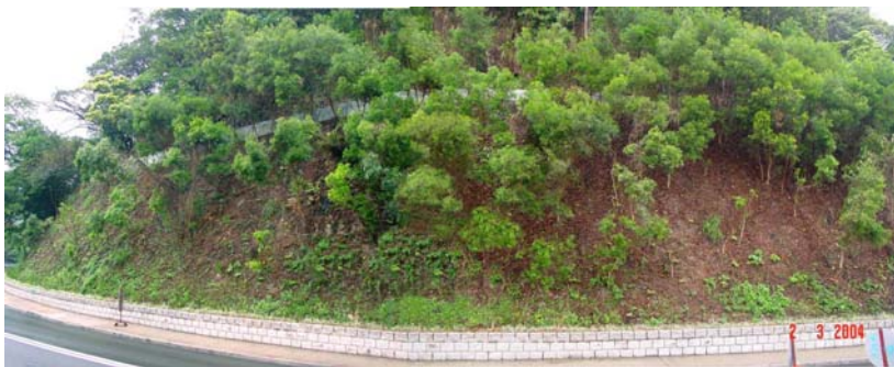
Overall view of slope applied with Tensarmat/EM4
