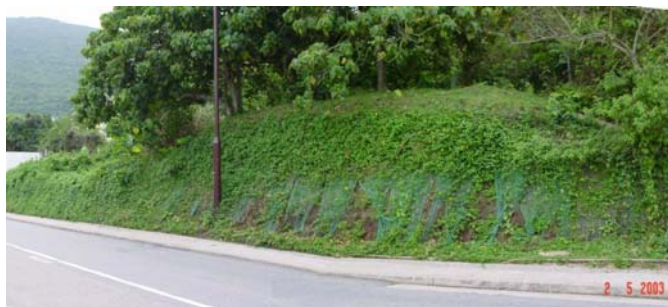
Overall view of slope treated with Hong Kong Mulching
