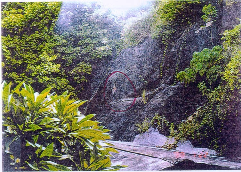
Plate A11 - Cracked Chunam on the Central Portion of the Slope above the Temple Taken on 22 July 1998 (Reproduced from Atkins China Ltd., 1998). Note that these cracks were also observed after the 1999 Landslide and appeared to have opened up.
