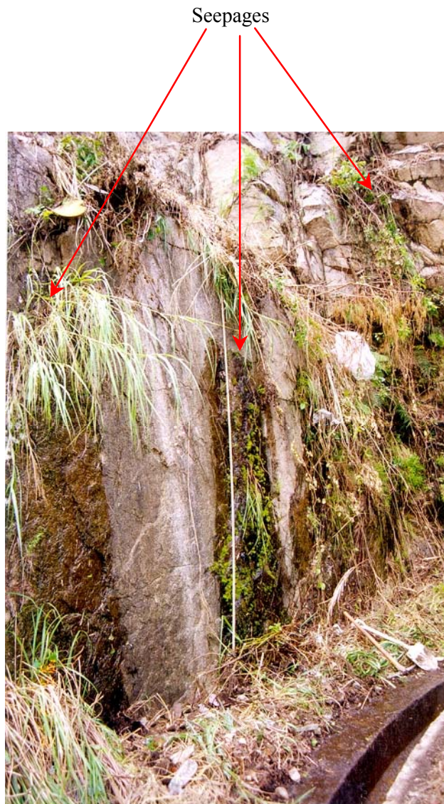
Plate 27 - Seepage at the Rock Outcrop at the Toe of Slope No. 11NW-B/C91. (Photograph Taken on 8 September 1999). See Figure 34 for location.
