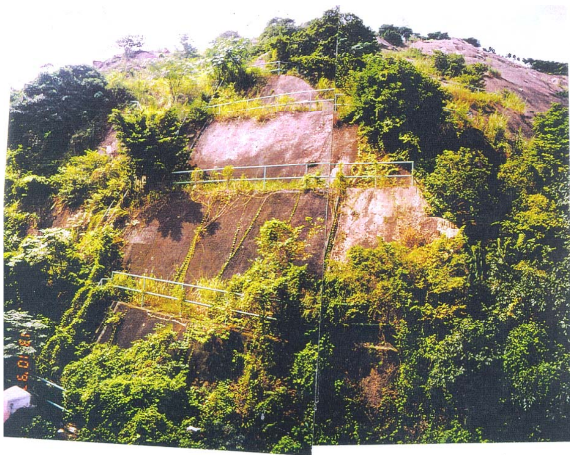
Plate A10 - General View of the Northern Portion of Slope No. 11NW-B/C90 Taken on 13 October 1997 (Reproduced from Atkins China Ltd., 1997). Note the extent of chunam with dark tone and dense unplanned vegetation on the slope.
