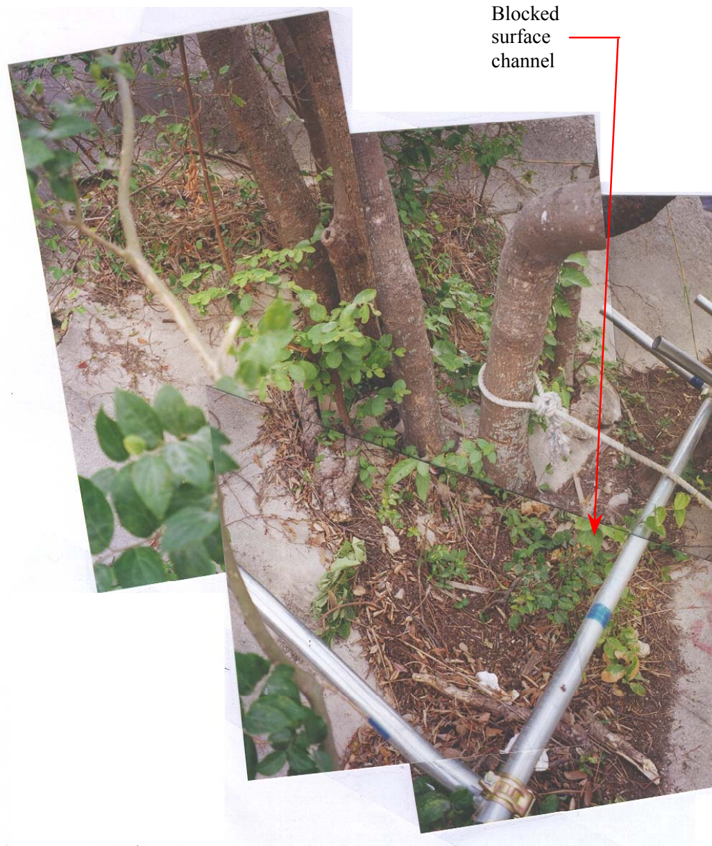
Plate 29 - Unplanned Tree Blocking Surface Channel (Photograph Taken on 9 November 1999). See Figure 34 for location.
