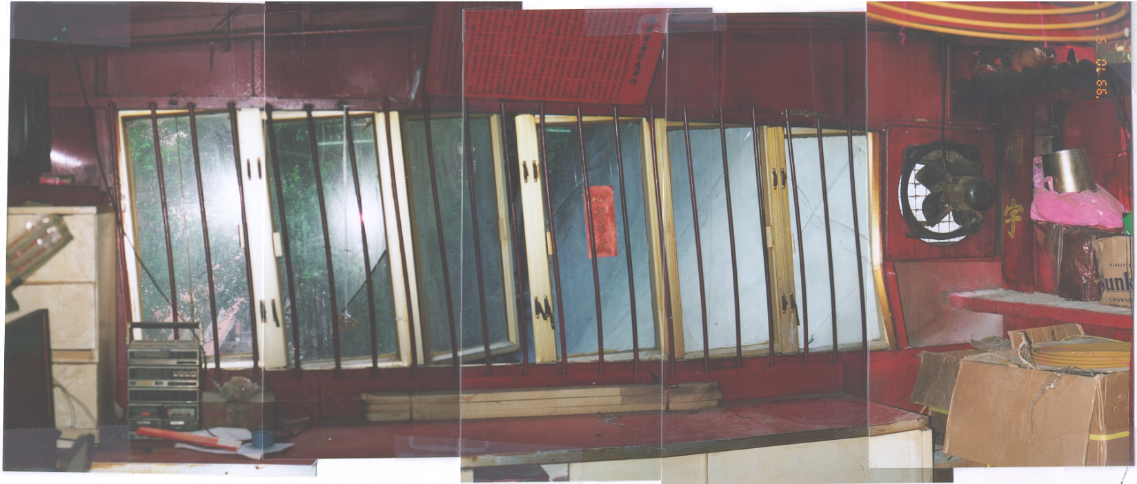
Plate 15 - Tilting of the Window Frames at the Temple (Photograph Taken on 9 October 1999). See Figure 34 for location.
