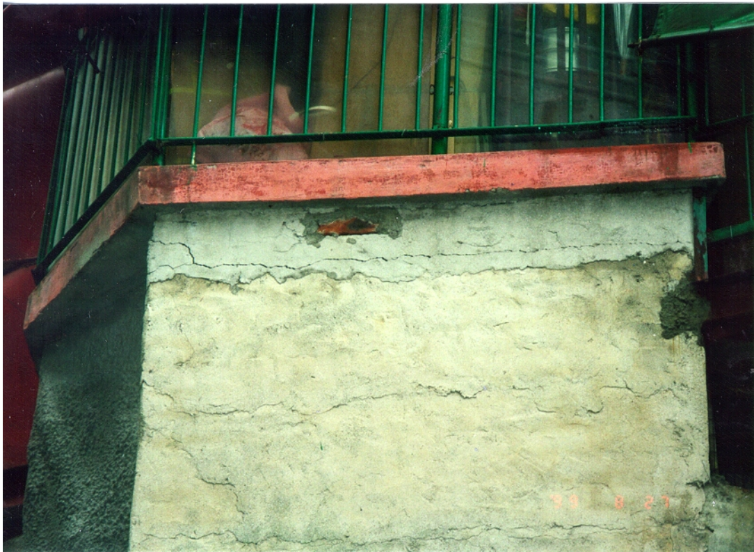
Plate 14 - Horizontal Crack in a Concrete Pier Supporting the Temple Structure (Photograph Taken on 27 August 1999). See Figure 34 for location
