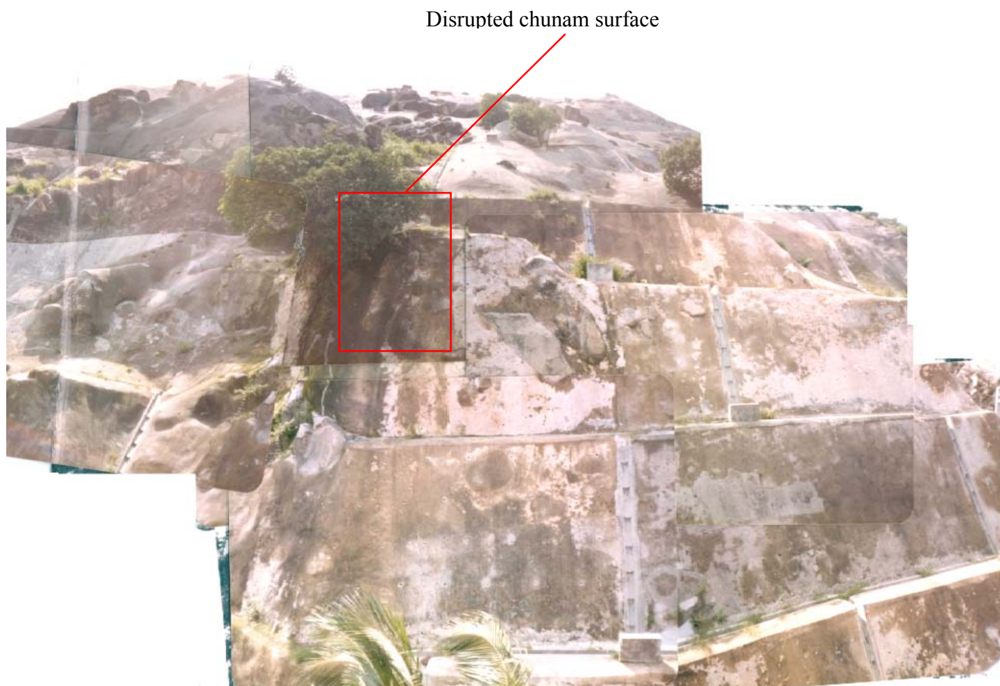
Plate A4 - General View of the Northern and Central Portions of Slope No. 11NW-B/C90 Taken on 4 June 1982 (Reproduced from B&P, 1982). Note the disrupted chunam, patches of repaired chunam and chunam with dark tone on the slope surface.
