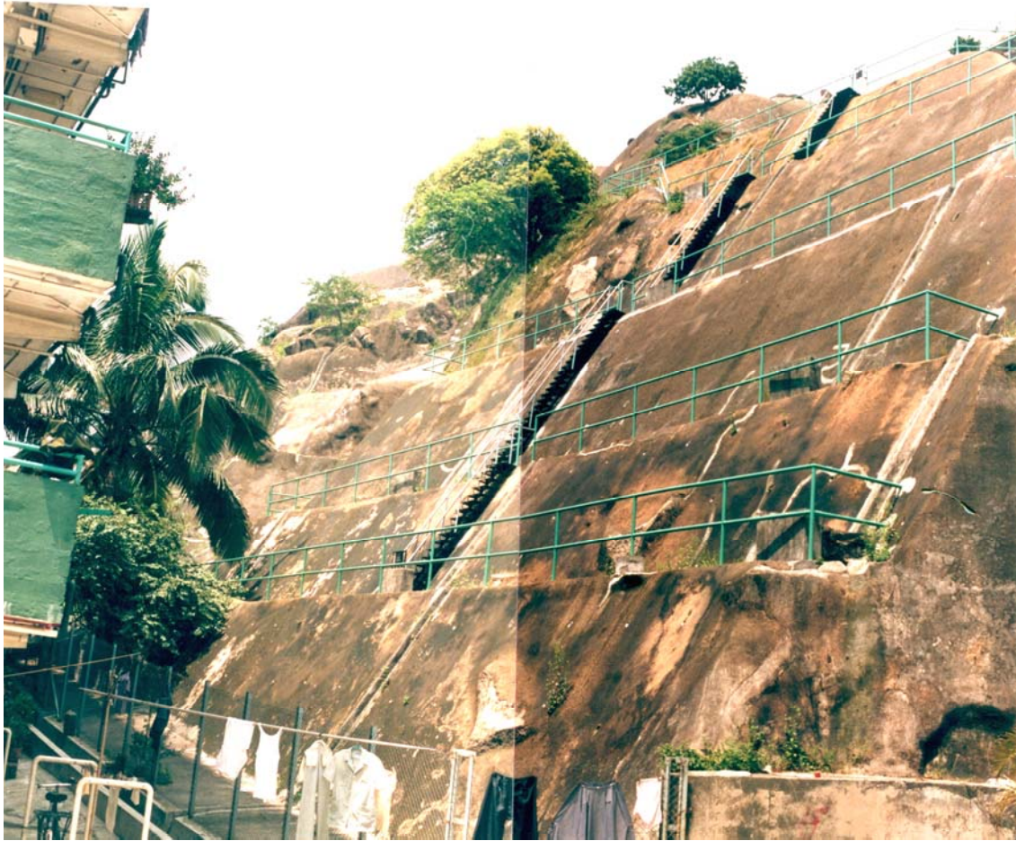
Plate A8 - General View of the Lower Northern Portion of Slope No. 11NW-B/C90 Taken on 14 August 1986 (Reproduced from Dames & Moore, 1986). Note the repaired chunam and sealed cracks on the slope.
