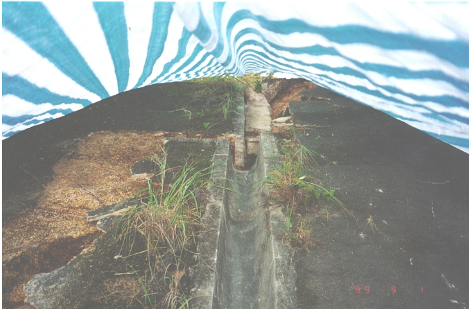
Plate 12 - Right Lateral Displacement across a Drainage Channel (Photograph Taken on 1 September 1999). See Figure 34 for location
