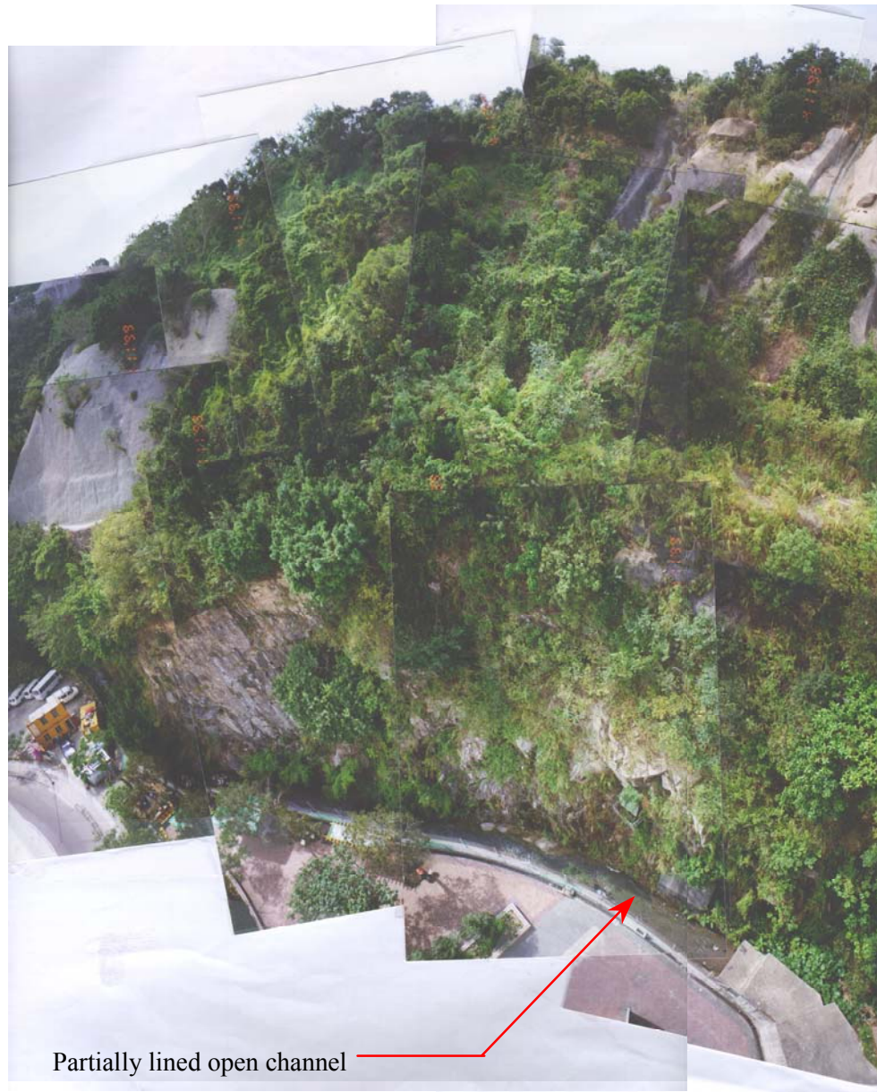
Plate 4 - View of Slope No. 11NW-B/C582 and the Partially Lined Open Channel along the Toe (Photograph Taken on 4 November 1999). See Figure 34 for location
