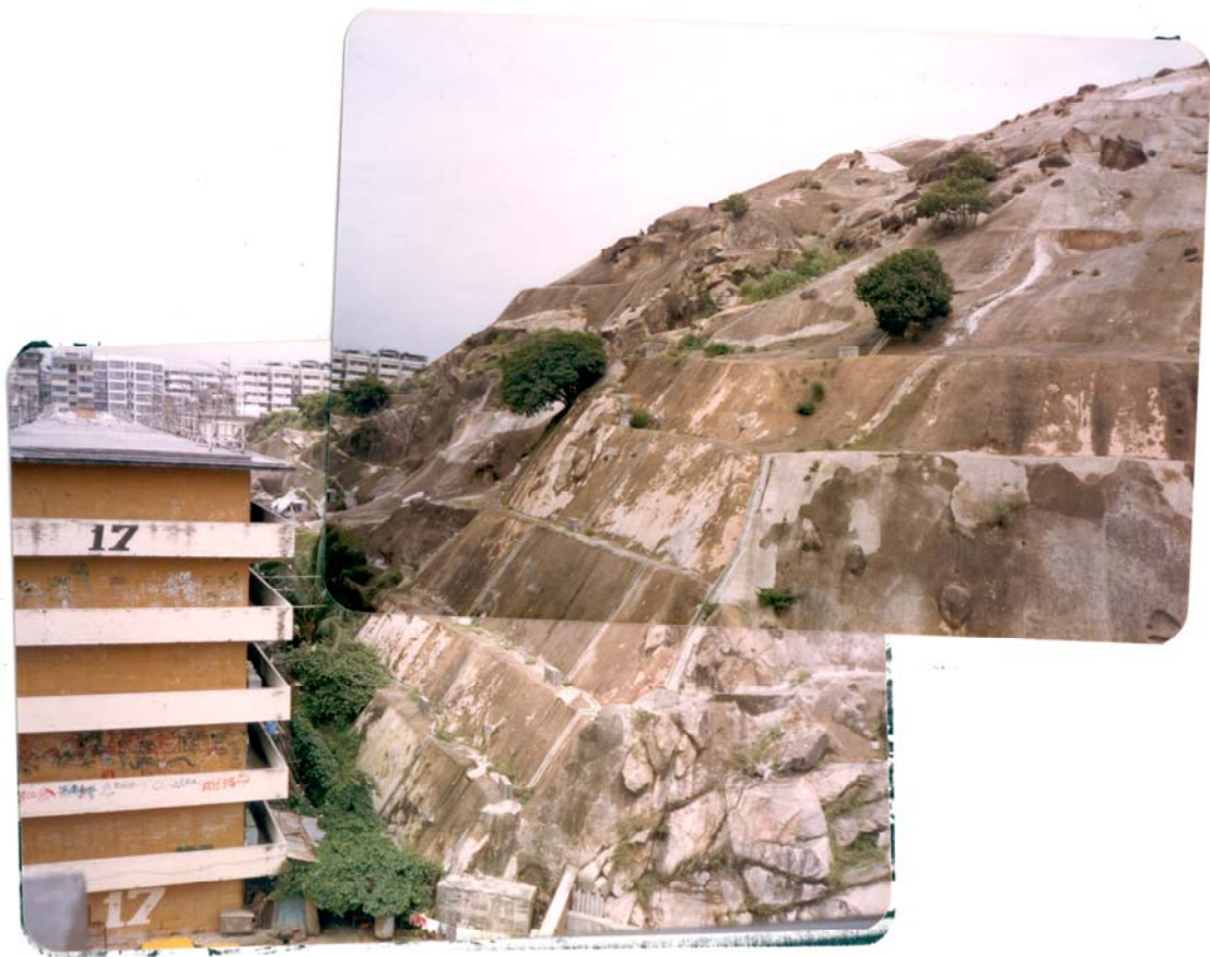
Plate A3 - General View of the Northern Portion of Slope No. 11NW-B/C90 Taken on 4 June 1982 (Reproduced from B&P, 1982). Note patches of repaired chunam on the slope surface.
