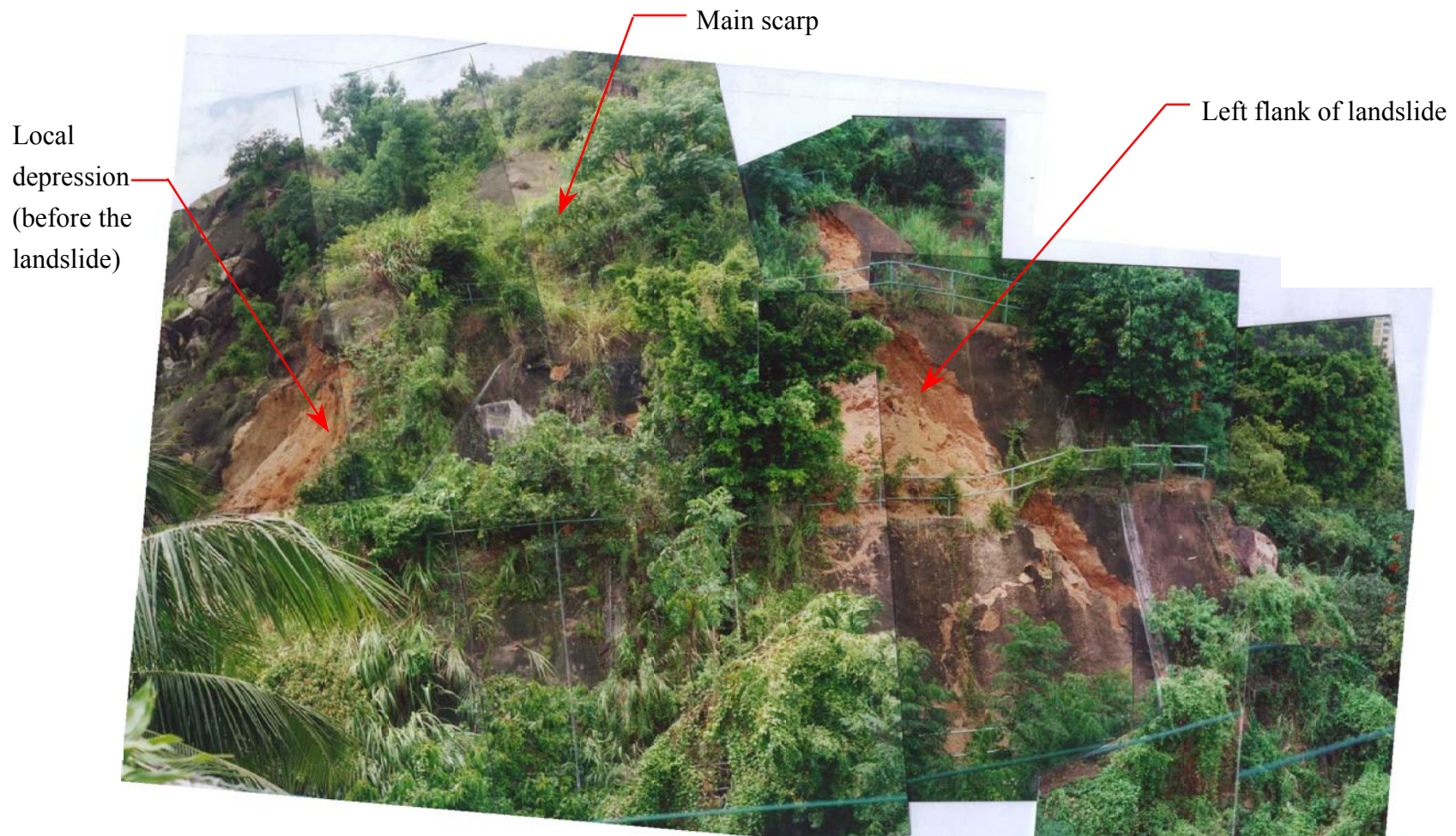
Plate 6 - General View of the Northern Distressed Zone (Photograph Taken on 26 August 1999). See Figure 34 for location.
