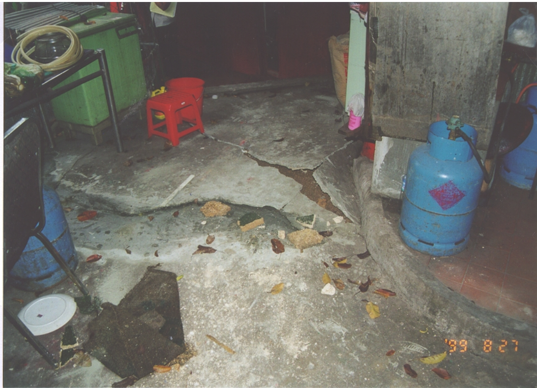
Plate 13 - Cracking and Heaving in the Concrete Platform to the Northeast of the Temple (Photograph Taken on 27 August 1999). See Figure 34 for location
