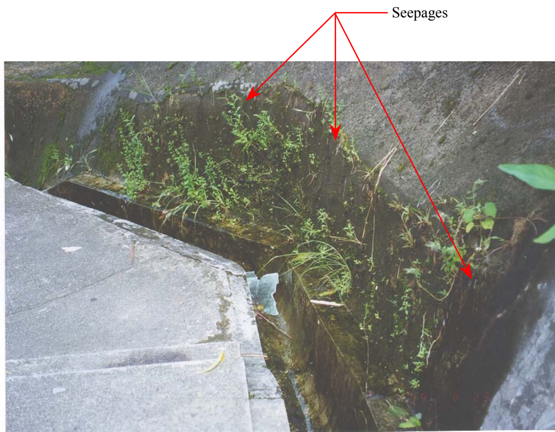
Plate 28 - Seepage at Slope No. 11NW-B/C68 (Photograph Taken on 25 August 1999). See Figure 34 for location.
