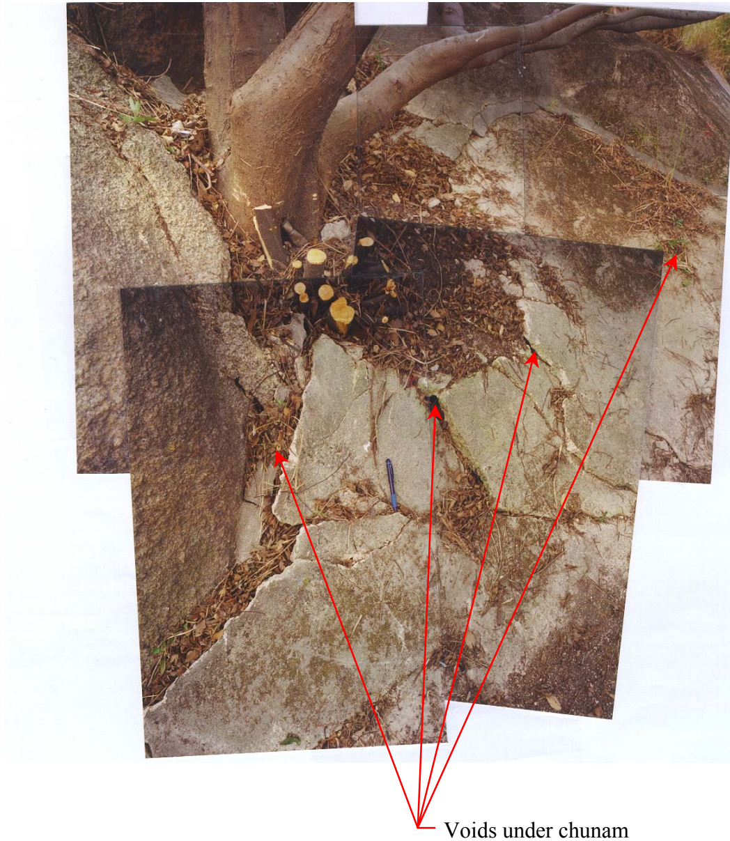
Plate 30 - Disrupted Chunam at Location of Unplanned Vegetation on Slope No. 11NW-B/C90 (Photograph Taken on 11 November 1999). See Figure 34 for location.
