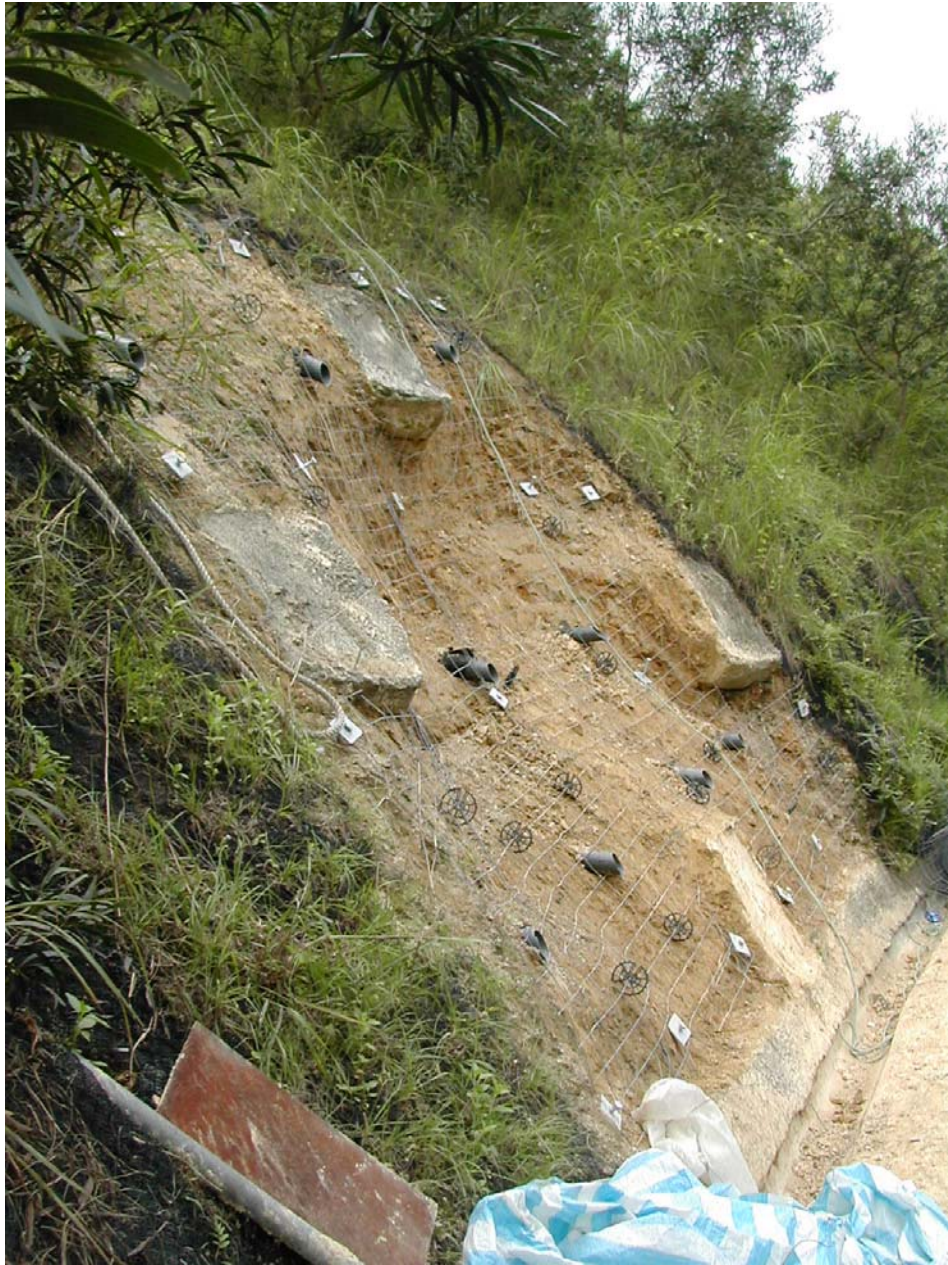
Plate 3 - Local Failure between Soil Nail Heads (Slope No. 6NE-B/C8) (Extracted from Landslide Study Report LSR 1/2004, GEO (2004))
