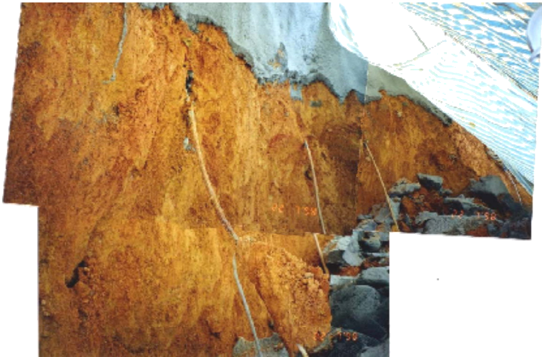
Plate 2 - Failure of Temporary Nailed Cut Slope by Sliding off Front of Soil Nails (Slope No. 8SW-A/C8)
