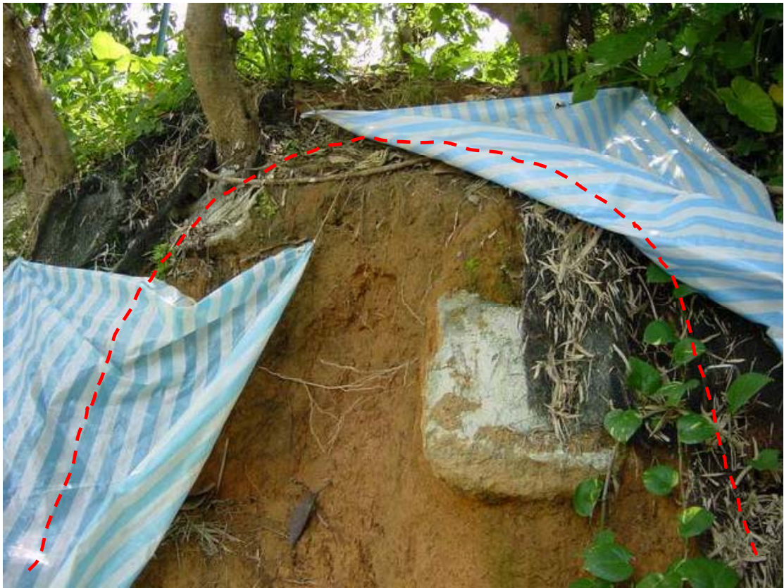
Plate 4 - Local Failure between Soil Nail Heads (Slope No. 6SE-D/C52)
