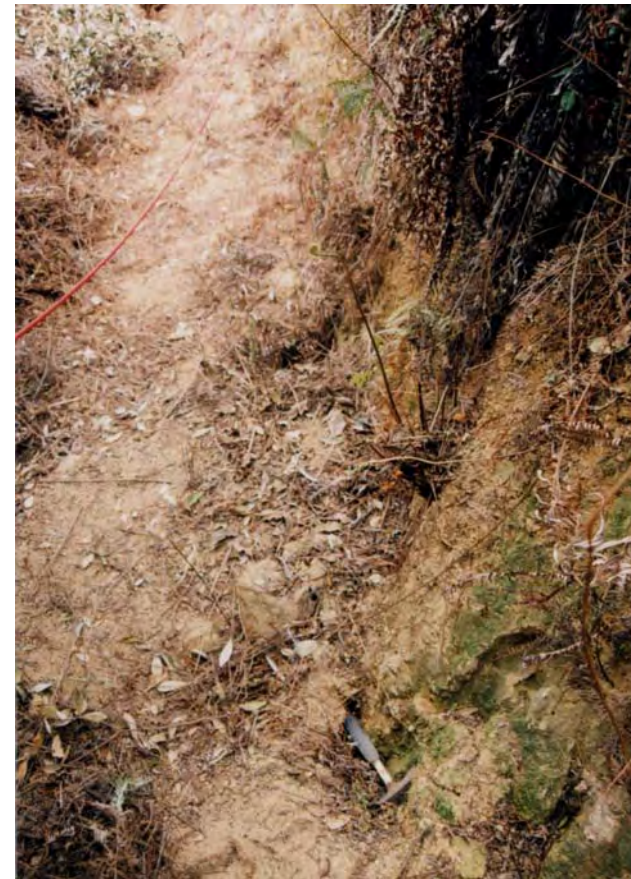
Plate 18 - Tension Crack Along the Base of the Main Scarp below Surface Strip SS1 (Photograph taken on 5 December 2001)
