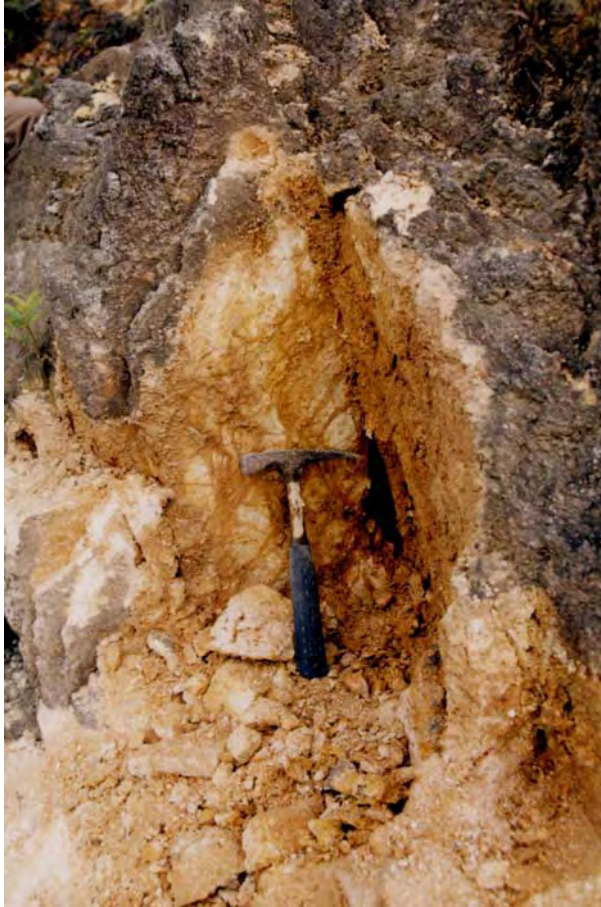
Plate 13 - View of Deformed Rock Mass Within Spur No. 1. Showing Dilation and Voids (Photograph taken on 18 March 2003)
