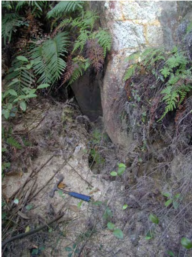
Plate 17 - Tension Crack Along the Base of the Main Scarp below Tor No. 3 (Photograph taken on 5 December 2001)
