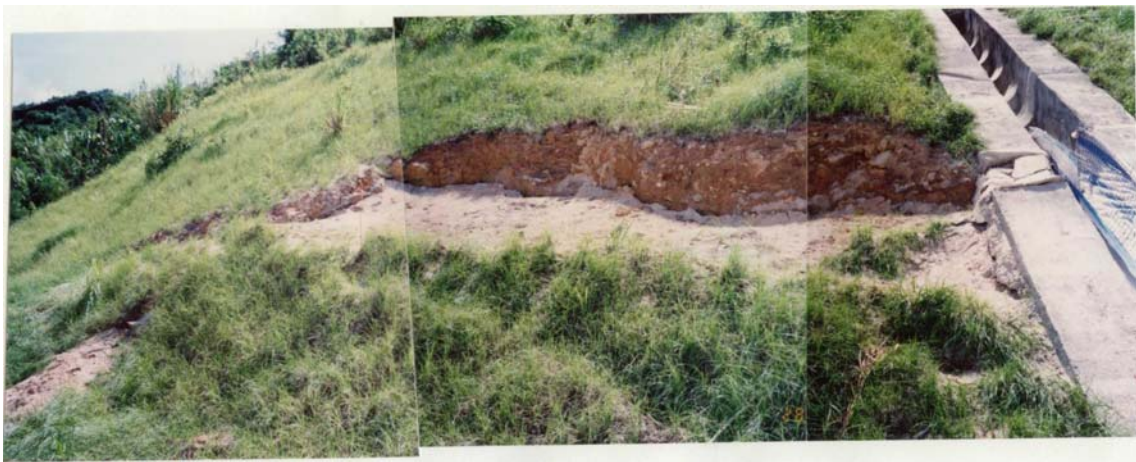
Note: View of a sealed-up tension crack
