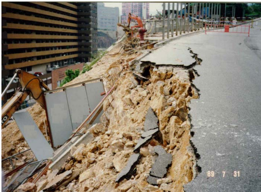
Note: One lane of Kwai Shing Circuit was closed as a result of the landslide
