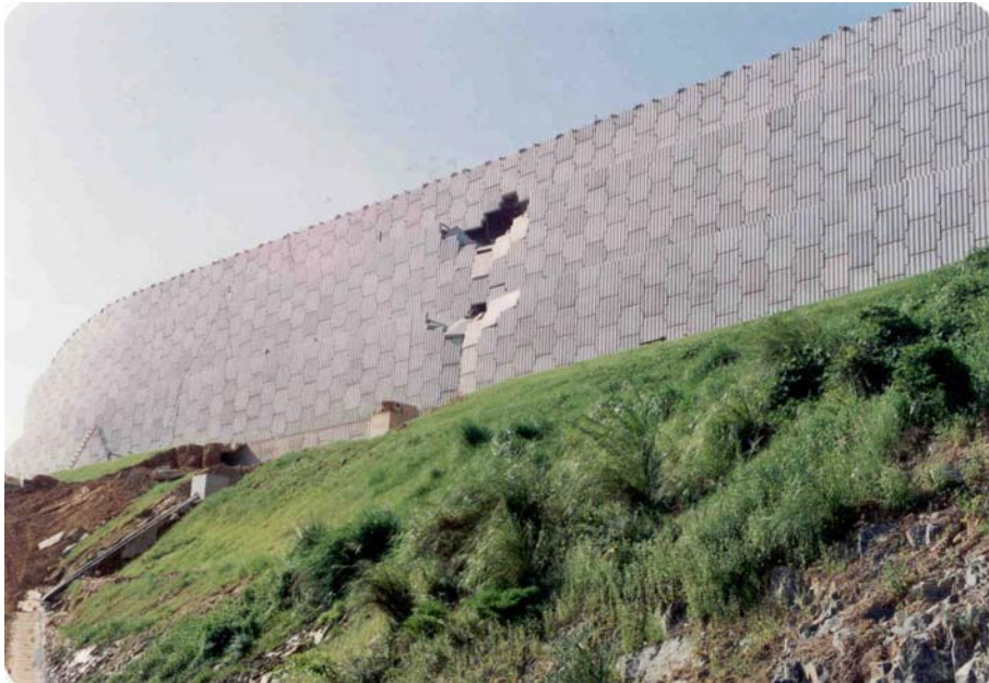
Note: Front view of the damaged facing panels of the reinforced fill wall
