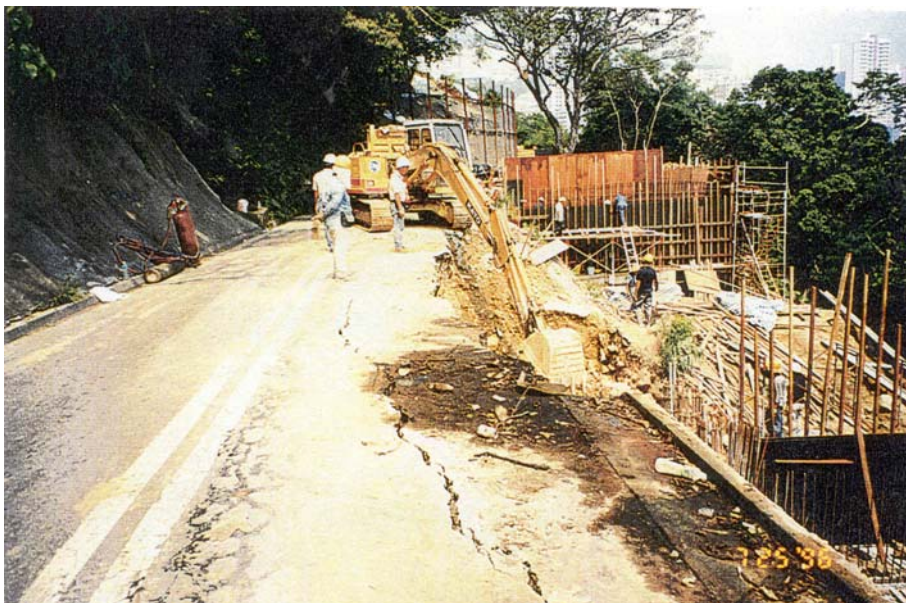
Note: Debris was trapped behind the partially completed concrete retaining wall
