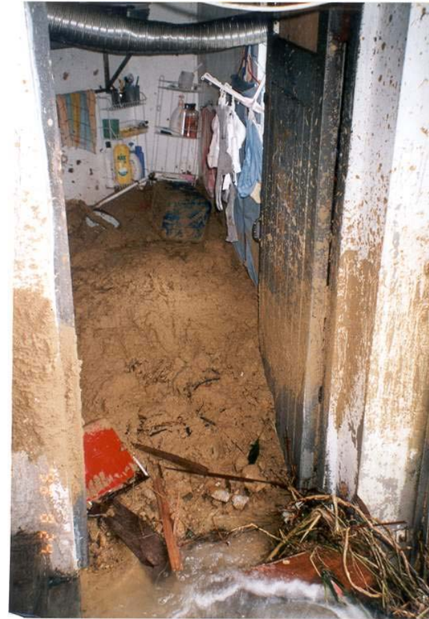
Plate 16 - Slurry-like Debris Inside the House No. 36TS Complex (Photographs Taken on 24 August 1999)
