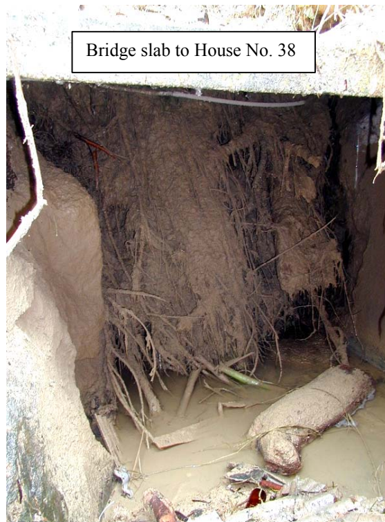
(a) Nullah beneath footbridge to House No.38 totally blocked by fresh vegetation and boulders (Photograph taken on 24 August 1999)
