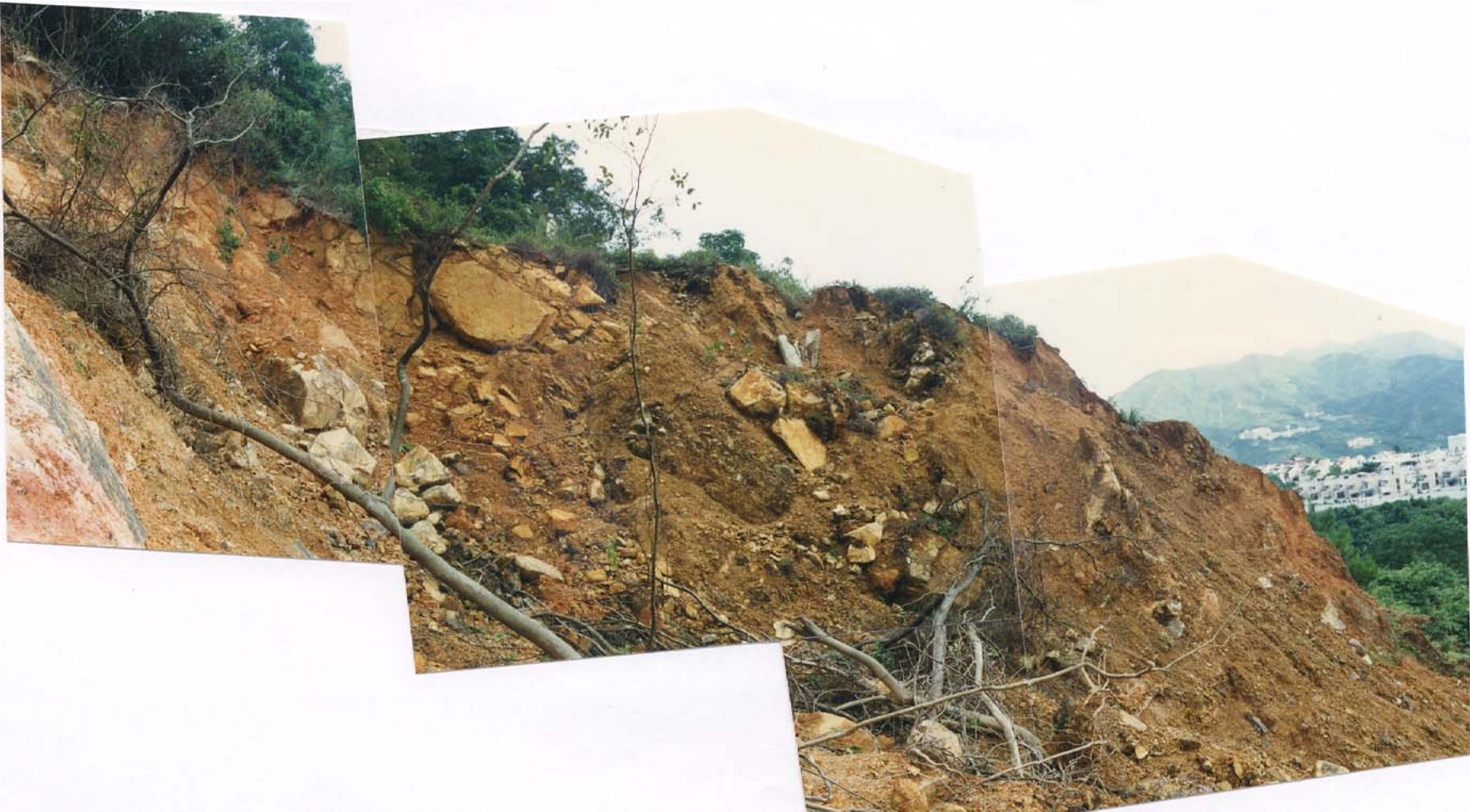
Plate 22 - Left Hand Flank of Landslide Scar 4 Showing Disrupted Rock Mass (Plate Location Shown on Drawing EG503) (Taken on 6/8/97)
