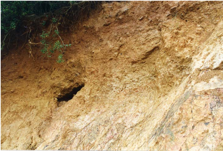
Plate 28(a) - A Large 1.5 m Wide Soil Pipe at the Old Colluvium-New Colluvium Interface Exposed in the Main Scarp of Landslide Scar 5 - Note Slight Seepage (Plate Location Shown on Drawing EG503) (Taken on 7/7/97) GS 97/53/07
