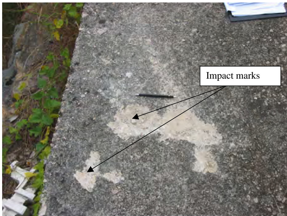
Plate 15 - View of the Impact Marks on Lowermost Berm of Slope No. 11SW-D/C639 (Photograph taken on 5 December 2002)
