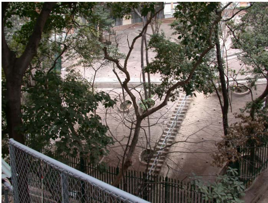
In 2002, the Minipiled Portion of Slope Covered with Shotcrete Surfacing after the Upgrading Works Recently Completed
