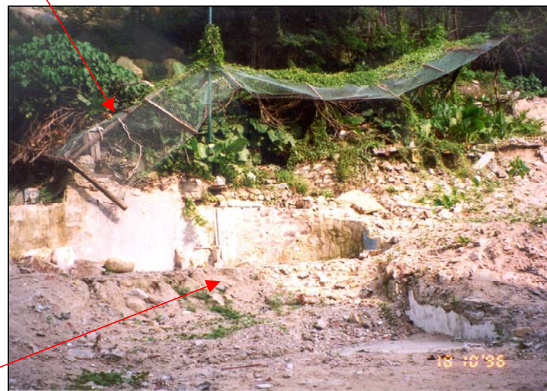
Plate 5 - View Showing the Mitigating Effects of the Rockfall Fence During a Previous Landslide (Photographs taken by GEO on 14 August 1995 and 18 October 1996)
