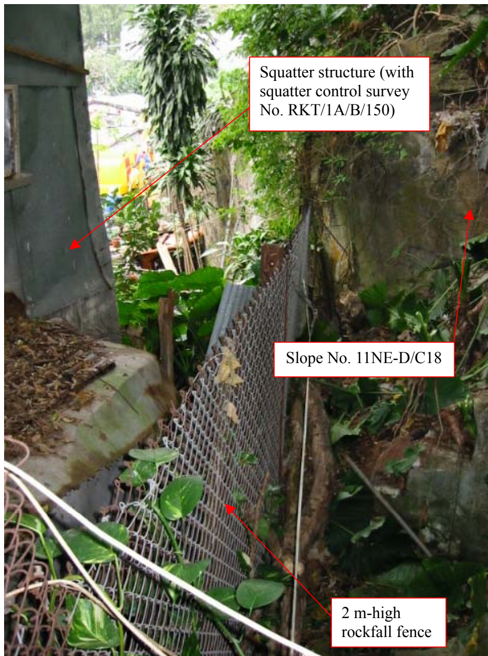
Plate 3 - View of the Rockfall Fence at the Slope Toe (Photograph taken on 27 November 2002)
