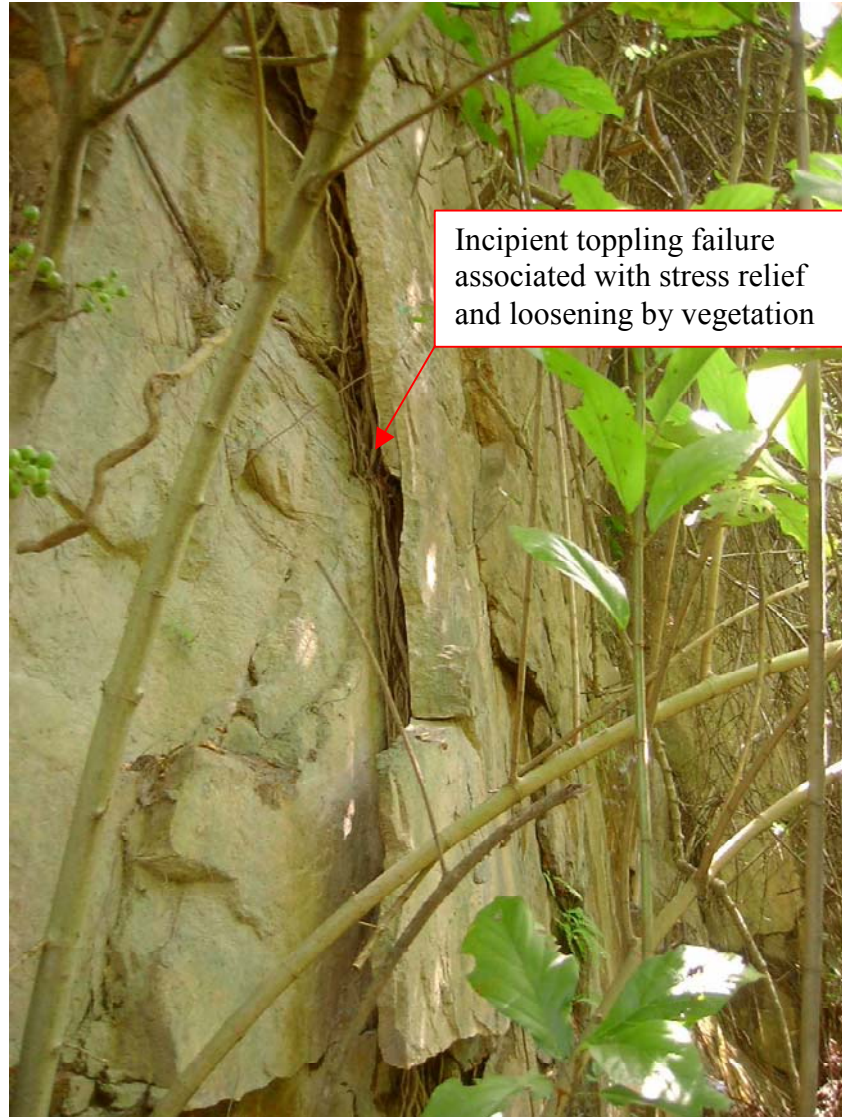
Plate 13 - View of Incipient Failure Exacerbated by Vegetation Growth (Photograph taken on 10 October 2002)
