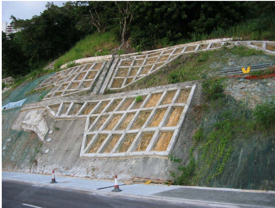
Plate 19 - Reinforced Concrete Beam Grillage Connecting Soil Nail Heads (Photograph taken on 16 August 2002)
