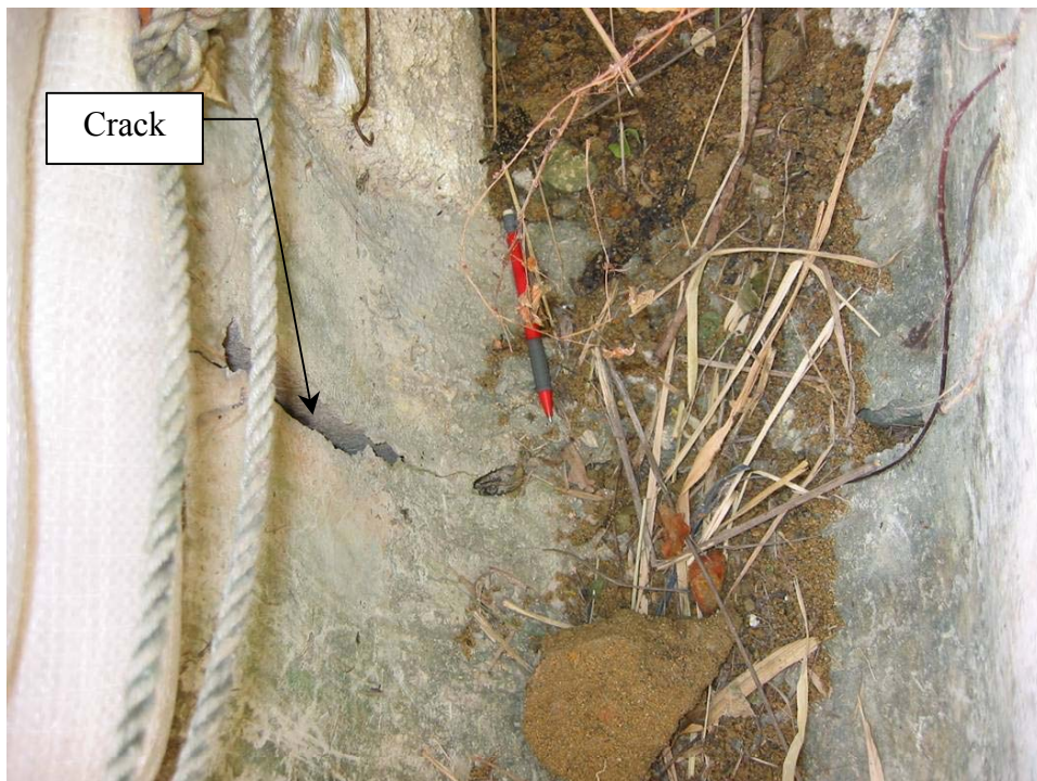
Plate 10 - Cracks up to 30 mm Wide along Construction Joints (Photograph taken on 16 August 2002)
