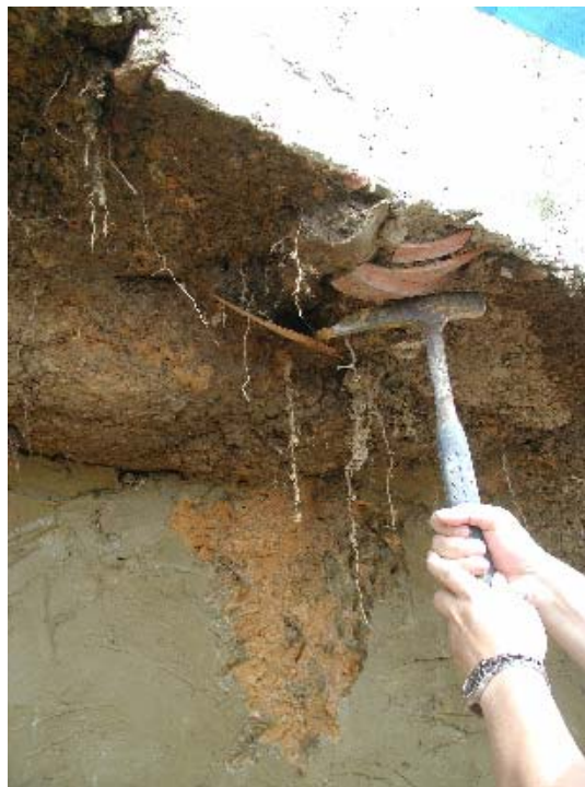
Plate 8 - Broken Ceramic Pipes and Pieces of Plastic beneath the Concrete Berm (Photograph taken on 19 August 2002)
