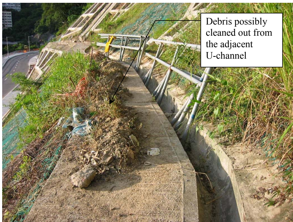
Plate 12 - Debris on the Concrete Berm (Photograph taken on 16 August 2002)
