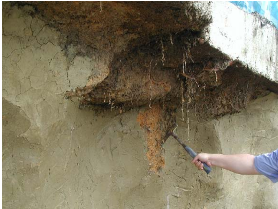
Plate 9 - Slight Seepage from Soil Surface in the Scarp (Photograph taken on 19 August 2002)
