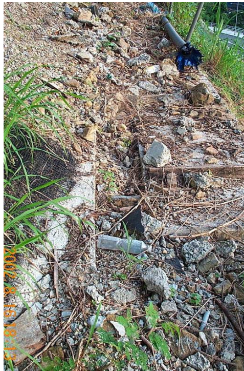
Plate 13 - Construction Waste Blocking a U-channel along the Second Berm (Photograph taken on 16 August 2002)
