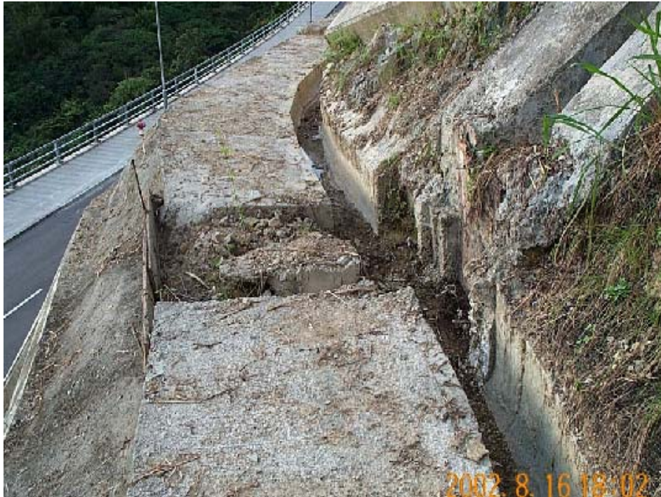
Plate 15 - Catchpit Yet to be Constructed on the First Berm (Photograph taken on 16 August 2002)
