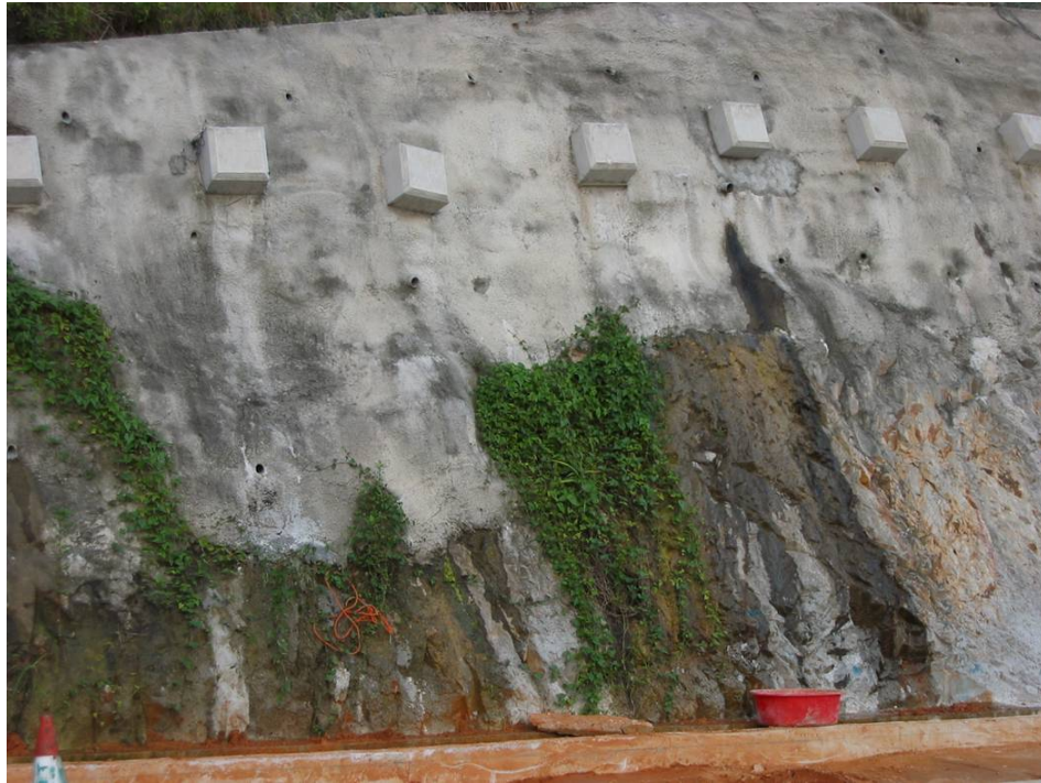
Plate 17 - Extensive Seepage below Shotcrete and above Exposed Rock (Photograph taken on 16 August 2002)
