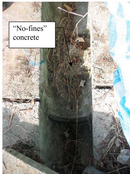
Plate 11 - "No-fines" Concrete in Stepped Channel (Photograph taken on 16 August 2002)
