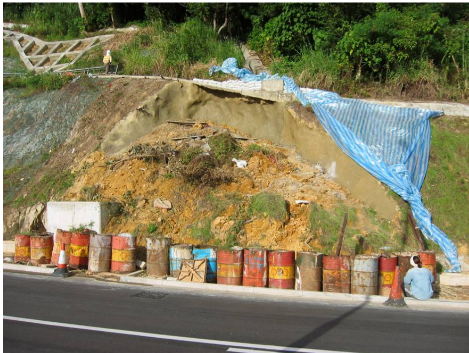
Plate 2 - View of the Failed Portion of the Subject Slope (Photograph taken on 16 August 2002)
