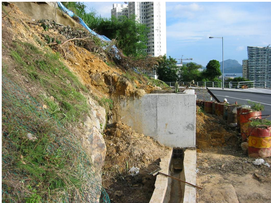
Plate 6 - Concrete Inlet Pit at the Northern End of the Landslide (Photograph taken on 16 August 2002)
