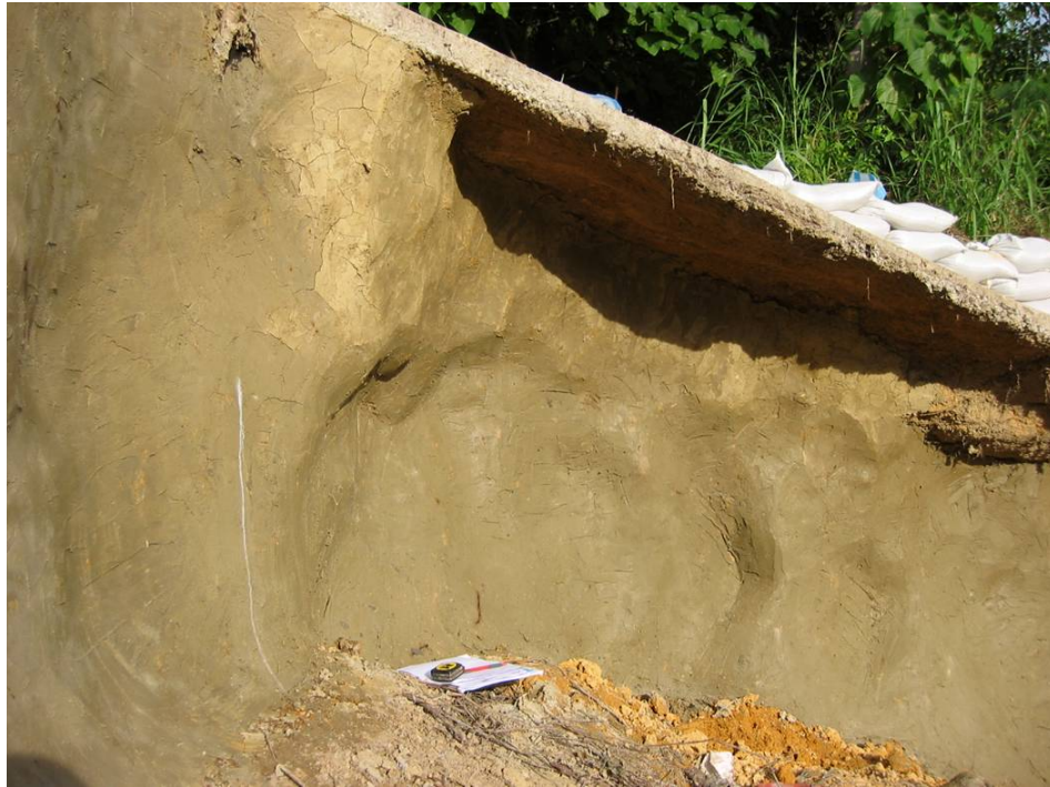
Plate 7 - Back Scarp (Covered with Cement Mortar) and Undercut Concrete Berm (Photograph taken on 16 August 2002)
