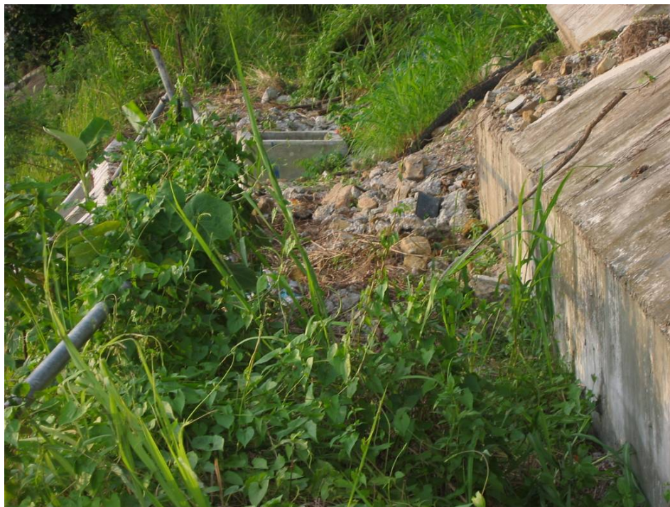
Plate 14 - View of the Blocked U-channel along the Second Berm (Photograph taken on 16 August 2002)
