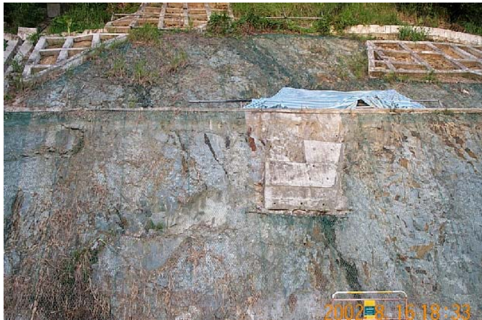
Plate 18 - Wire Mesh Netting Cover to Rock Section (Photograph taken on 16 August 2002)
