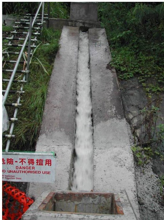
Plate 22 - Heavy Flow of Water in the Stepped Channel to the South of the 2002 Landslide during a Rainstorm (Photograph taken on 17 September 2002)
