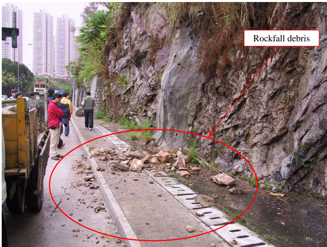
Plate 2 - View of Slope No. 11NW-A/C61 Looking West Showing Rockfall Debris (Photograph taken by GEO on 23 March 2002)
