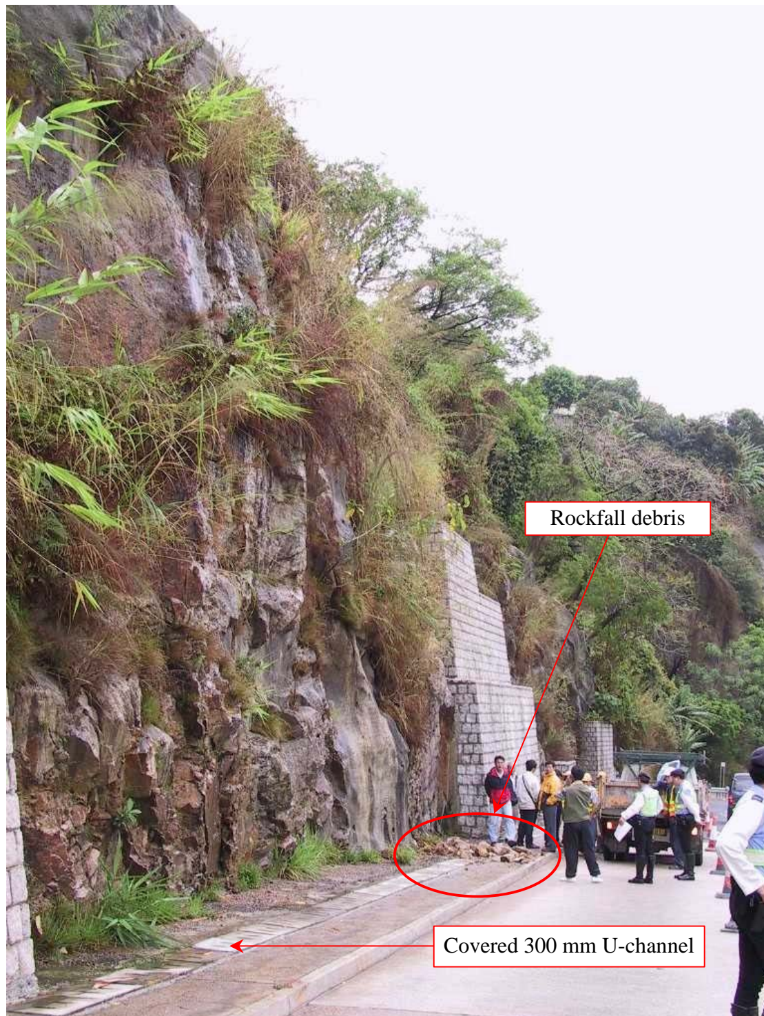
Plate 1 - View of Slope No. 11NW-A/C61 Looking East Showing Debris on the Footpath (Photograph taken by GEO on 23 March 2002)
