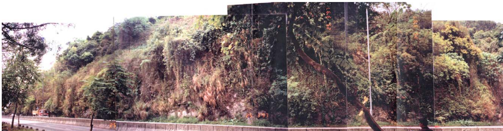
Plate 3 - View of Slope No. 11NW-A/C61 Showing Unplanned Vegetation on the Rock Cut Portion in 1997 (Photograph taken by Mott Connell Ltd on 25 March 1997)
