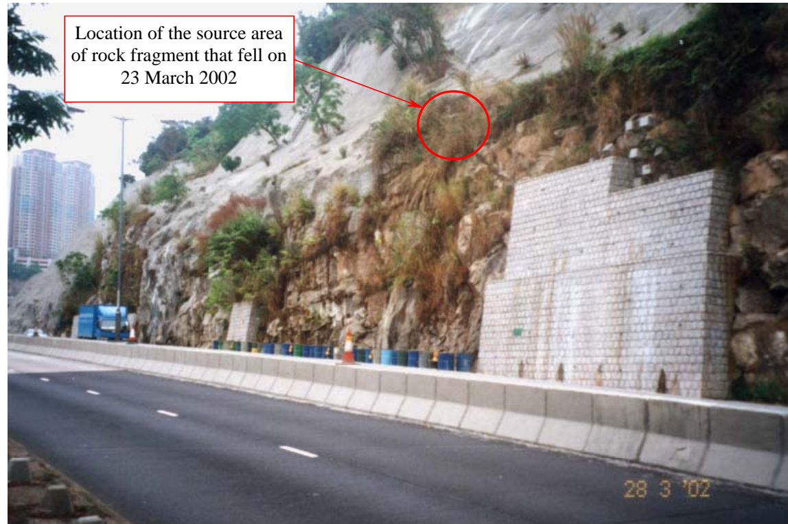
Plate 9 - View of Slope No. 11NW-A/C61 Showing Growth of Unplanned Vegetation on the Rock Portion (Photograph taken on 28 March 2002)
