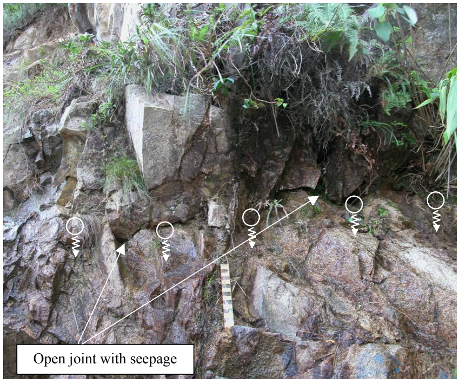
Plate 12 - Detailed View of an Open Joint Daylighting Below a Series of Large Potentially Unstable Blocks (Photograph taken on 14 June 2002 by HCL)
