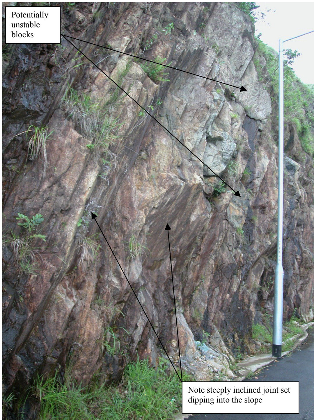
Plate 15 - View of Potentially Unstable Blocks Located at the Central Portion of Slope No. 11NE-A/C284 (Photograph taken on 3 July 2002 by HCL)
