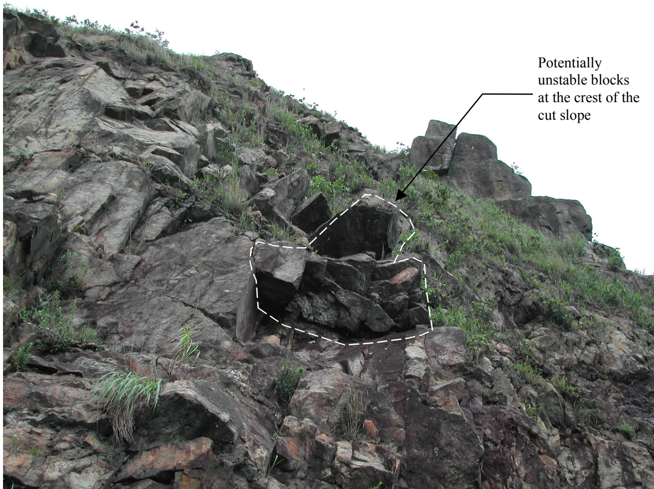
Plate 18 - View of Potentially Unstable Blocks Located at the Crest of Slope No. 11NE-A/C281 (Photograph taken on 23 July 2002 by HCL)
