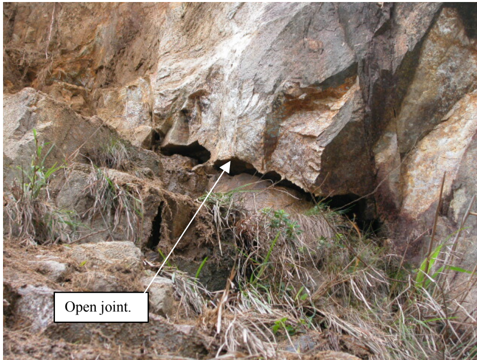
Plate 13 - Detailed View of Open Joint Adjacent to the Source of the Rockfall (Photograph taken on 24 May 2002 by HCL)
