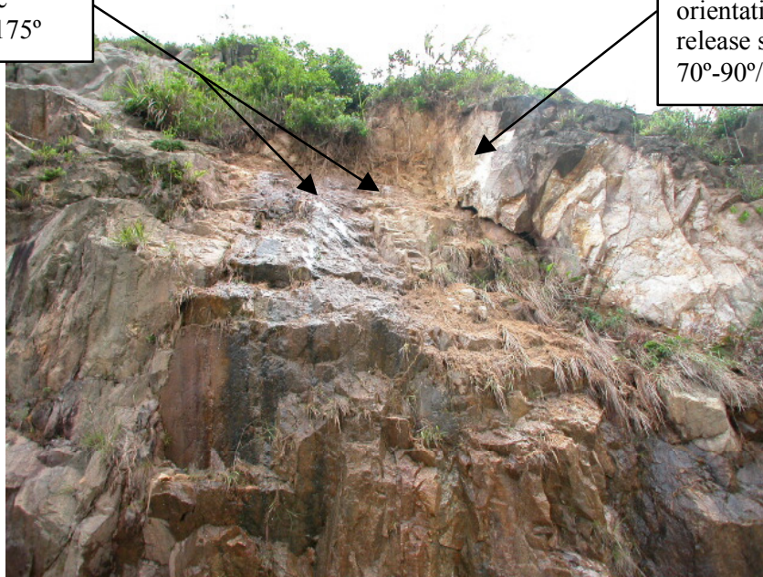
Plate 11 - View of the Source of the Rockfall Showing the Orientations of Principal Release Surfaces (Photograph taken on 24 May 2002 by HCL)
