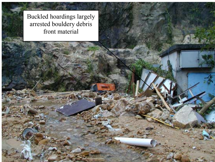
Plate 14 - Buckled Hoardings Adjacent to Pump House Compound (Photograph taken on 5 September 2001)
