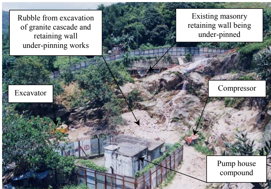
Plate 11 - View of the Active Construction Site (Photograph taken on 1 August 2001)
