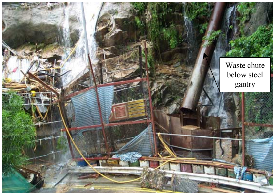
Plate 16 - Deformed Temporary Fence on Lei Pui Street below the Active Construction Site (Photograph taken on 2 September 2001)
