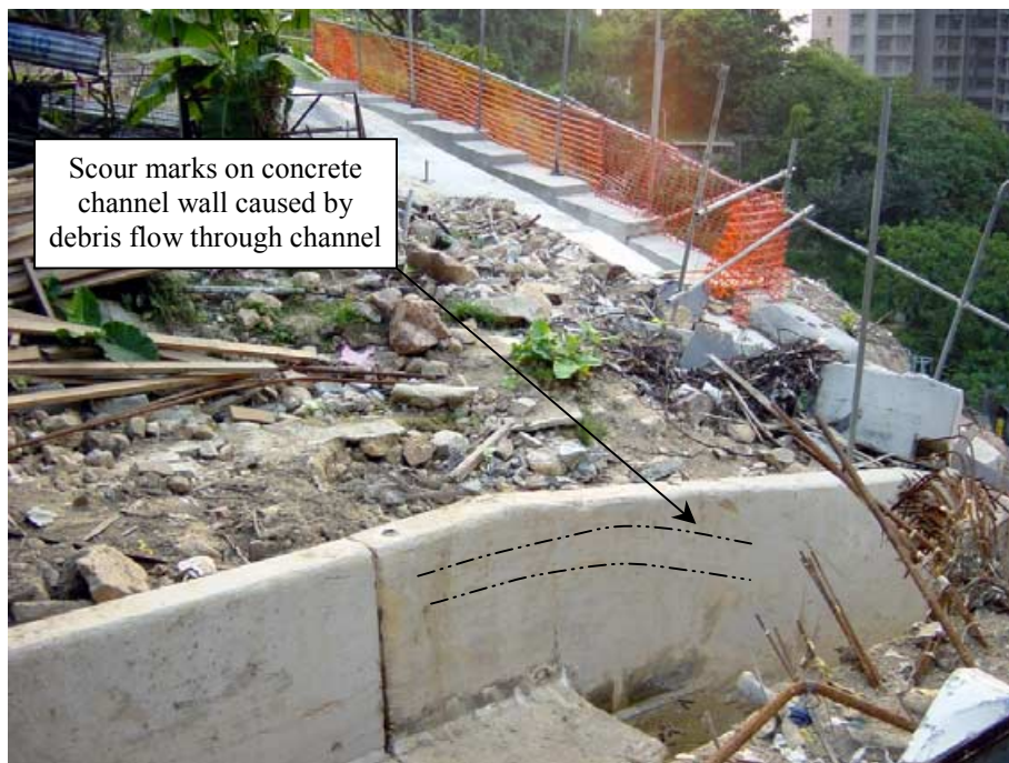
Plate 24 - View of the Concrete Channel above the Active Construction Site Showing Scour Marks on the Wall Face Indicating the Debris Trajectory (Photograph taken on 18 October 2001)
