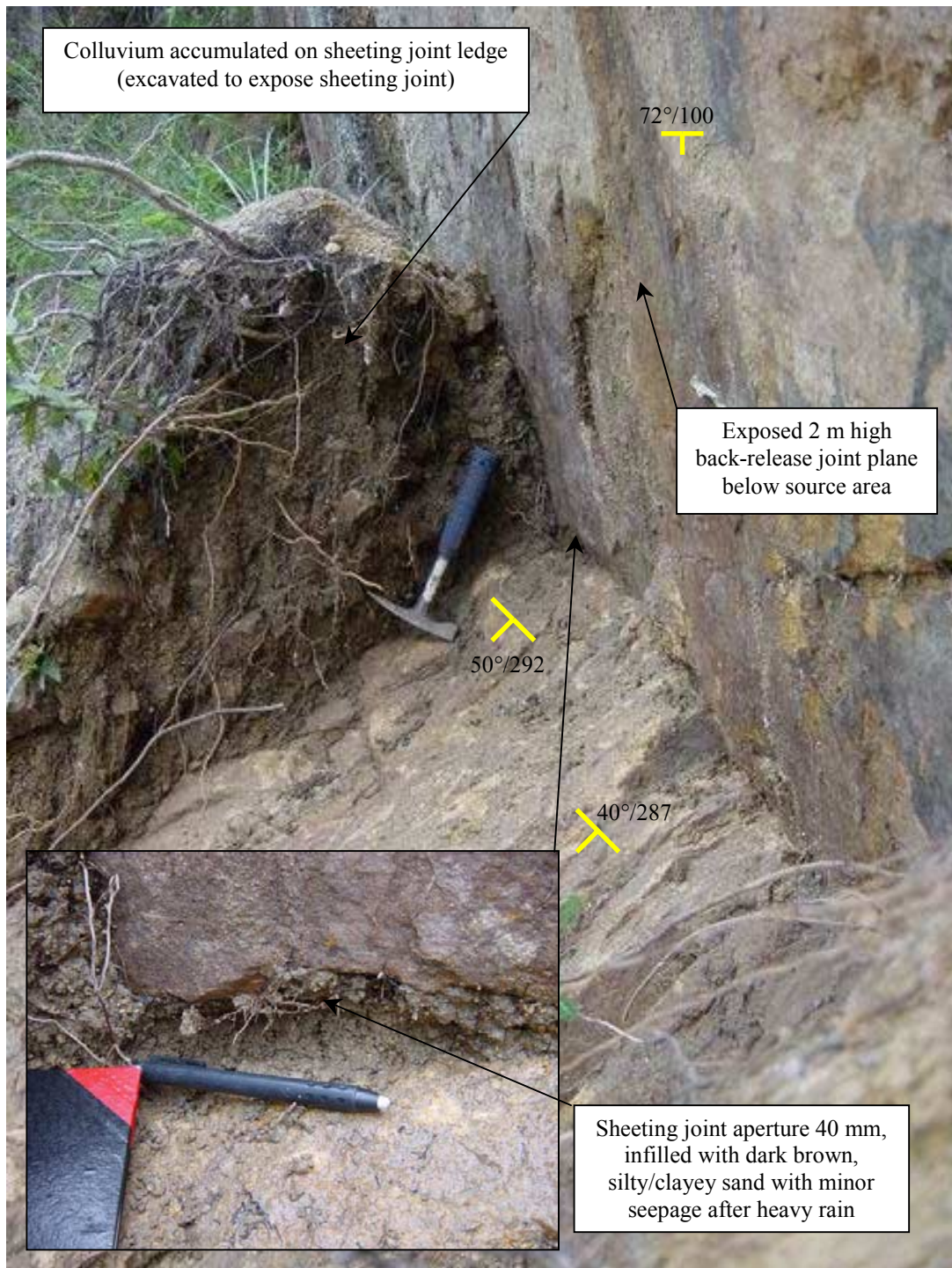
Plate 34 - View of the Sheeting Joint Ledge below the Source Area (Photograph taken on 24 May 2002)
