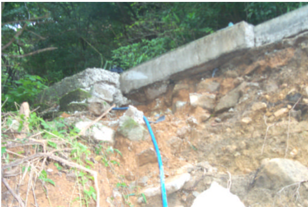
Plate 4 - View of a Section of Collapsed No-fines Concrete Edge Strip and Kerbstone (Photograph taken on 10 September 2001)
