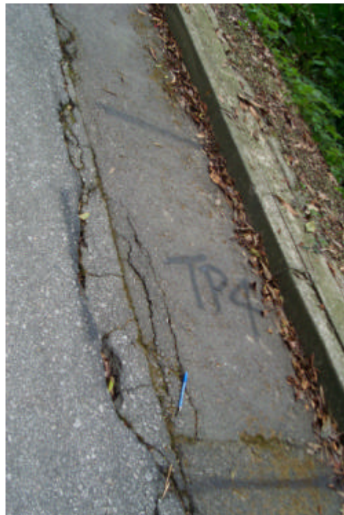
Plate 8 - View of Crack No. 1 Observed above Landslide Scar on Western Side of Kwun Ping Road (Photograph taken on 13 December 2001)
