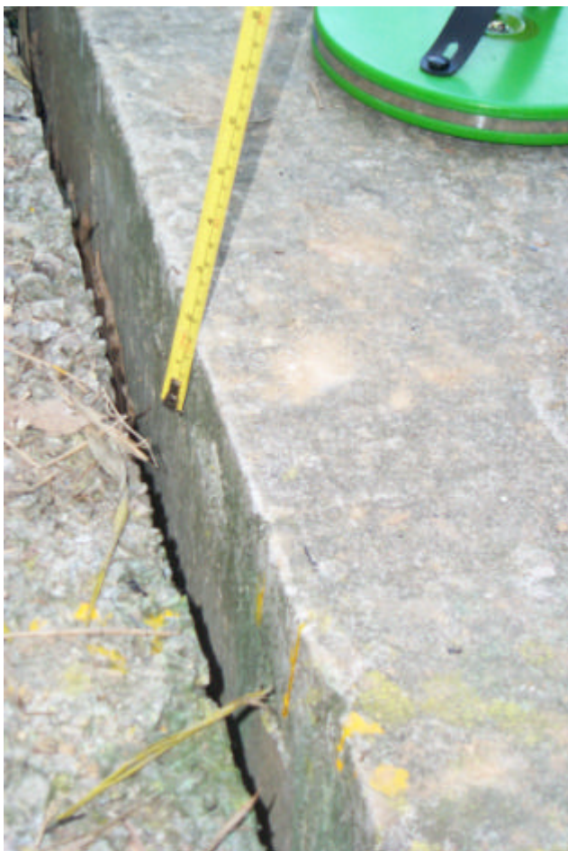
Plate 11 - Differential Settlement about 30 mm across Crack No. 2 (Photograph taken on 4 January 2002)
