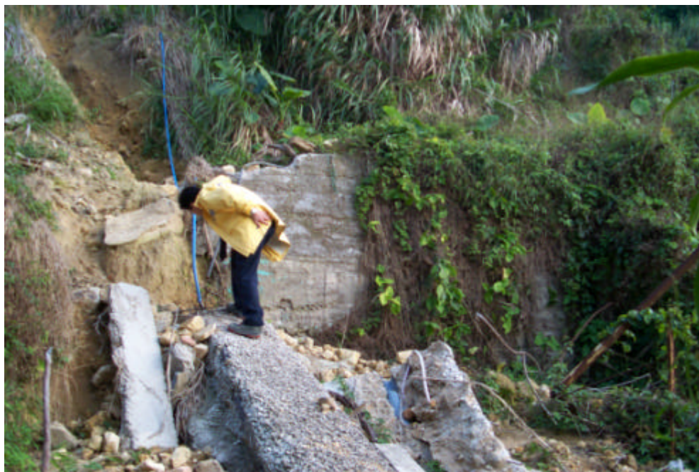
Plate 5 - View Showing Damaged Concrete Retaining Wall behind Area with Remains of Squatter Units (Photograph taken on 21 January 2002)
