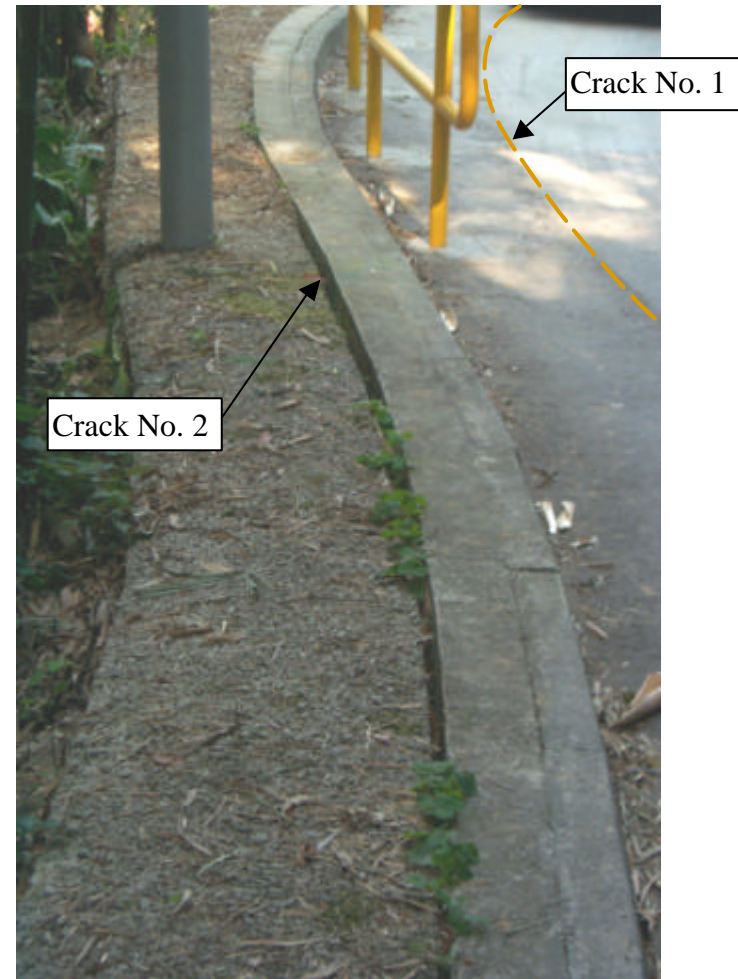
Plate 10 - Differential Settlement along Kerb/No-fines Concrete Edge Strip (Photograph taken on 4 January 2002)
