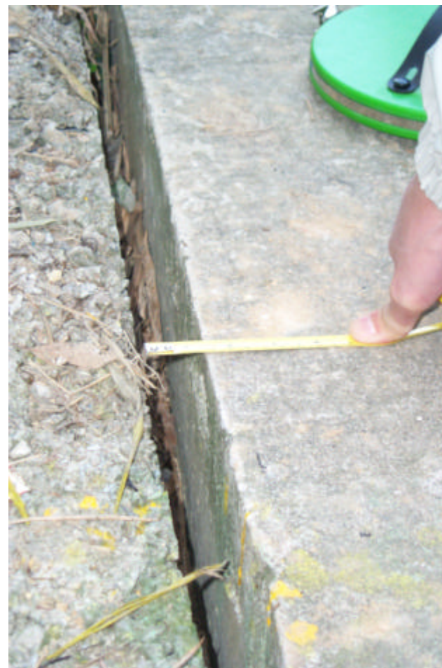
Plate 12 - Width of Gap about 35 mm across Crack No. 2 (Photograph taken on 4 January 2002)
