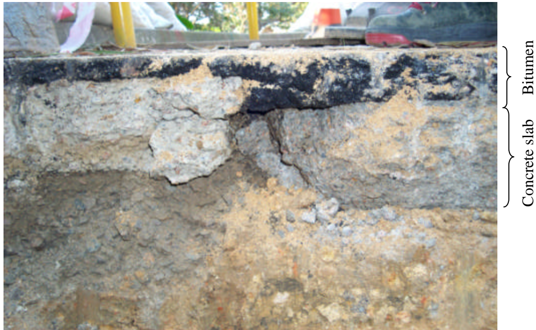
Plate 13 - View Showing a Typical Section through the Road Pavement in Trial Pit No. TP3 (Photograph taken on 21 January 2002)
