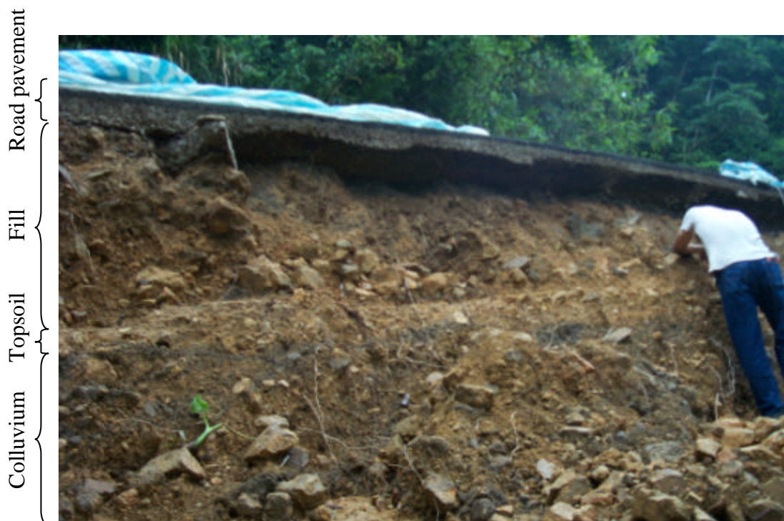
Plate 2 - Collapse of Sub-grade below Kwun Ping Road (Photograph taken on 10 September 2001)
