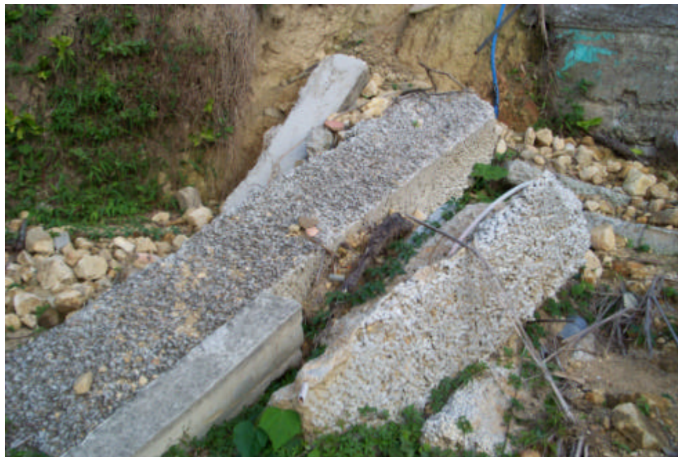
Plate 6 - View Showing Fragments of Displaced No-fines Concrete Edge Strips (Photograph taken on 21 January 2002)
