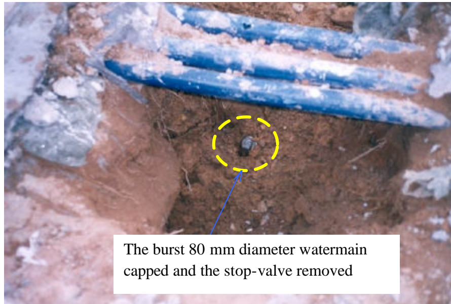
Plate 6 - The Burst Watermain Capped (Photograph taken on 14 December 2001 by WSD)
