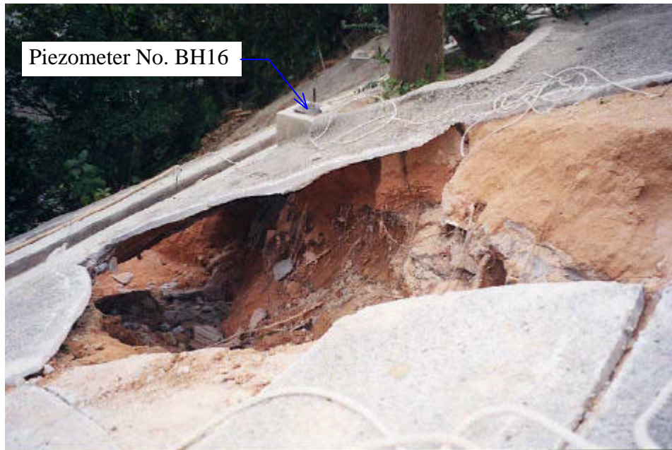
Plate 1 - Washout of Soil from underneath the Shotcrete Cover at the Subject Slope (Photograph taken on 4 February 2002)
