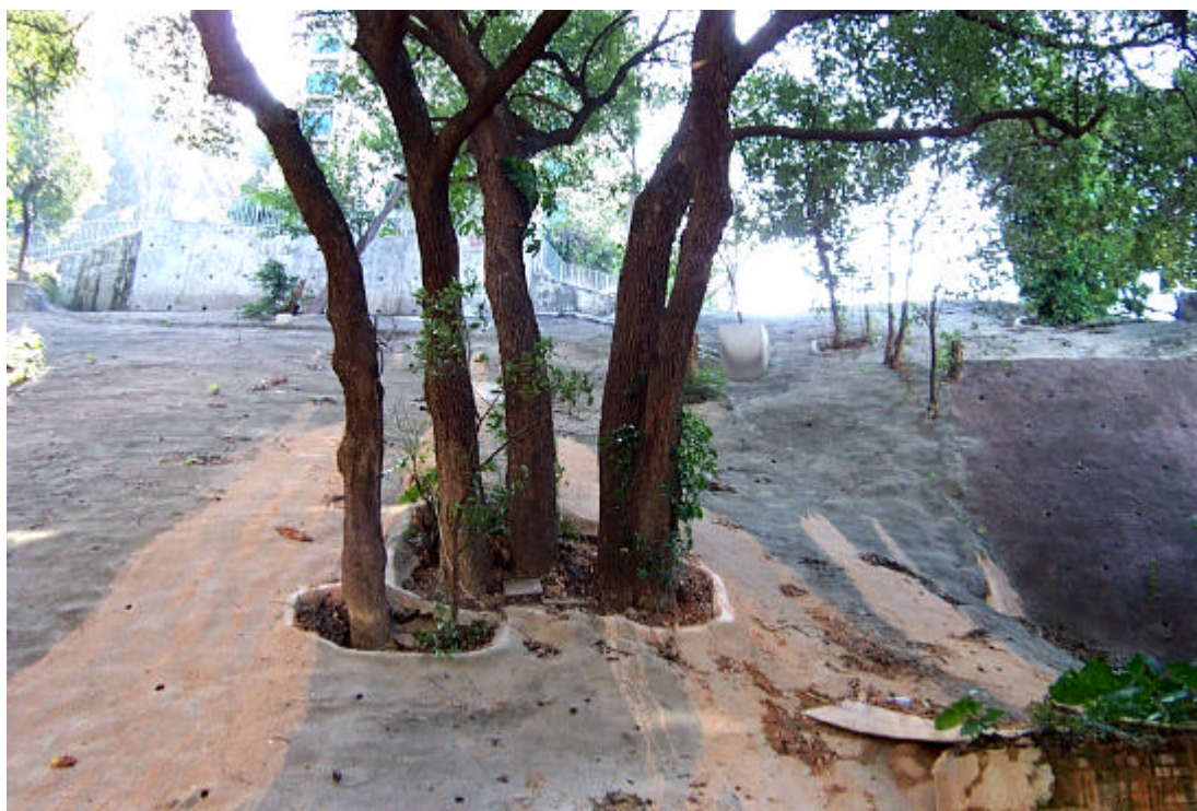
Plate 10 - Washout of Soil at the Subject Slope through Weepholes and Cracks on the Shotcrete Cover (Photograph taken on 15 December 2001)
