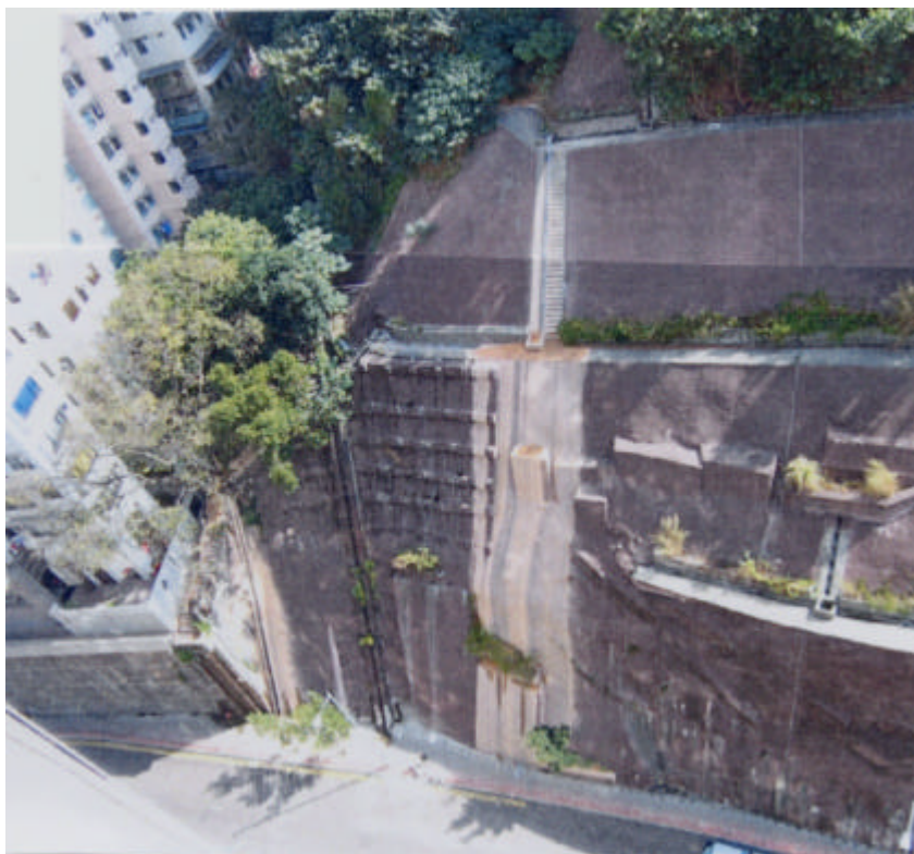
Plate 2 - Outwash Cascaded down the Face of Slope No. 11SW-A/C747 (Photograph taken on 15 December 2001)
