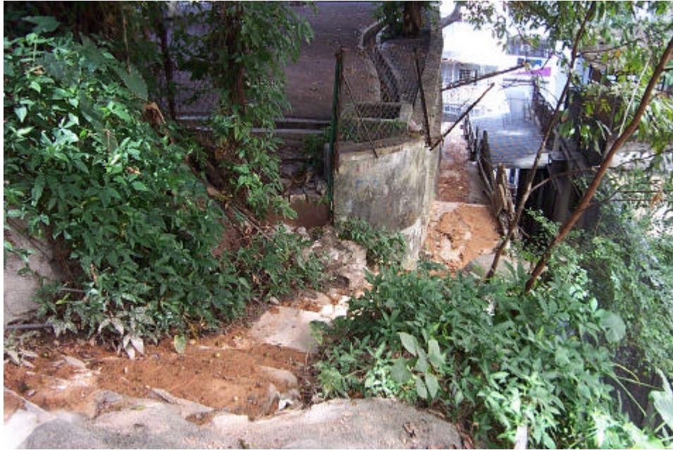
Plate 11 - Washout Debris Deposited along a Footpath Leading to Rock Hill Street (Photograph taken on 15 December 2001)
