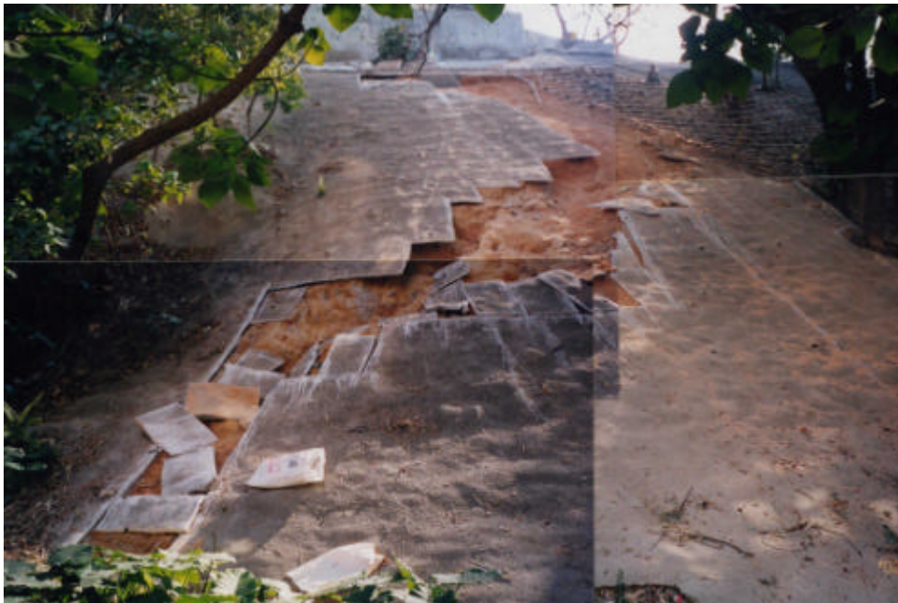
Plate 12 - Erosion Gully at the Subject Slope (Photograph taken on 25 February 2002)
