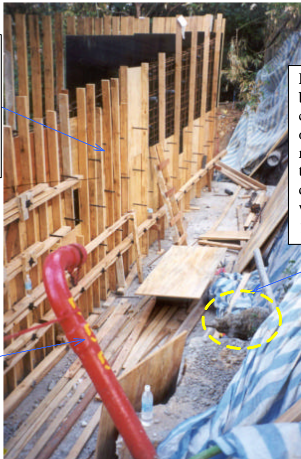
Plate 4 - L-shaped Retaining Wall being Constructed After the August 1999 Landslide Incident (Photograph taken in November 1999 by HyD)
