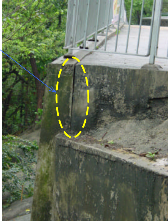
Plate 8 - Gap Observed at the Western End of the Wall (Photograph taken after the 14 December 2001 watermain burst)
