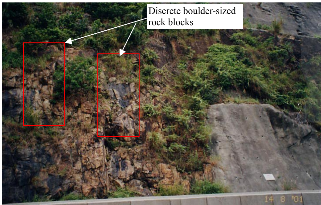
Plate 22 - View of Discrete Boulder-sized Rock Blocks near the Middle of the Exposed Rock Portion of Slope No. 11NW-A/C58 (Photograph taken on 14 August 2001)
