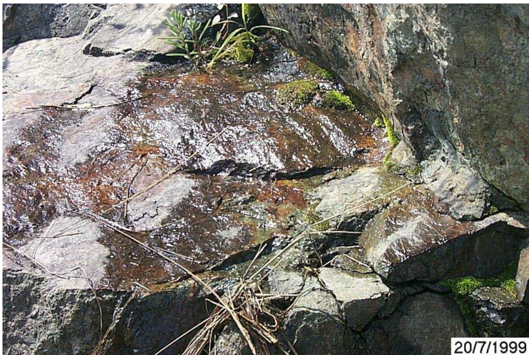
Plate 16 - Slight to Moderate Seepage at Mid-height on Slope No. 11NW-A/C58 (Photograph taken by GEO on 20 July 1999)
