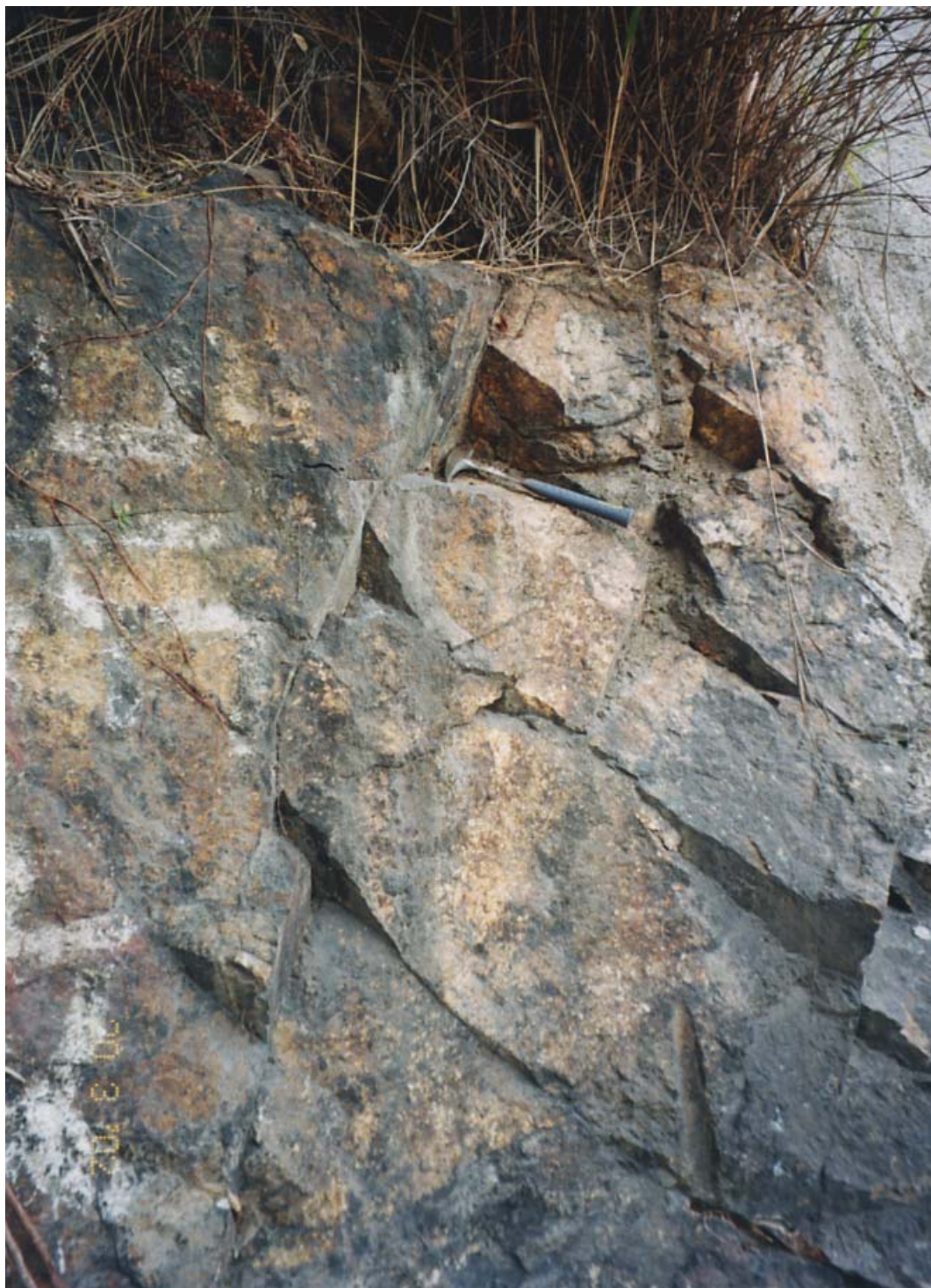
Plate 18 - View of Wedge Failure at the Rock Portion of Slope No. 11NW-A/C 58 (Photograph taken on 20 March 2002)
