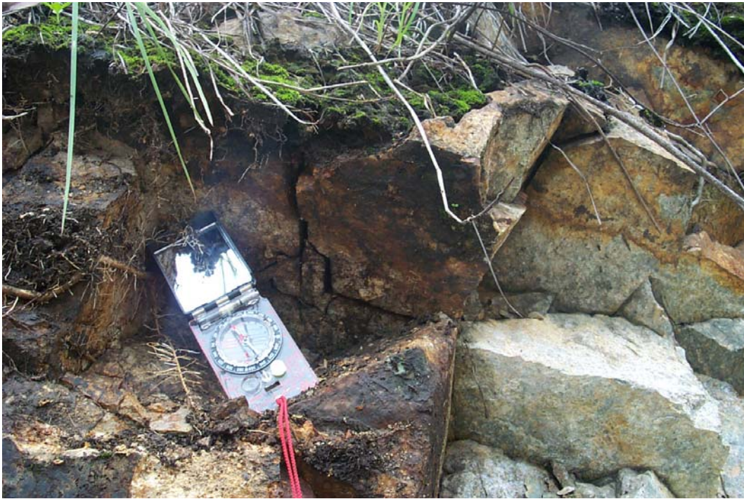
Plate 21 - View of Loose Rock Fragments on the Surface of the Exposed Rock Portion of Slope No. 11NW-A/C58 (Photograph taken on 14 June 2001)
