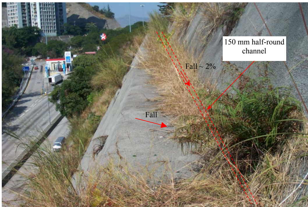
Plate 28 - View Looking Northwest along Second Berm near Location of Discharge onto Exposed Rock Face (Photograph taken on 14 August 2001)
