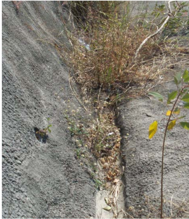
Plate 27 - View Looking Southeast along Second Berm showing Berm Drainage Partly Blocked by Unplanned Vegetation (Photograph taken on 14 August 2001)
