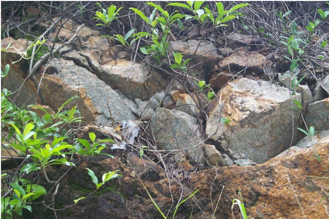
Plate 20 - View of Loose Rock Fragments with Vegetation Growing in the Joints (Photograph taken on 14 June 2001)
