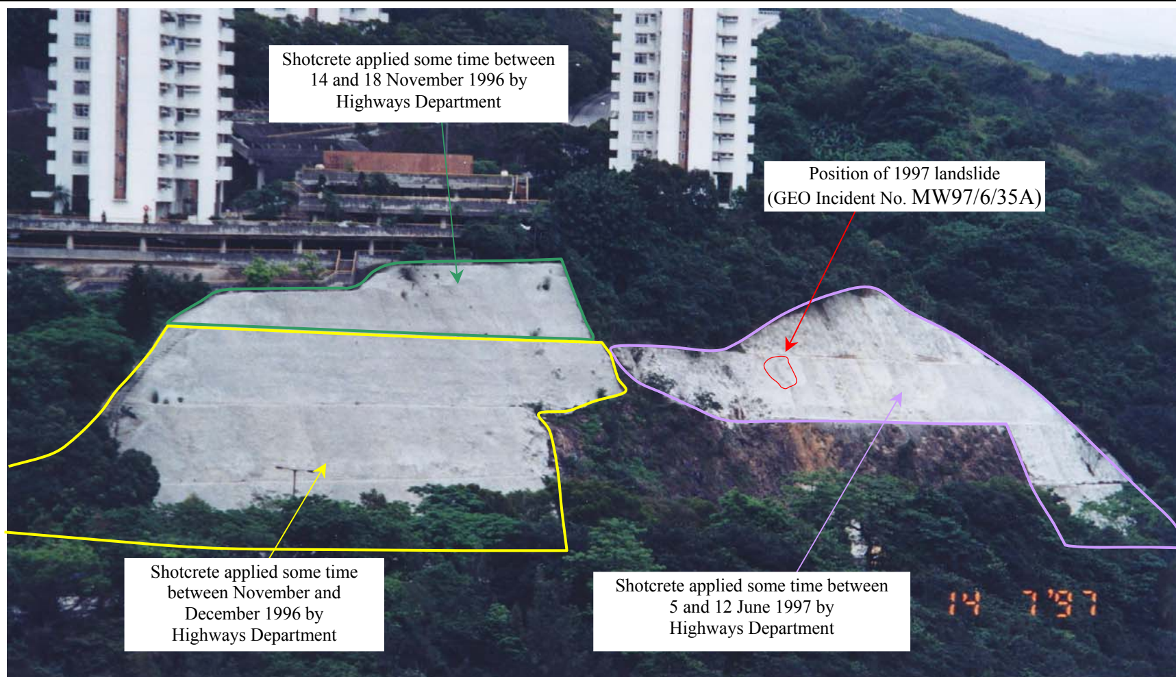
Plate 11 - General View of Slope No. 11NW-A/C58 showing Date and Extent of New Shotcreting Based on API and Site Inspection Record (Photograph taken by HAP on 14 July 1997)
