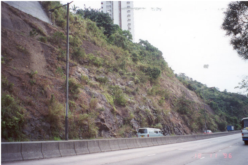
Plate 10 - General View of Slope No. 11NW-A/C 58 in 1996 showing Unplanned Vegetation on Exposed Rock Portion (Photograph taken by GEO on 18 November 1996)
