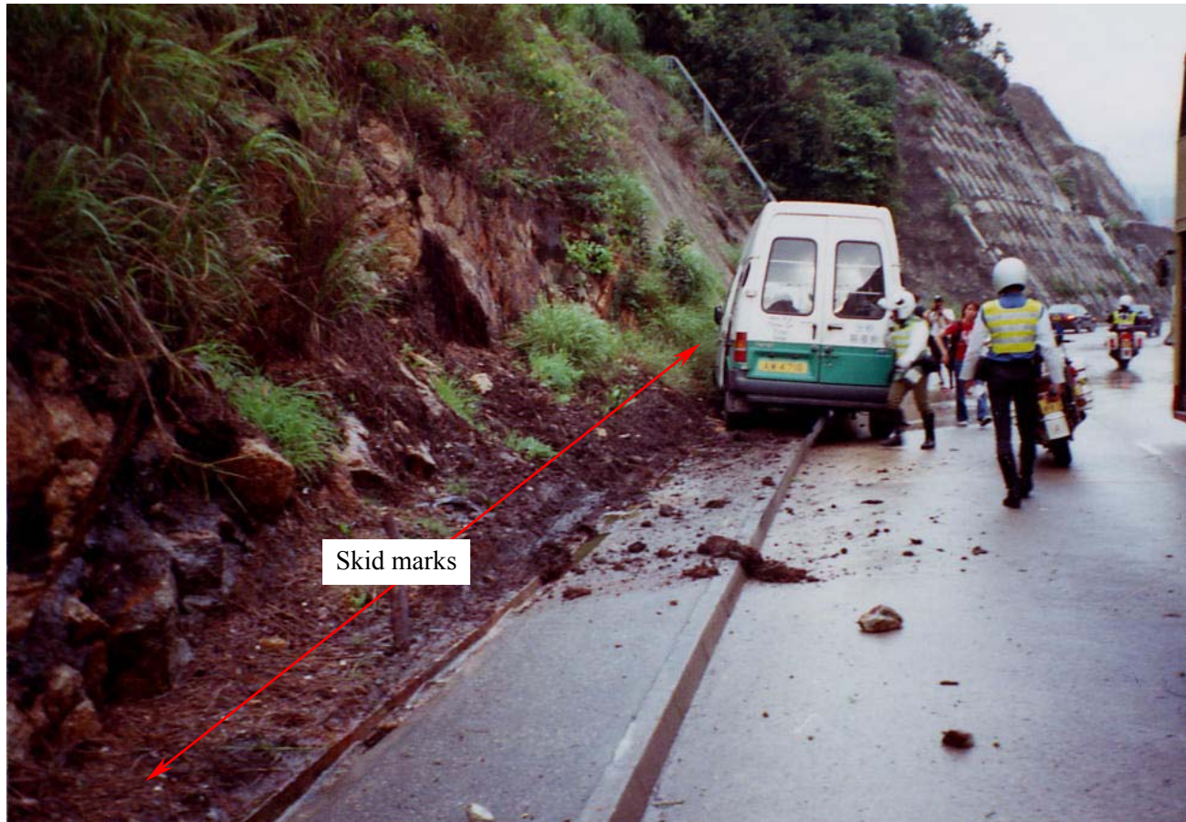
Plate 3 - View from Rear of Post Office Van after Rockfall Incident (GEO Incident No. MW2001/06/007) (Note skid marks at toe of slope shows the van travelled at least 10 m after the incident. Photograph taken by Police on 9 June 2001)
