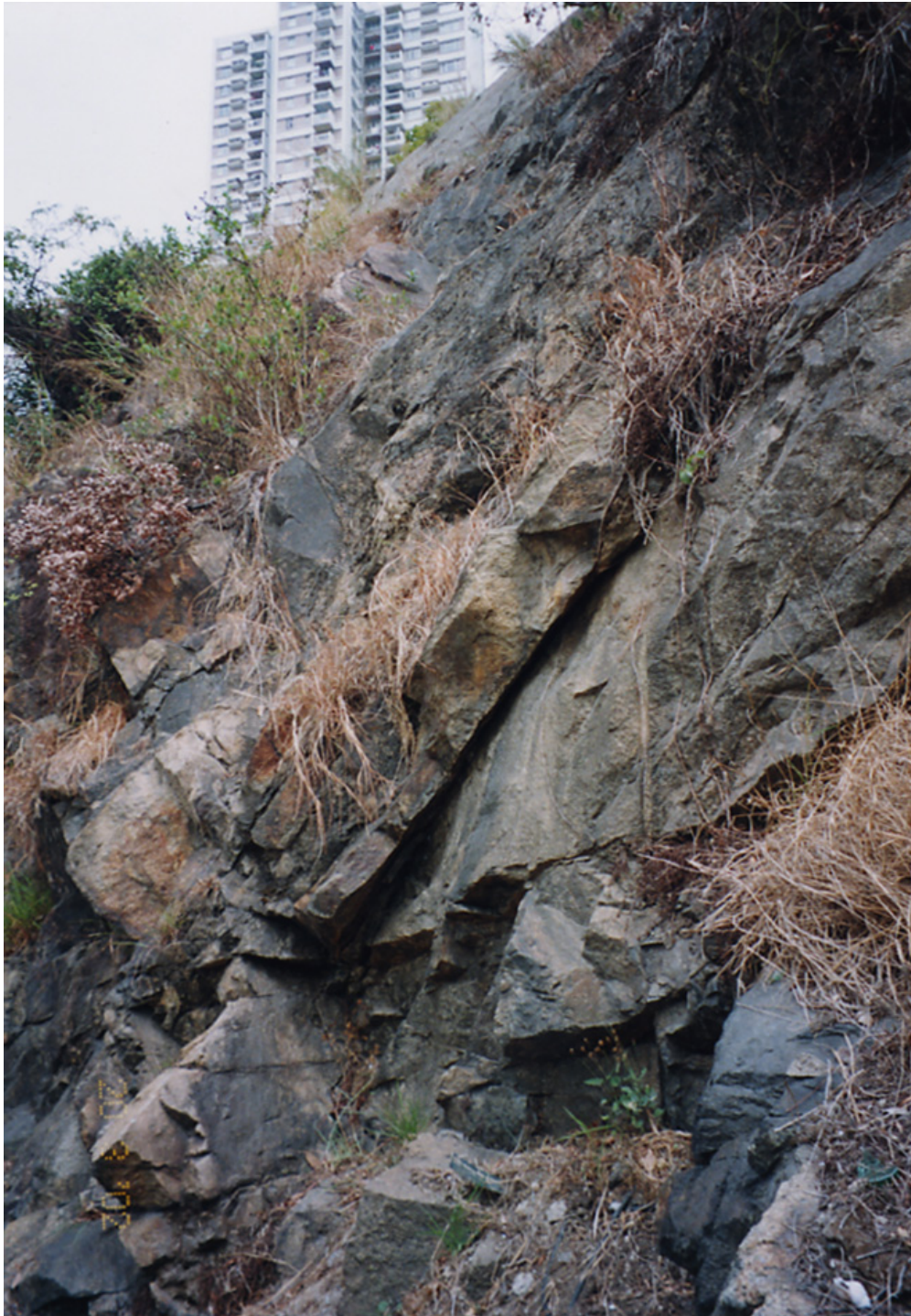
Plate 17 - View of Adverse Sheeting Joint near Centre of Rock Portion of Slope No. 11NW-A/C 58 (Photograph taken on 20 March 2002)
