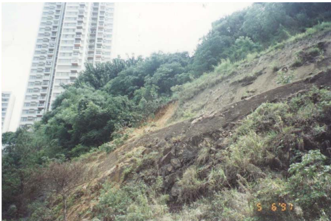
Plate 15 - Failure Scar on Slope No. 11NW-A/C58 of the GEO Incident No. MW97/6/35A (Photograph taken by GEO on 5 June 1997)
