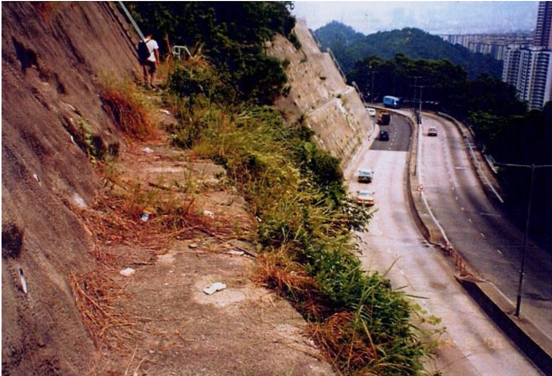
Plate 6 - View of Second Berm on Slope No. 11NW-A/C58 (Note there is no drainage provision on the berm near the southeastern end. Photograph taken on 14 August 2001)
