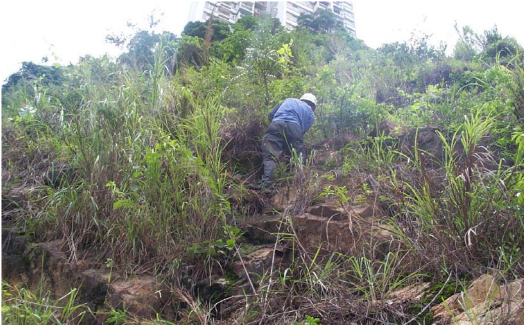
Plate 23 - Heavy Growth of Vegetation on the Exposed Rock Portion of Slope No. 11NW-A/C58 (Photograph taken on 21 June 2001)
