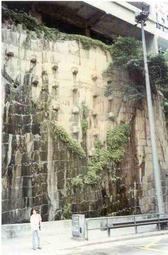
Plate 10 - View East across King's Road towards Slope No. 11SE-A/C14 Following Installation of Rock Bolts in Large Wedge Exposed in Slope Face. Note Seepage from Joint Sets Forming Wedge. Vegetation on Slope Face in 1983 Photograph (Plate 9) Removed. (Photograph Taken by the GEO in January 1984)
