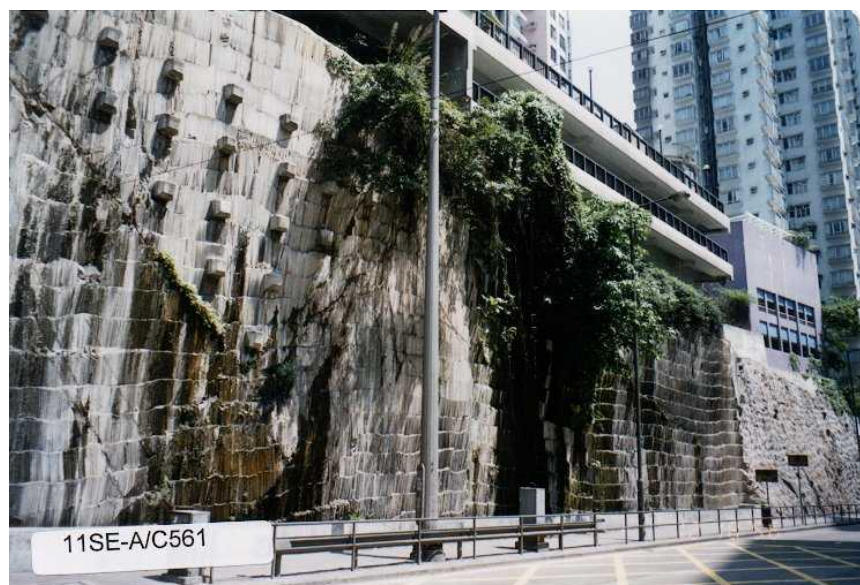
Plate 2 - View Southeast across King's Road towards Slope No. 11SE-A/C561 Showing Vegetation Growing on Slope Face and Seepage Issuing from Joints Defining Large Wedge (Photograph Taken in April 1996)
