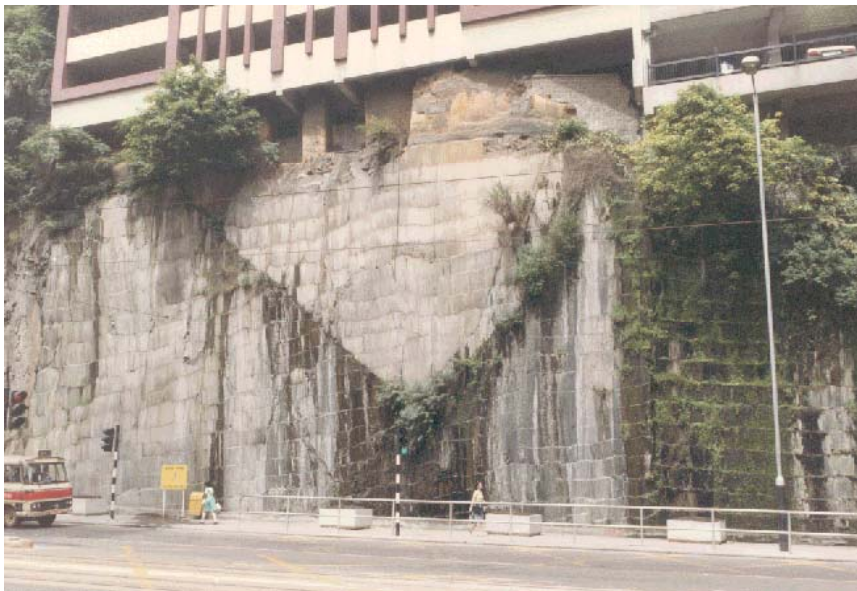
Plate 9 - View East across King's Road towards Slope No. 11SE-A/C14 Prior to Installation of Rock Bolts in Large Wedge Exposed in Slope Face. Note Seepage from Joint Sets Forming Wedge and Vegetation Growing on Slope Face, Notably at Location of June 2001 Rockfall. (Photograph Taken in 1983)
