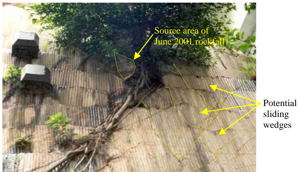
Plate 5 - Close View of Slope Face Showing Source Location of Rock Fall Immediately above Tree (Unplanned Vegetation) Growing on Slope Face. Intersection of Predominant Joint Orientations Results in Potential Sliding Wedges (Photograph Taken on 26 June 2001)
