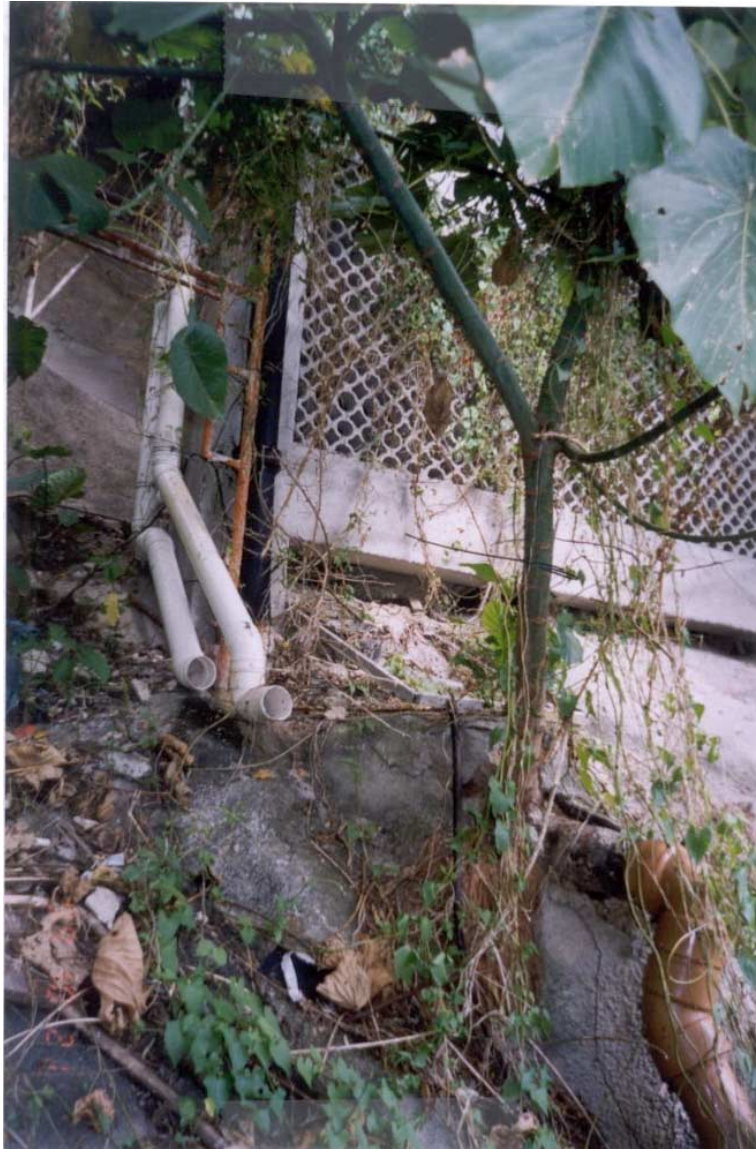
Plate 9 - Discharge Pipes below Podium of Golden Time Villas (Photograph Taken on 21 October 1999)
