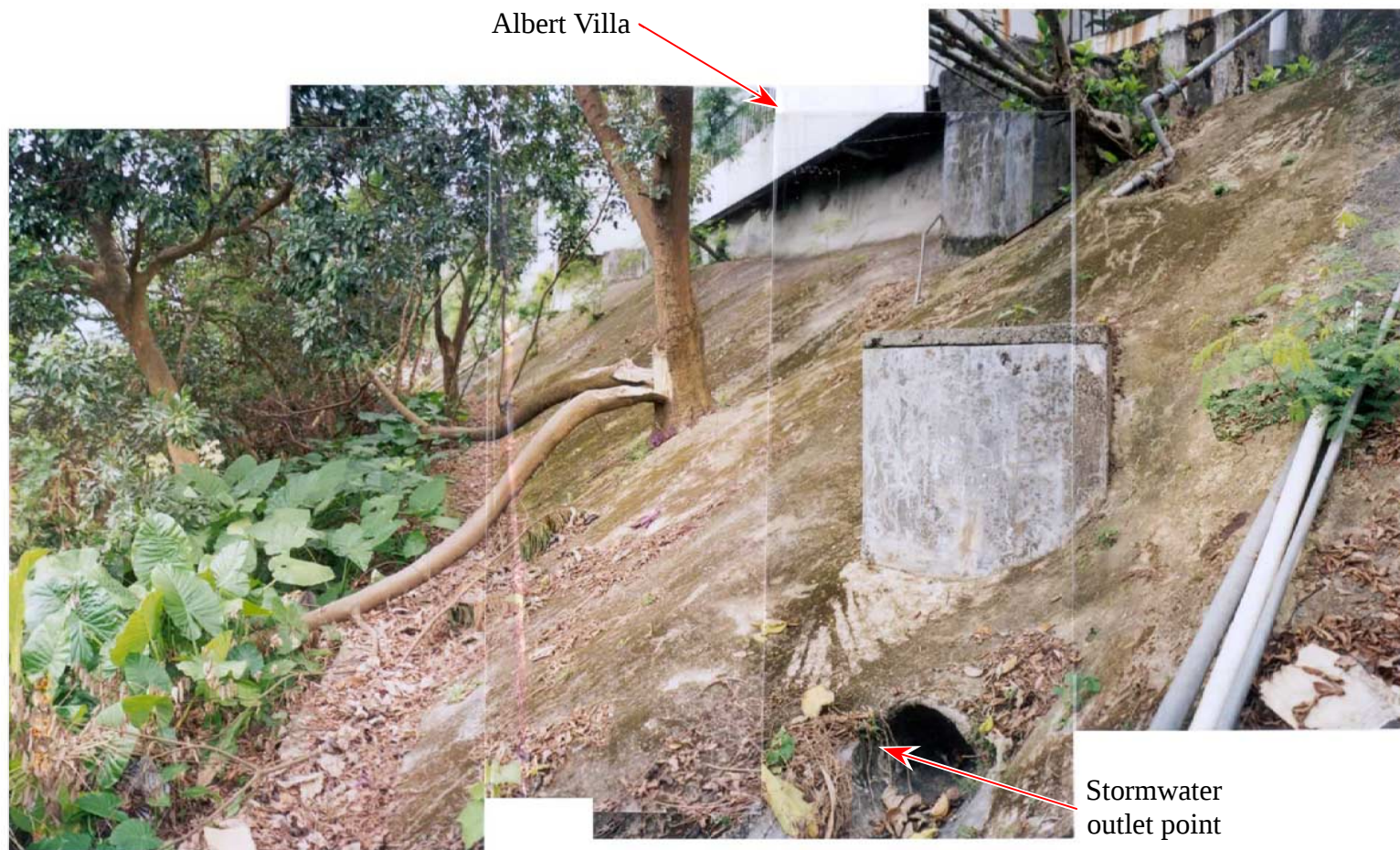
Plate 12 - Stormwater Outlet from Albert Villa (Photograph Taken on 12 October 1999)
