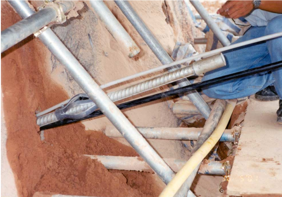
Plate 1 - Inserting the Steel Soil Nail with the Plastic Tube into a Drillhole
