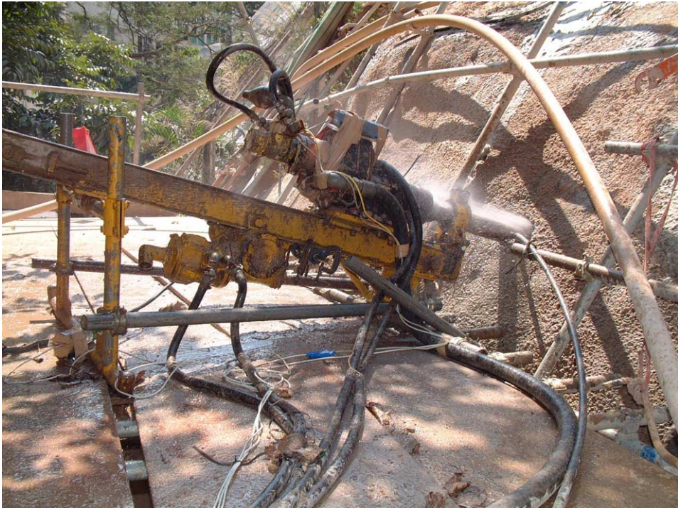
Plate 3 - Drilling Rig Equipped with the DPM
