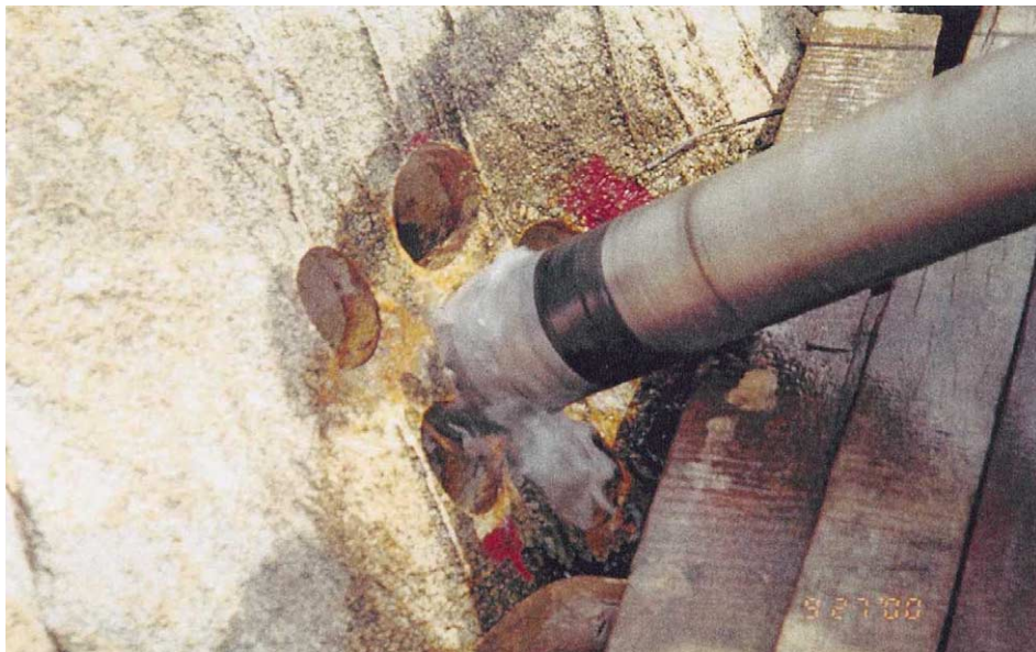
Plate 14 - Stitch Drilling around a Steel Soil Nail
