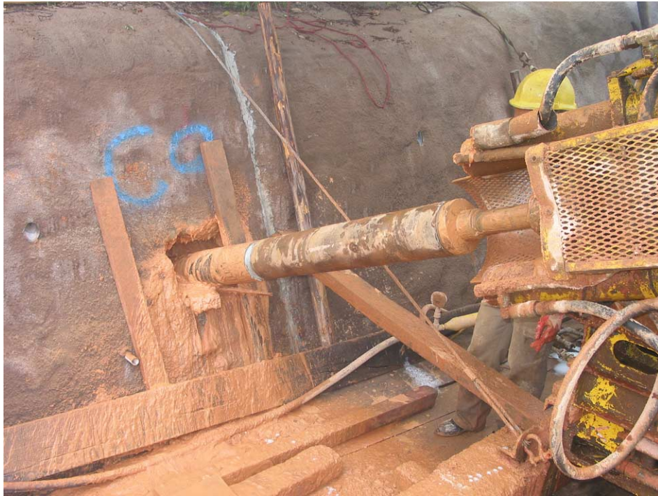
Plate 15 - Over-coring of a Steel Soil Nail
