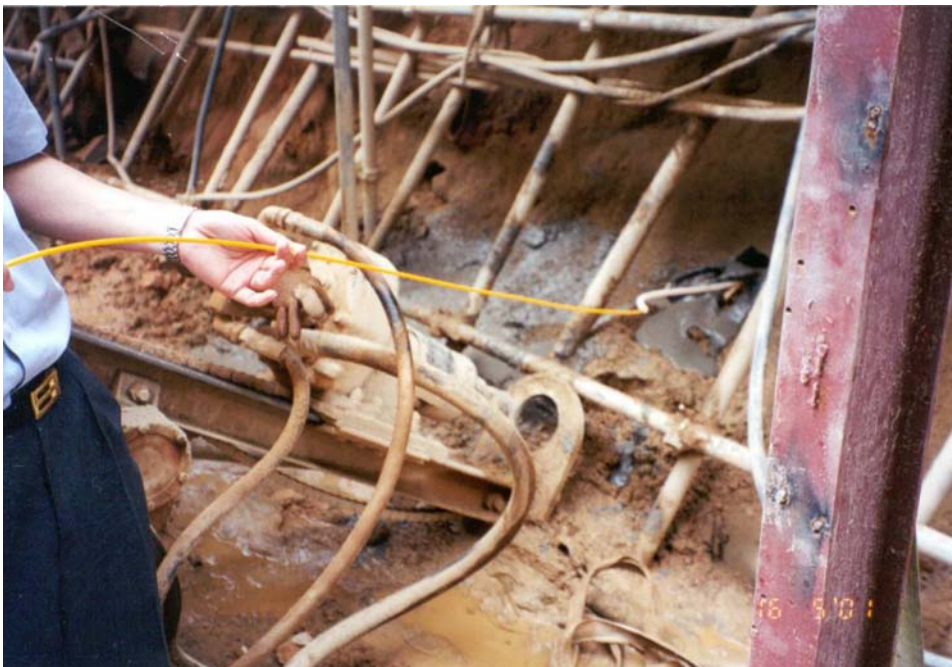
Plate 2 - Measuring the Length of Drillhole by Inserting a Flexible Plastic Rod into the Plastic Tube
