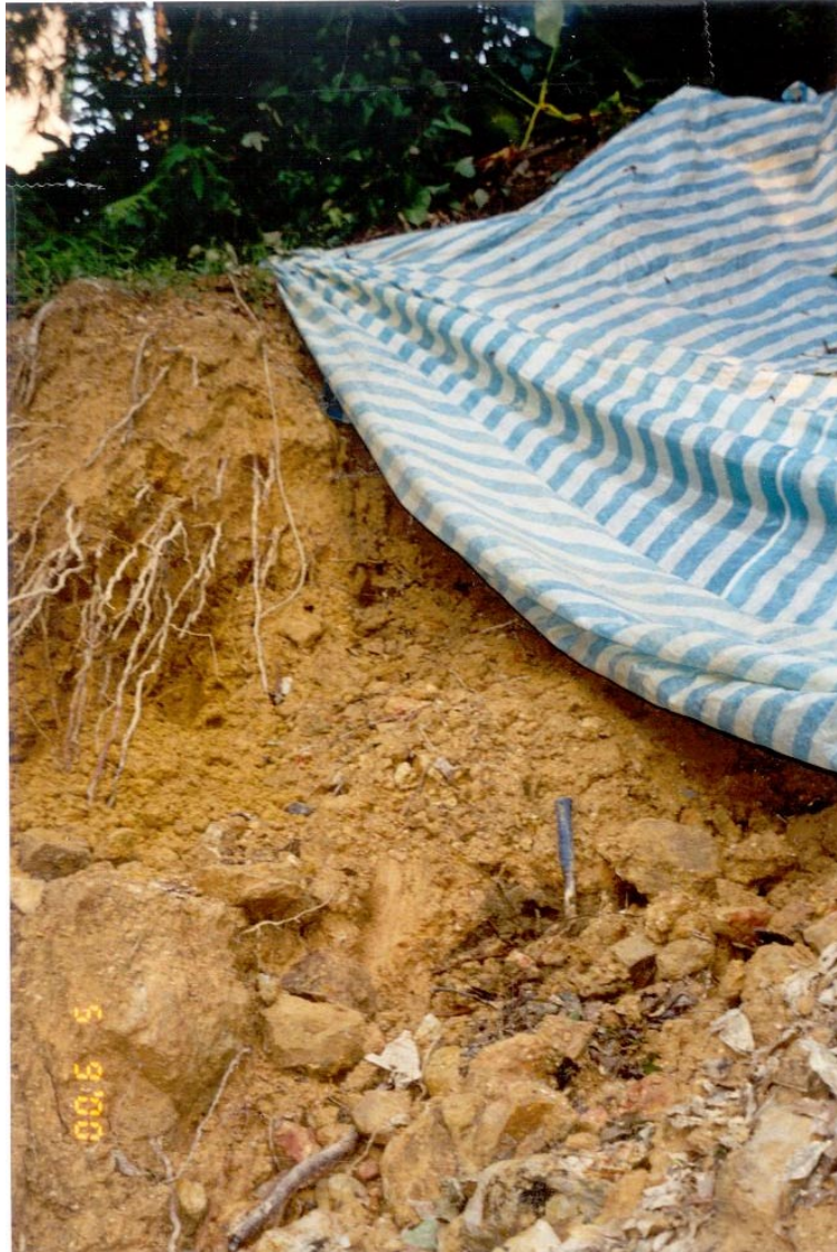
Plate 12 - Close View of Main Scarp Showing Exposed Fill Material (Photograph Taken on 9 September 2000. Note Old Topsoil Horizon Exposed in Base of Scarp at Location of Geological Hammer)
