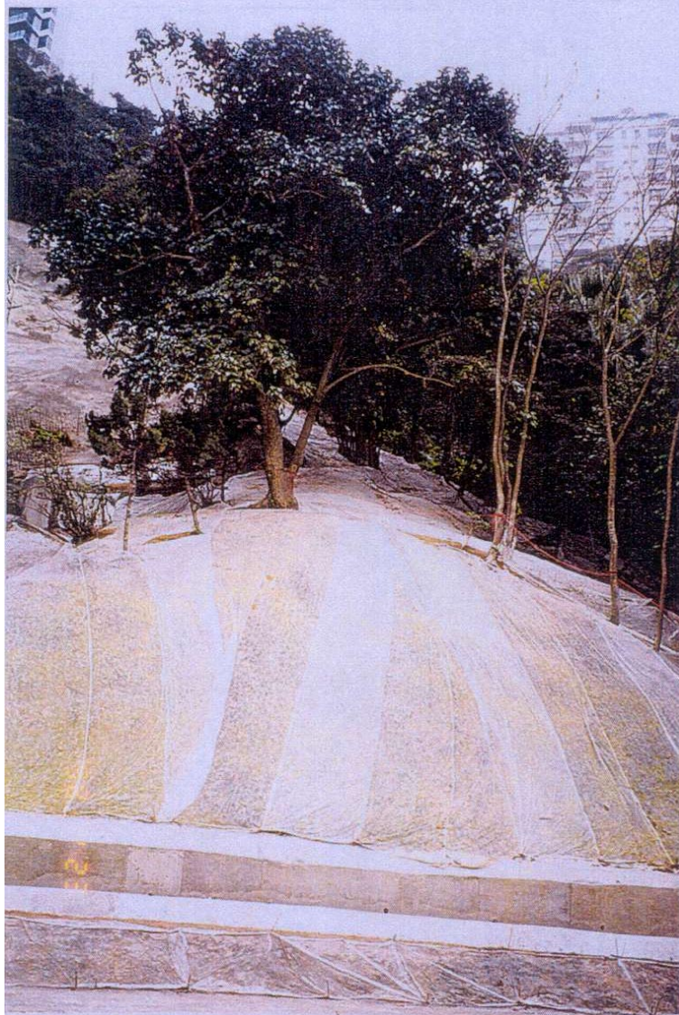
Plate 3 - View South from Bowen Road towards Newly Hydroseeded Slope No. 11SW-B/C179 and Western “Green Hatched Black” Area (Extract from CMW (1998b))
