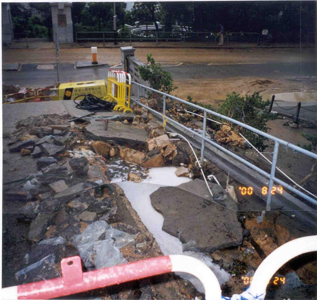
Plate 11 - View North along Covered Nullah at Kennedy Road Showing Cover Slabs Having Been Lifted and Broken by Force of Water and Debris (Photograph Taken on 24 August 2000)
