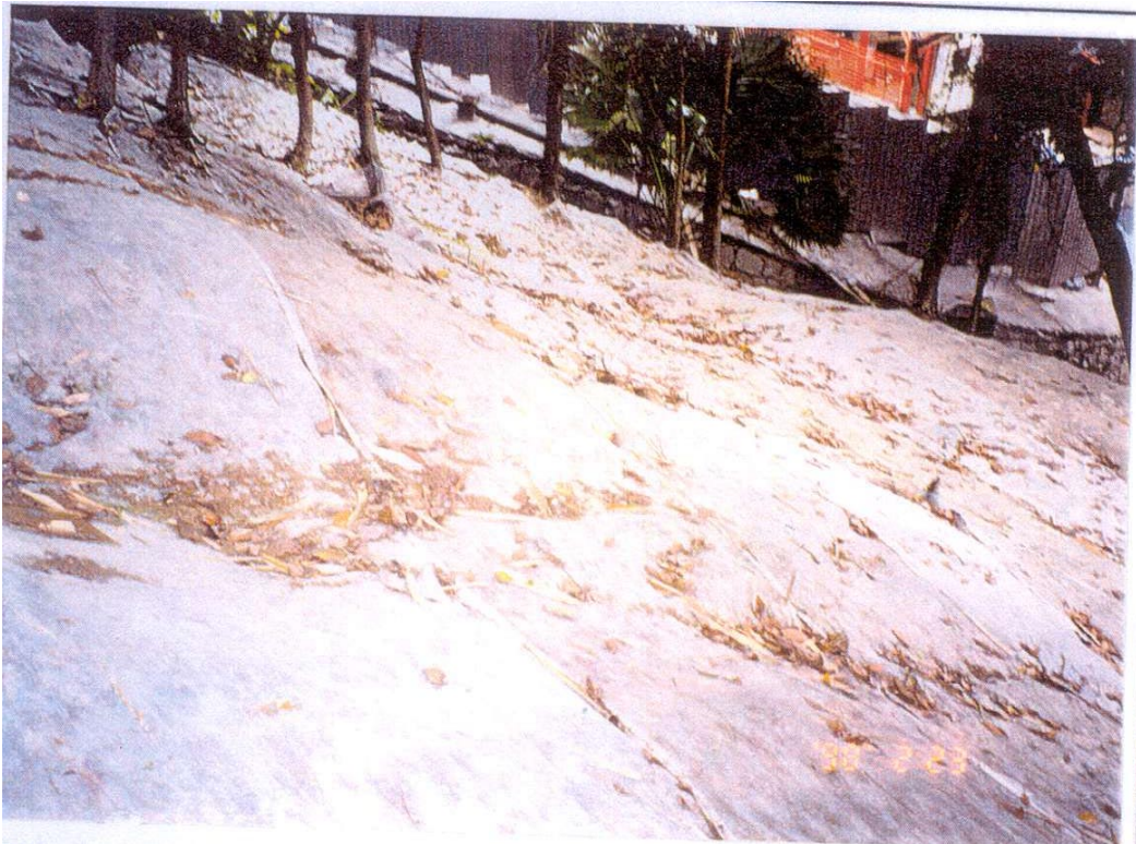
Plate 5 - View Northwest towards Nullah across Location of August 2000 Landslide Scar Showing Newly Hydroseeded Western “Green Hatched Black” Area (Extract from CMW (1998b))
