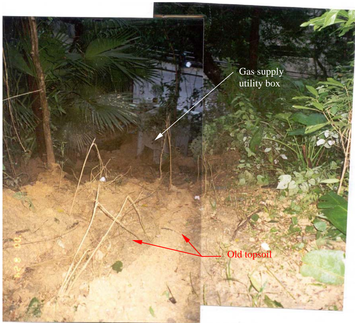
Plate 6 - View Northwest down Landslide Scar from Main Scarp (Photograph Taken on 24 August 2000. Note Old Topsoil Horizon Exposed in Channels Scoured in Fill)
