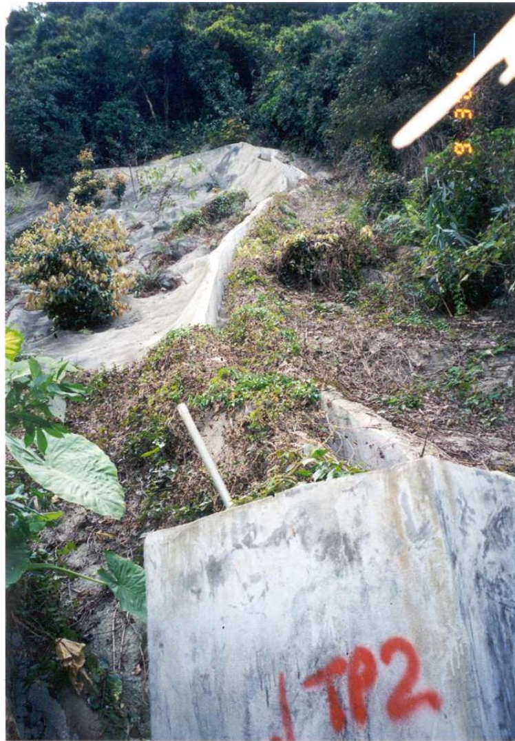
Plate 8 - View South from Catchpit above August 2000 Landslide Scar Showing Steeply Inclined 450 mm Crest U-channel of Slope No. 11SW-B/C180 (Photograph Taken on 9 March 2001)
