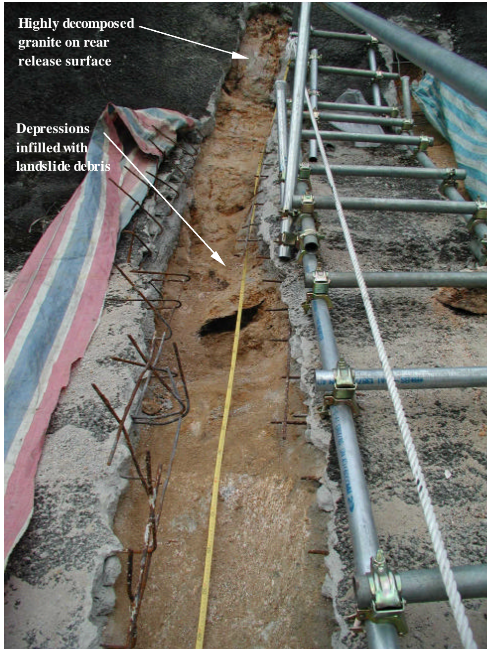
Plate 15 - View of Surface Strip SS1 Revealing Completely to Highly Decomposed Granite at the 1993 Landslide Scar (Photograph Taken on 27 December 2000)
