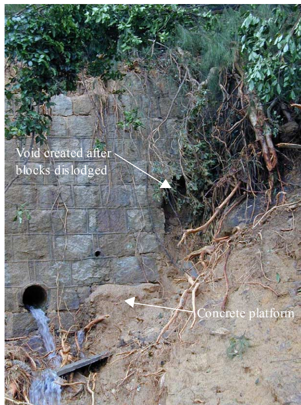
Plate 9 - View Showing Northern End of the Masonry Toe Wall and Location from Where Masonry Blocks have been Dislodged (Photograph Taken on 24 August 2000)
