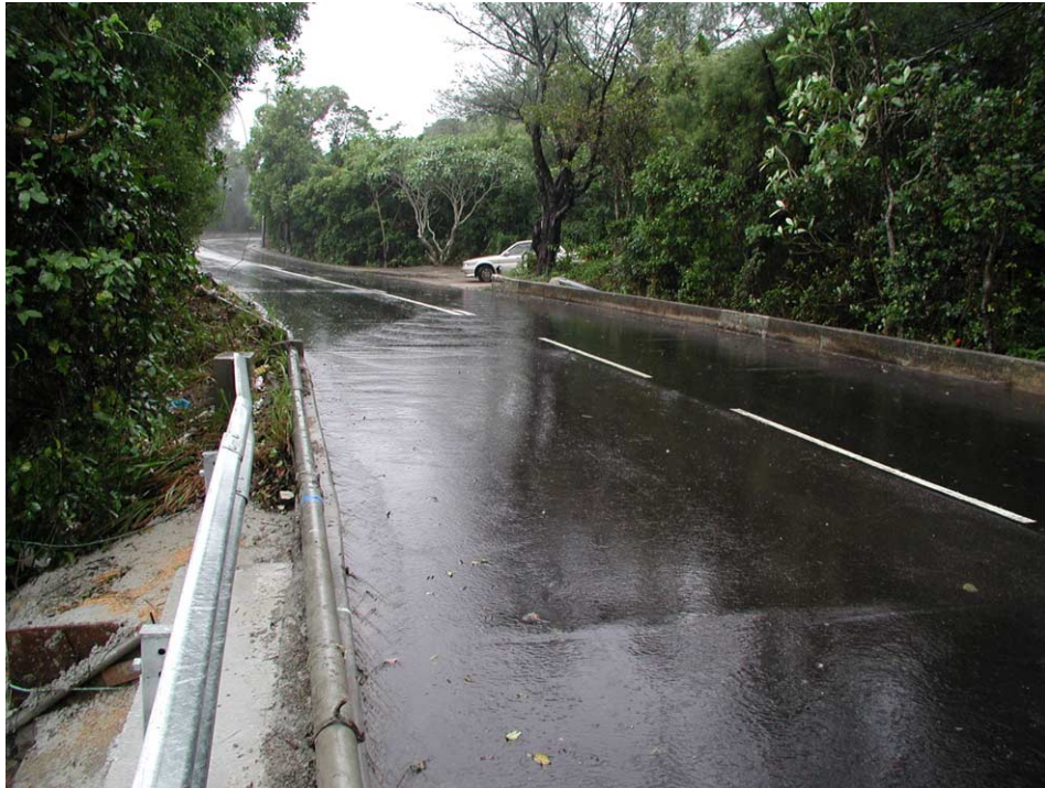
Plate 5 - Water Flowing from Access Road to No. 18 Shek O Road towards Slope No. 15NE-B/FR123 (Photograph Taken on 20 October 2000)
