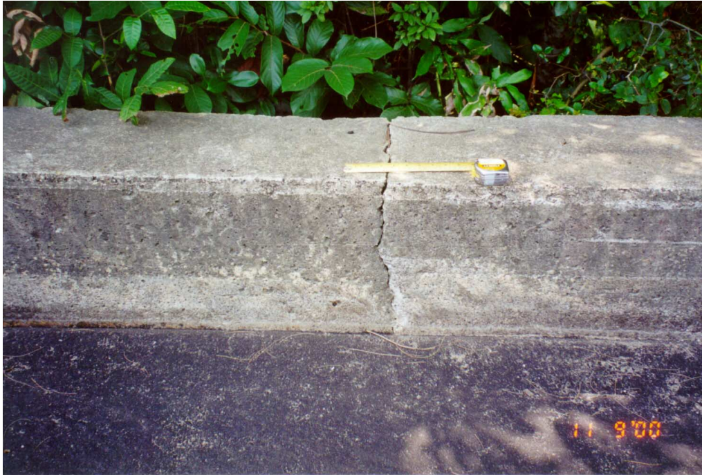
Plate 11 - View Showing the Crack on Kerb on the Northbound Lane of Shek O Road (Photograph Taken on 11 September 2000)
