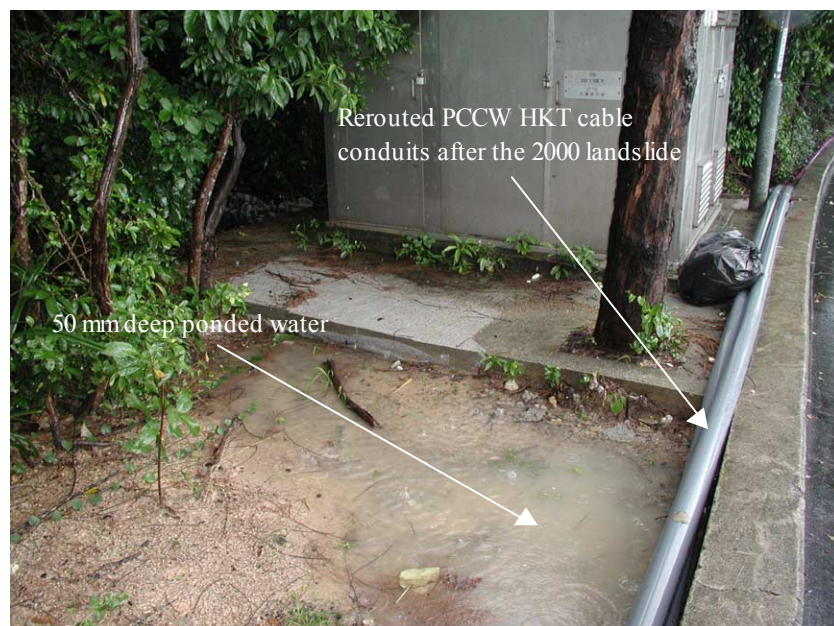
Plate 10 - Ponding Water Adjacent to HEC Transformer Pillar (Photograph Taken on 20 October 2000)
