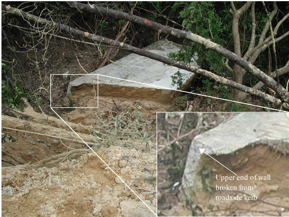
Plate 7 - General View of the Collapsed Retaining Wall (Photograph Taken on 29 August 2000)
