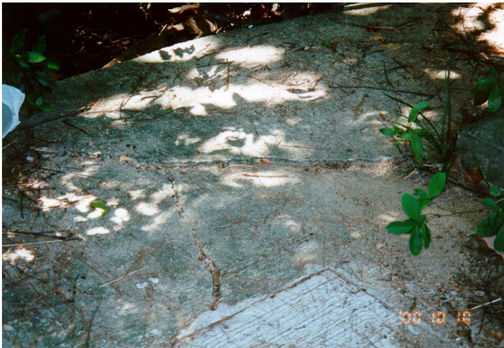
Plate 12 - The Cracks with Maximum Width of 10 mm on the Concrete Foundation Pad of HEC Transformer Pillar (Photograph Taken on 10 October 2000)
