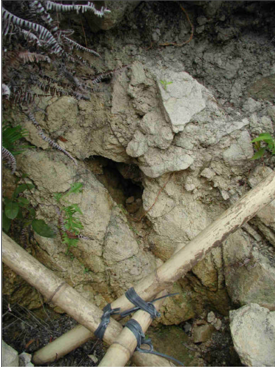
Plate 21 - Erosion Pipe Located Below the Crown of Landslide B (Photograph taken on 12 October 2000)
