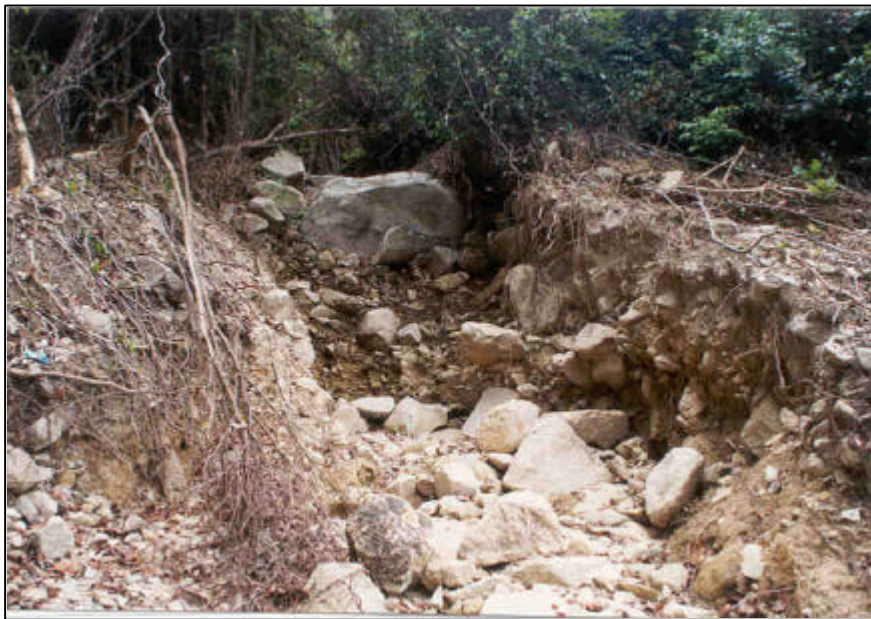
Plate 29 - View of Eroded Channel within the Colluvium Substrate (Note the 2 m Diameter Boulder at Chainage 250. Photograph taken on 6 June 2000)
