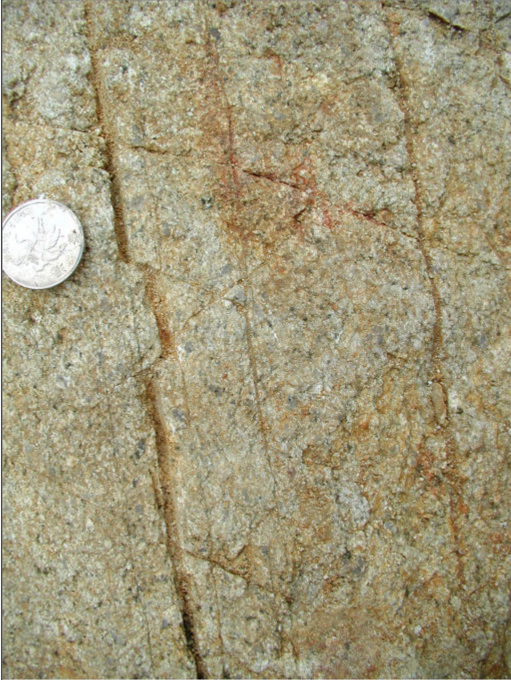
Plate 14 - Detail of Offset Clay Infilled Joint on the Floor of Landslide B (Photograph taken on 12 October 2000)
