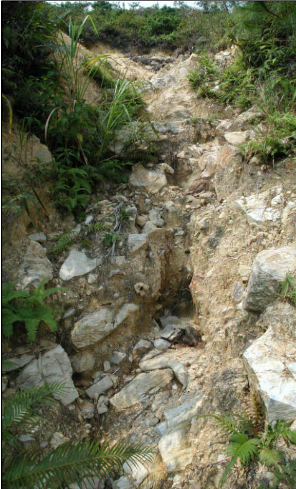
Plate 35 - View of Eroded Channel within Mining Waste Located Directly Below the Source Area of Landslide C (Photograph taken on 18 September 2000)
