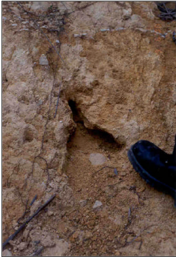
Plate 34 - Erosion Pipe with V-shaped Washout Feature Below (Photograph taken on 9 June 2000)
