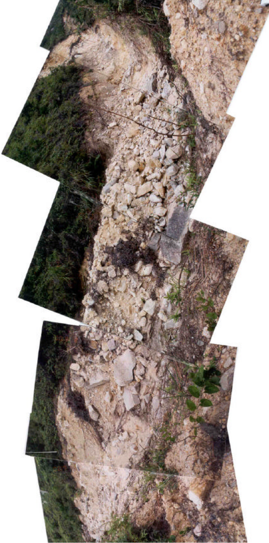
Plate 26 - Possible Breached Dam Below Landslide B Between Chainages 65 and 95 (Photograph taken on 8 June 2000)
