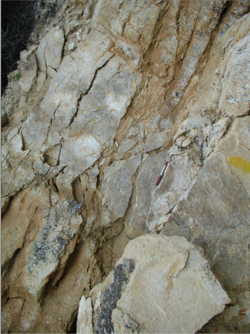
Plate 18 - Detail of Open and Sediment-infilled Joints Exposed on the Eastern Release Surface (Photograph taken on 14 July 2000)
