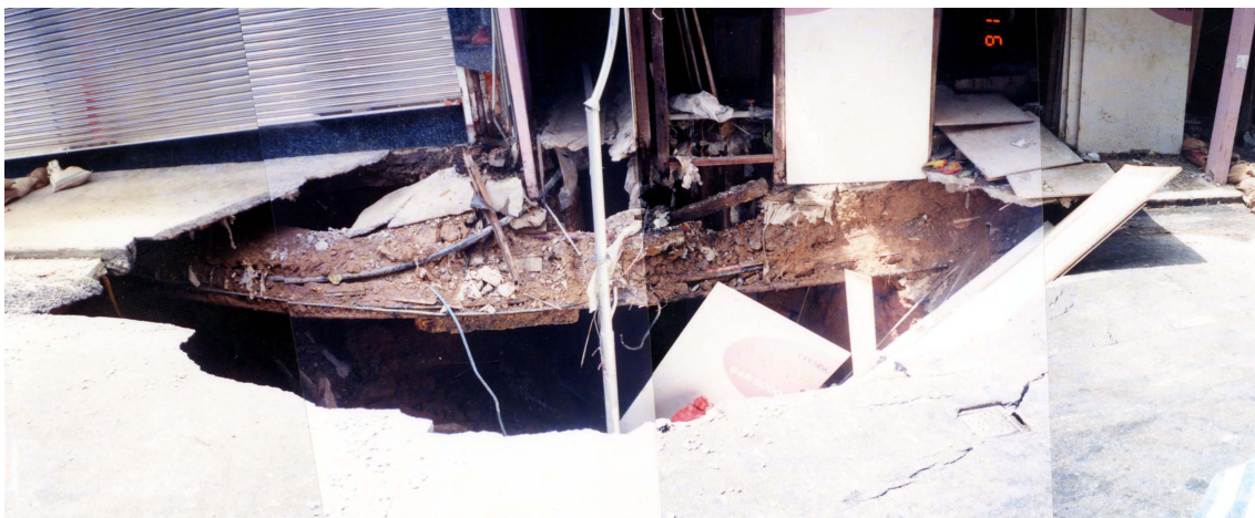
Plate 3.4 - Collapse of Mau Lam Street, Hong Kong June 1991
