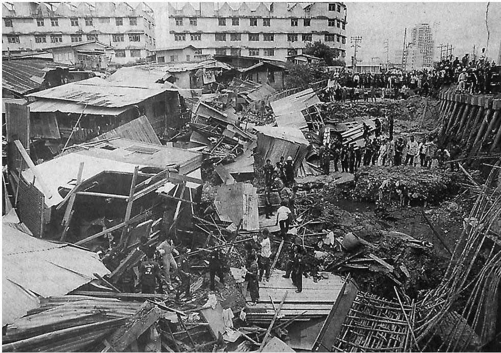
Plate 3.1 - Failed Cofferdam Bangkok 1998
