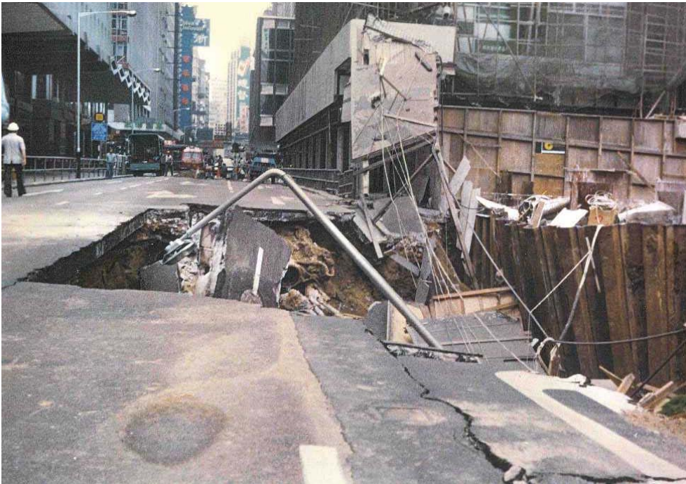
Plate 4.1 - Collapse of Queen's Road Central
