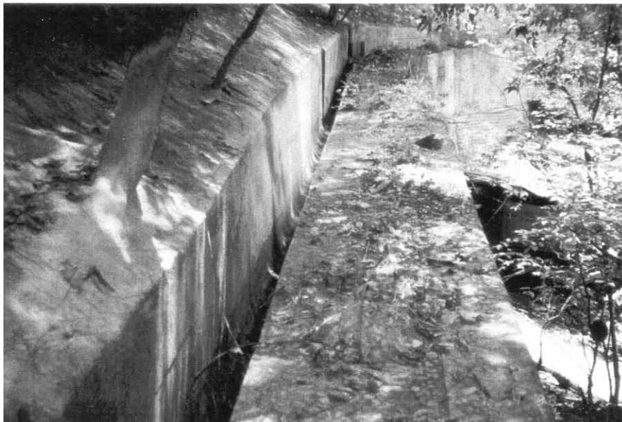
Plate L – View of Repaired Upstand Wall at the Toe of the Slope (Record Photograph Extracted from HyD Report on RMI of 17 April 1998)
