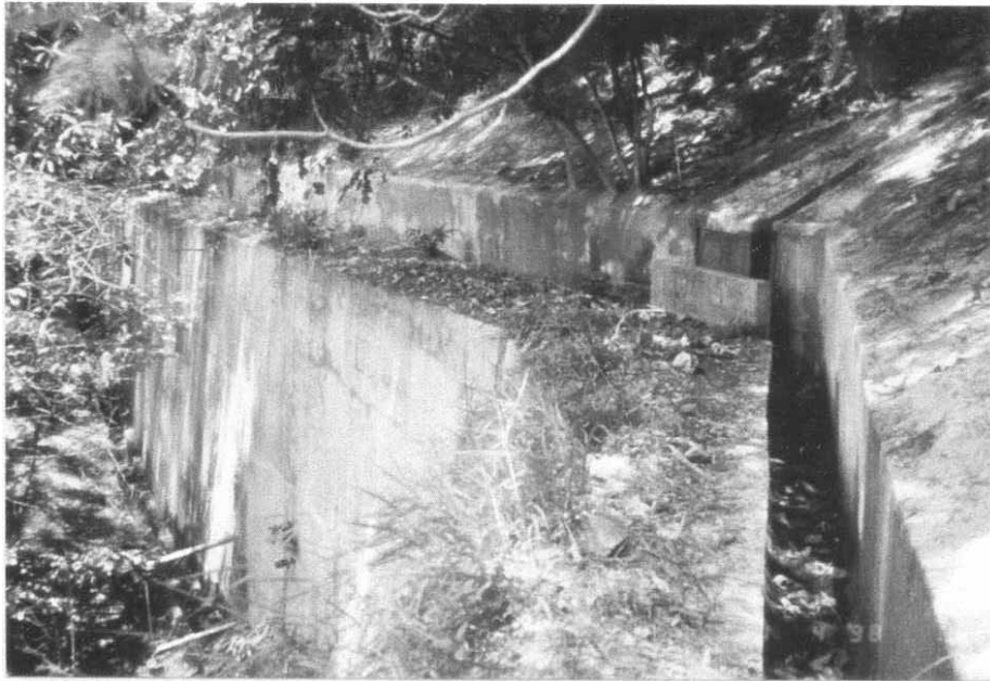
Plate K – View of Repaired Upstand Wall at the Toe of the Slope (Record Photograph Extracted from HyD Report on RMI of 17 April 1998)
