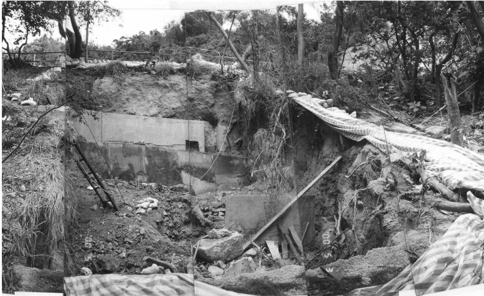
Plate 15 – View of Concrete Buttress Built to Support the Trough after the Incident (Photograph Taken on 3 May 2000)
