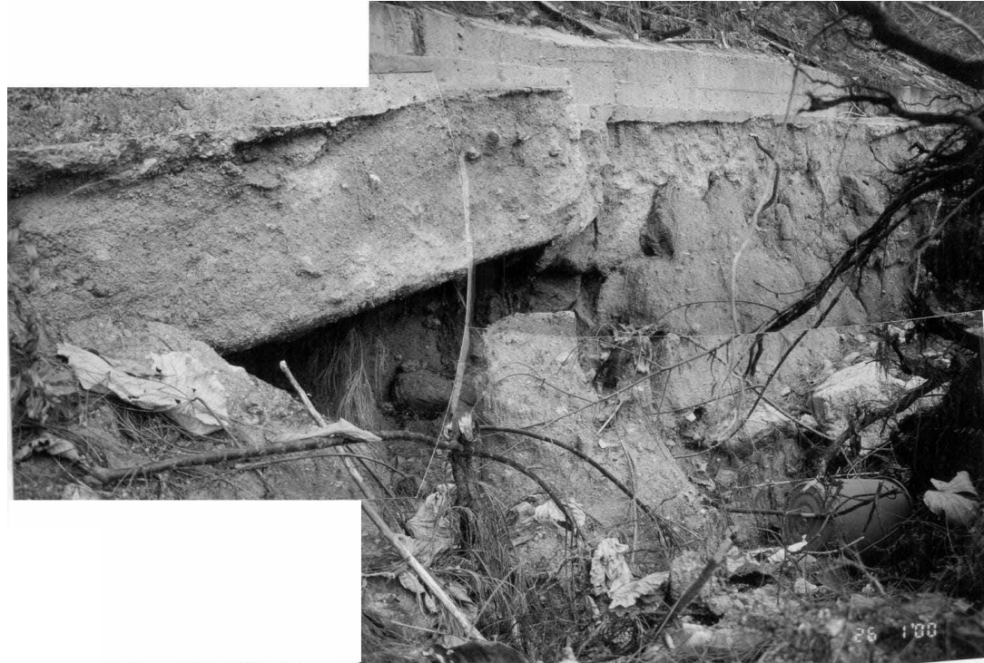
Plate 9 – Subsurface Void in the Lowest Batter to the Southwest of the Main Scar (Photograph Taken on 26 January 2000)
