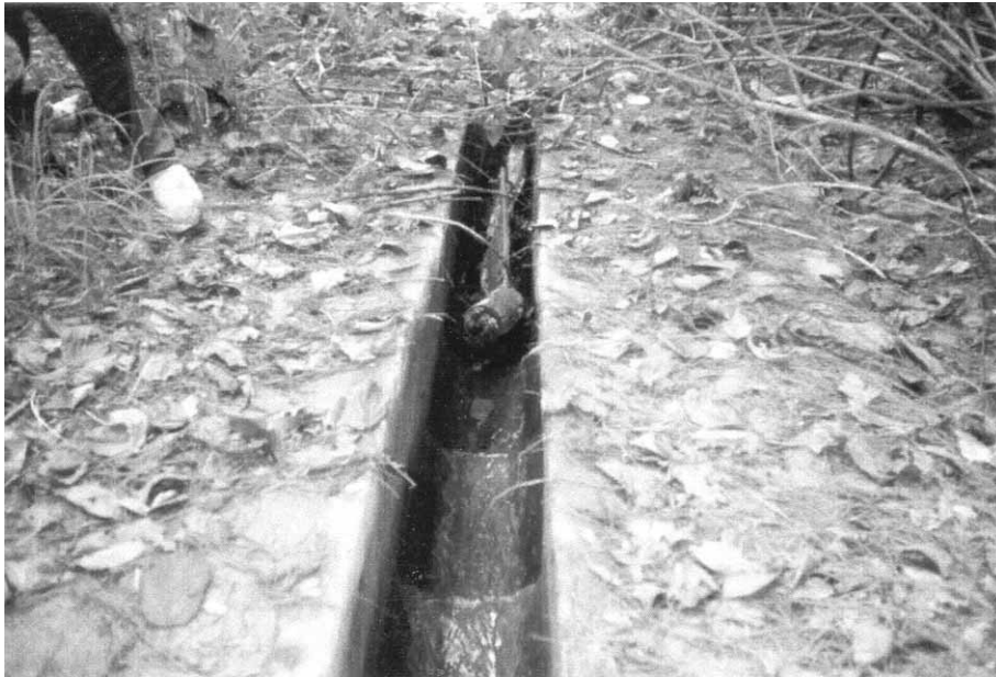
Plate I – View of Partly Blocked Channel (Record Photograph Extracted from HyD Report on RMI of 14 April 1997)
