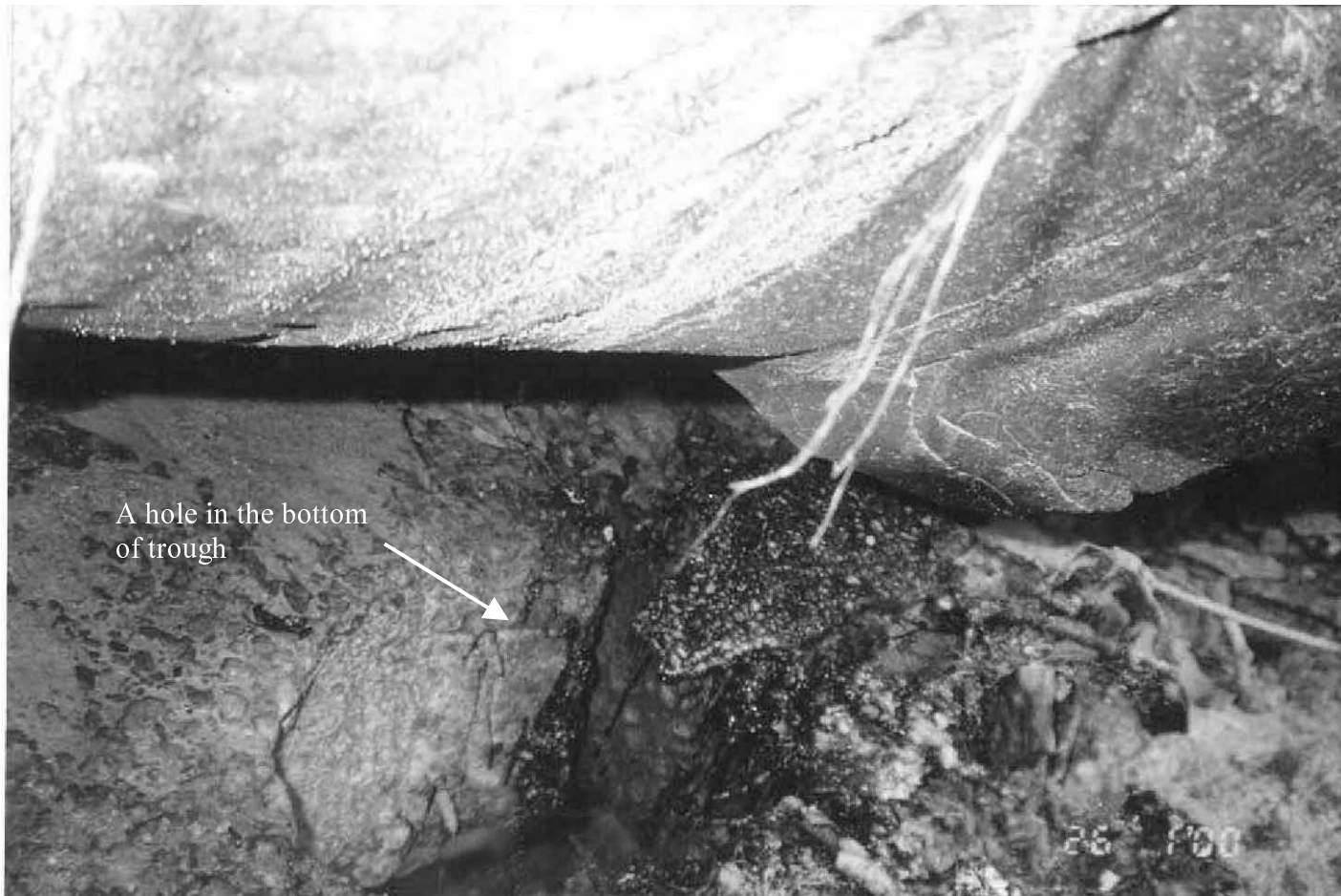
Plate 11 – View of the Hole at the Bottom of Trough (Photograph Taken on 26 January 2000)
