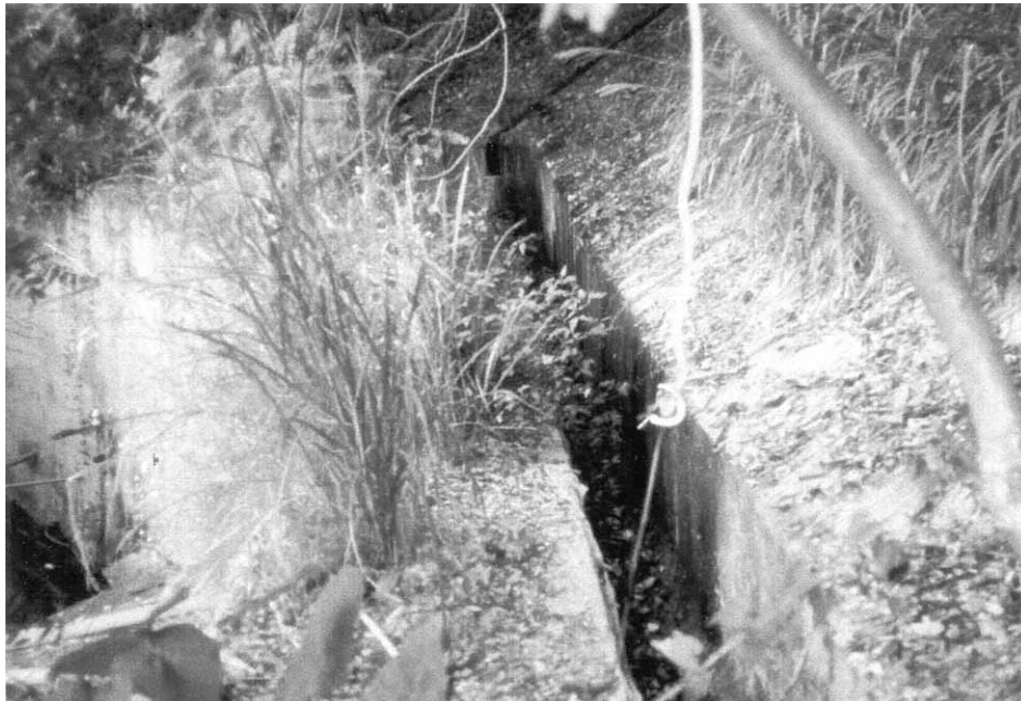
Plate N – View of Seepage at the Toe of the Slope (Record Photograph Extracted from HyD Report on RMI of 14 January 1999)
