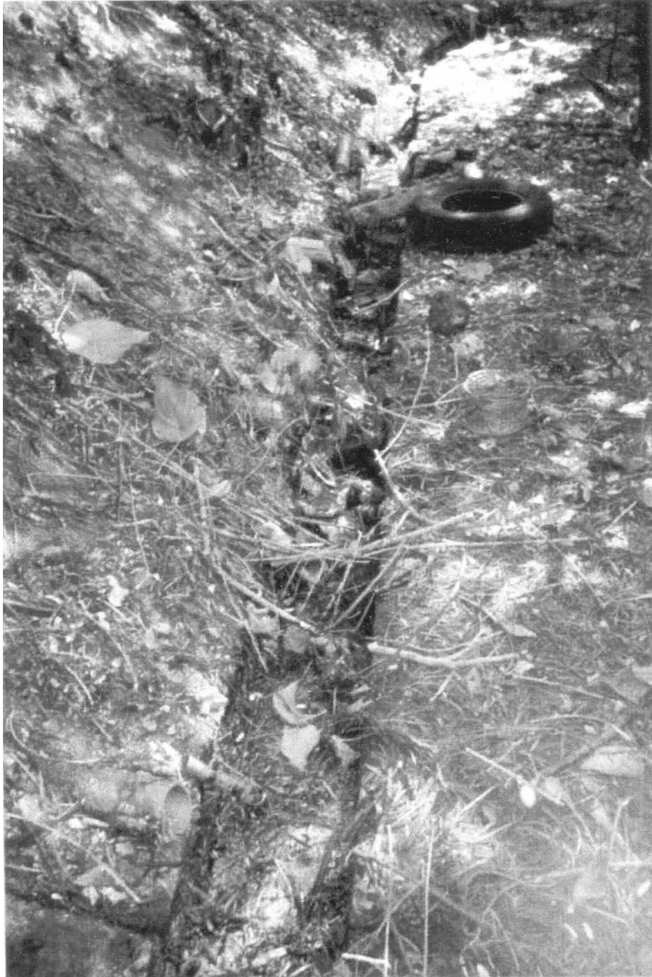
Plate B – View of Blocked Drainage Channel (Record Photograph Extracted from HyD Report on RMI of 1 November 1996)
