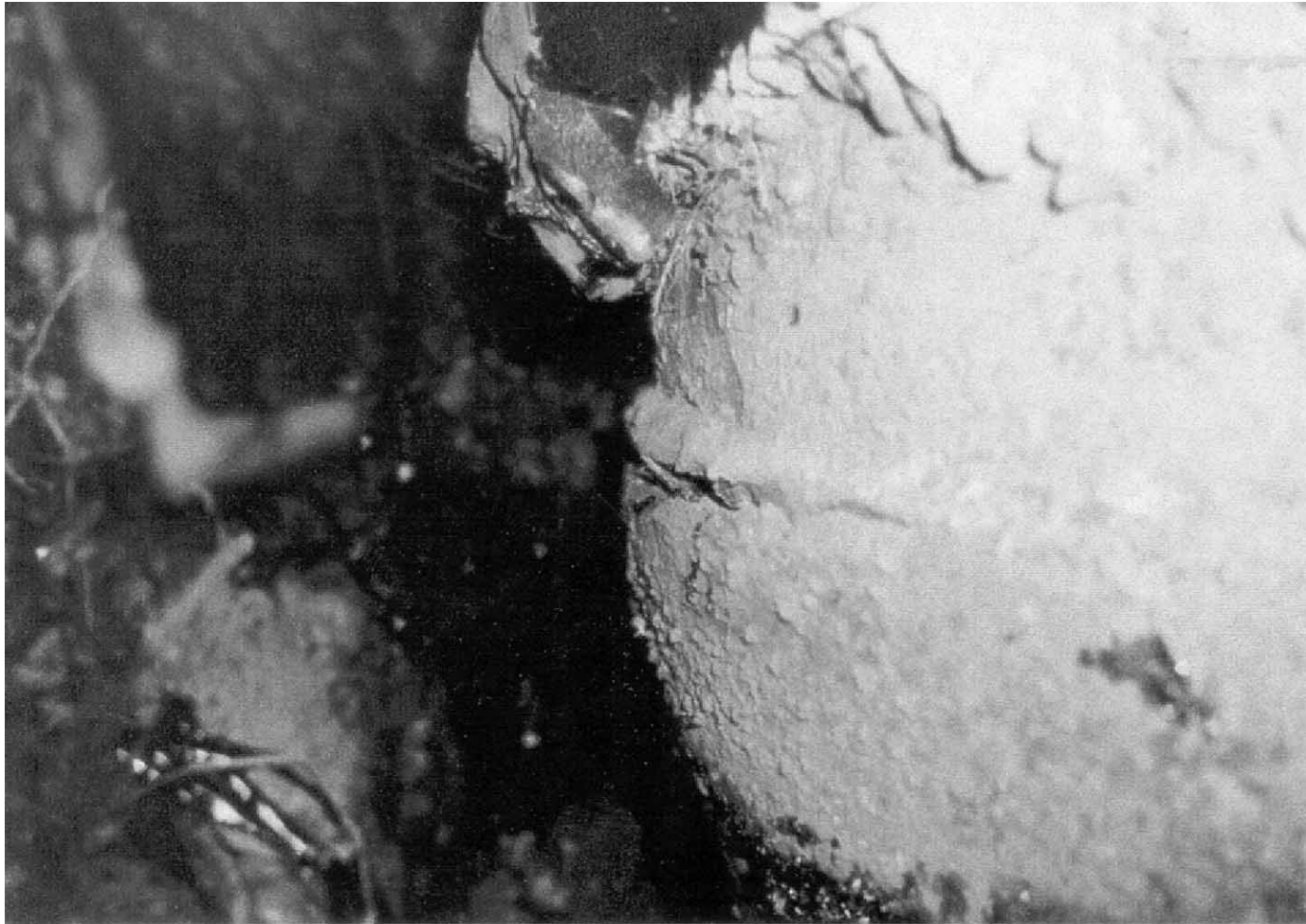
Plate 14 – Close-up View of the Crack along the Welded Joint (Photograph Taken by WSD on 15 January 2000)
