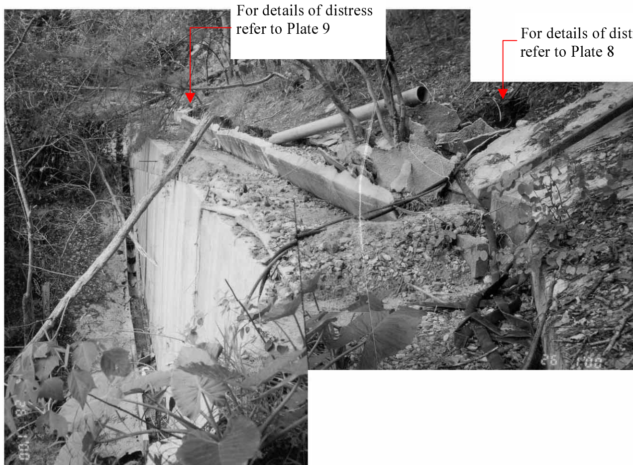
Plate 10 – Tilted Upstand Wall at the Toe of the Lowest Batter (Photograph Taken on 26 January 2000)
