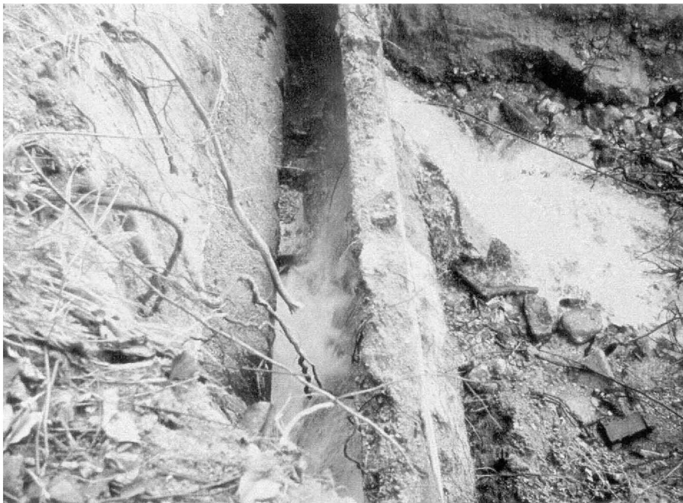
Plate 6 – View of Leaking Pipe at the Time of Inspection by WSD (Photograph Taken on 15 January 2000)
