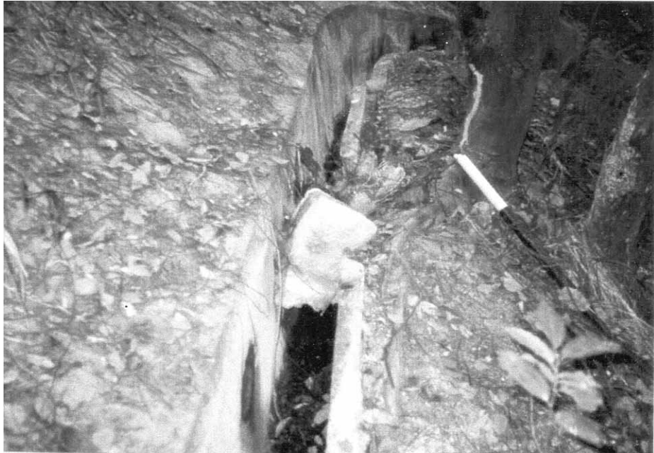
Plate M – View of Slight Seepage/Dampness at the Discharge Point of the Overflow Pipe (Record Photograph Extracted from HyD Report on RMI of 14 January 1999)
