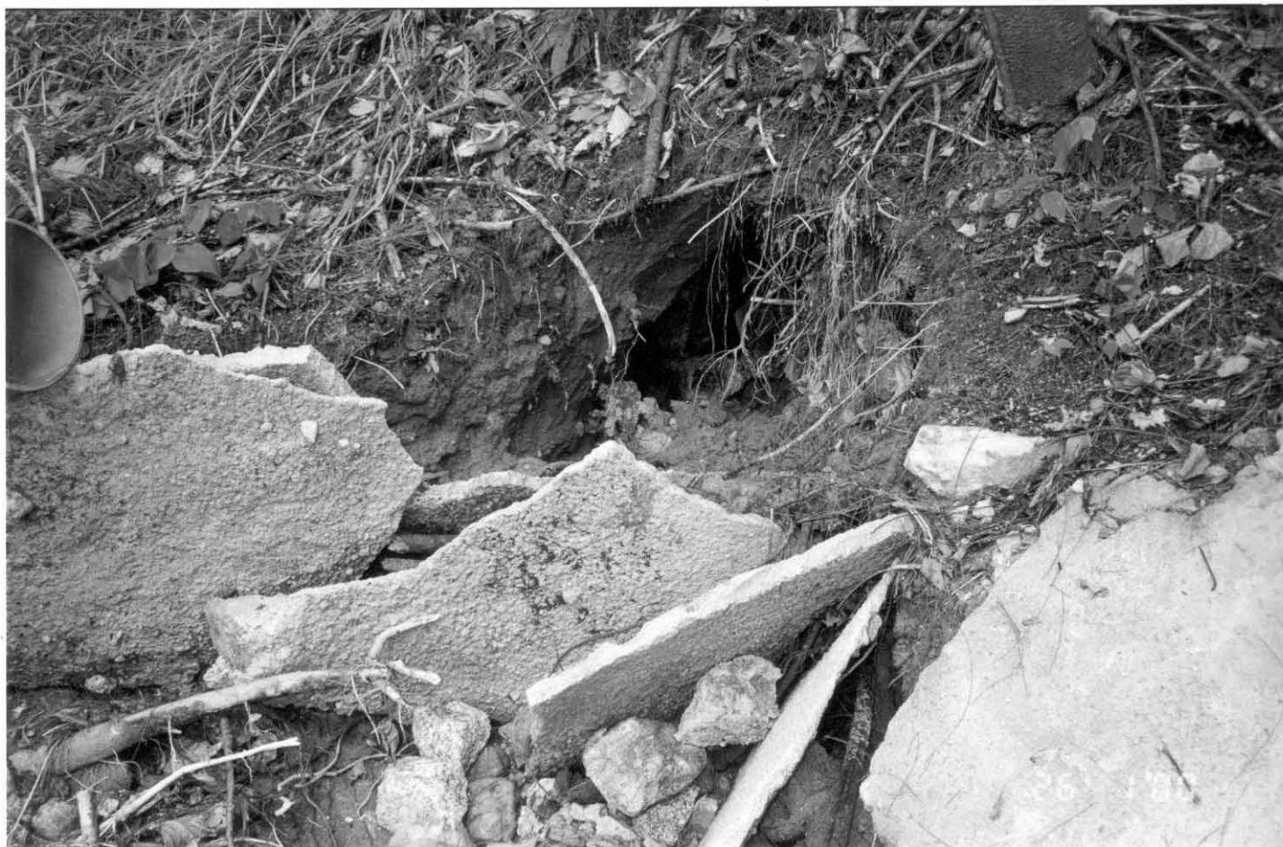
Plate 8 – Subsurface Void (approx. 0.6 m in diameter) in the Lowest Batter of the Slope below the Main Scar (Photograph Taken on 26 January 2000)
