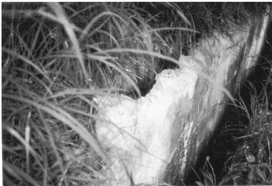
Plate J – View of Tilting Upstand Wall at the Toe of the Slope (Record Photograph Extracted from HyD Report on RMI of 14 April 1997)
