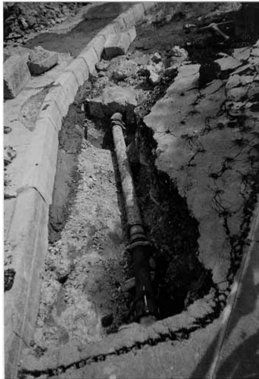
Plate 19 – Repair Works Effectuated to 75 mm Diameter Fire Services Main Following Identification of Additional Leak (Photograph Taken on 5 August 1999)
