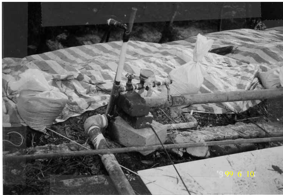
Plate 12 – Local Arrangement of Services at Slope Crest above Landslide. Note Temporary Spigots (Photograph Taken on 10 June 1999)
