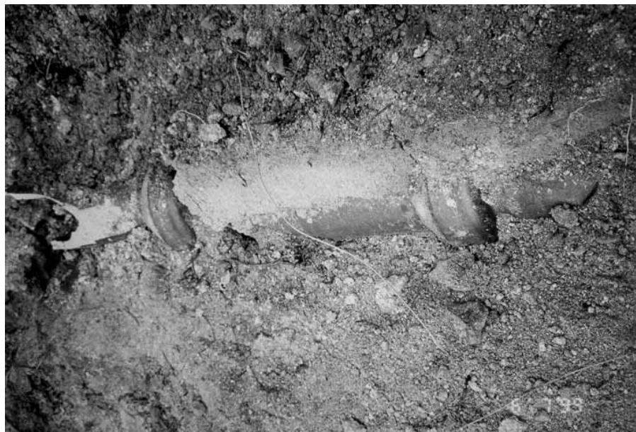
Plate 10 – Intact Length of Foulwater Sewer in Landslide Debris (Photograph Taken on 6 July 1999)
