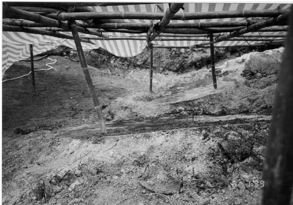
Plate 8 – Intact Portions of Chunam Surfacing on Displaced Blocks of Debris near Northern Flank. Transition to Southern-Facing Portion of Slope Visible on Left of Frame (Photograph Taken on 6 July 1999)
