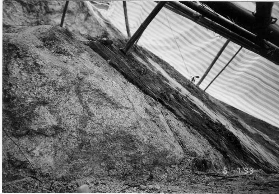
Plate 7 – Intact Portion of Chunam Surfacing on Displaced Debris Block (Photograph Taken on 6 July 1999)
