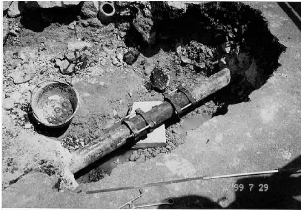
Plate 17 – Repair Works Effected to 75 mm Diameter Fire Services Main (Photograph Taken on 29 July 1999)
