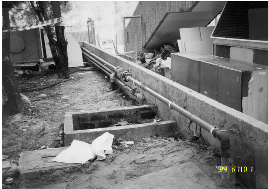
Plate 11 – View South across Crest Area above Landslide Scar Indicating Arrangement of Pipework. Valves and Fittings Appear New (Photograph Taken on 10 June 1999)
