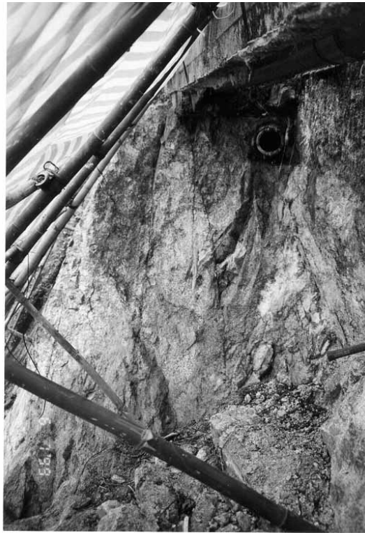
Plate 9 – Southern Flank of Scar Showing Sub-Vertical Main Scarp Coincident with Relic Joint Surfaces. Severed Foulwater Sewer Visible beneath Intact Berm U-Channel Upstand. Western Wall of Sewer Trench Coincident with Main Scarp. Kaolin-Rich Zone Visible in Centre-Right of Frame (Photograph Taken on 6 July 1999)
