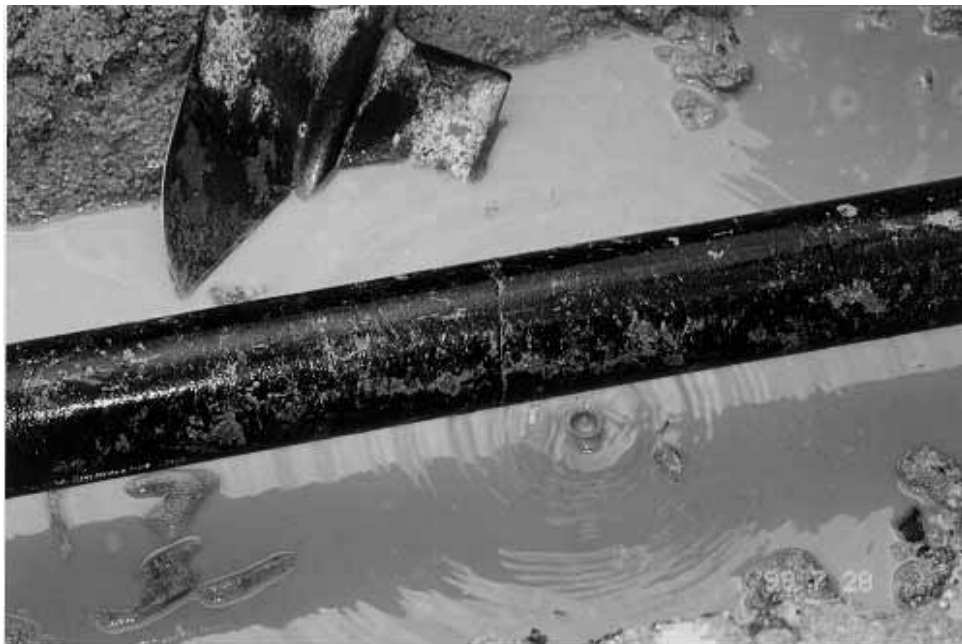
Plate 16 – Leak Identified in 75 mm Diameter Fire Services Main within Driveway at Slope Crest (Photograph Taken on 28 July 1999)
