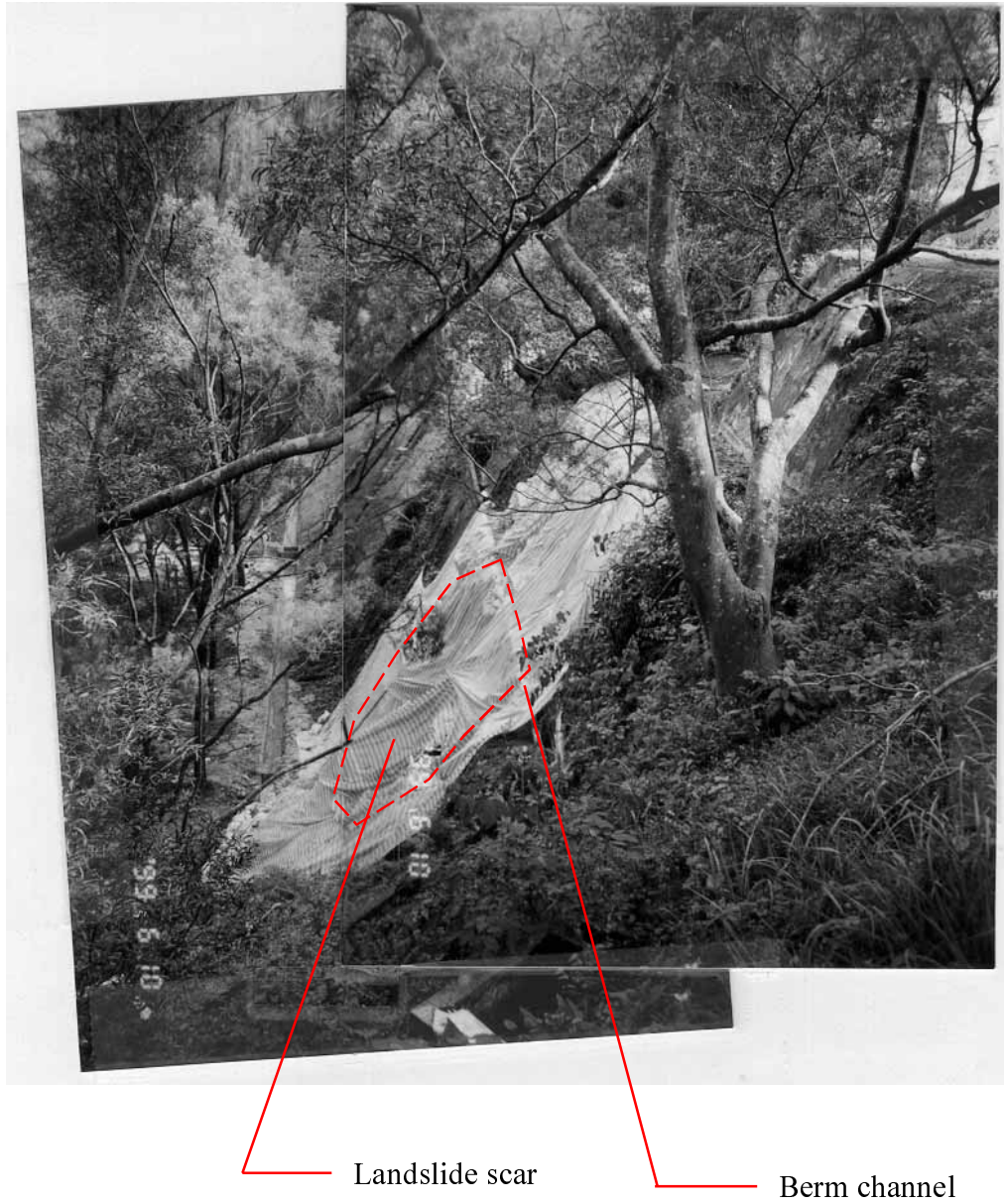
Plate 1 – General View South across Slope No. 7NE-C/C23 and Landslide Location, Obscured by Plastic Sheeting. Berm Channel at Main Scarp Indicated. Slope above Not Affected (Photograph Taken on 10 June 1999)
