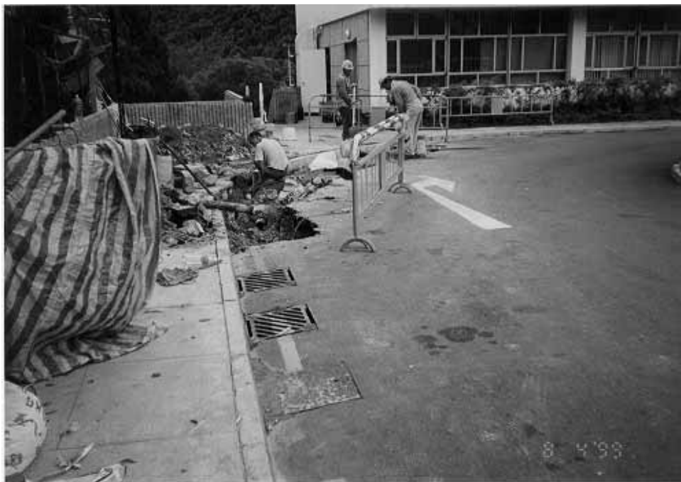
Plate 18 – Excavation of Driveway Pavement Following Second Incidence of Damage by Heavy Vehicle. Additional Leak in 75 mm Diameter Fire Services Main Identified During Pavement Repair Works (Photograph Taken on 4 August 1999)
