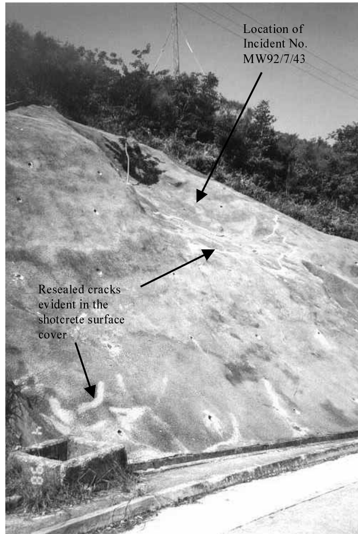
Plate 4 – View of Slope No. 9SW-D/C115 Showing Concave Depression Following a Landslide in 1992 (GEO Incident No. MW1999/7/43) (Photograph Taken on 4 November 1998)
