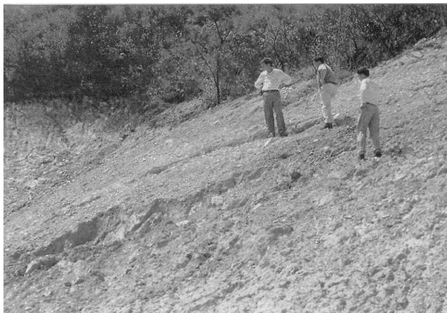
Plate 6 - View of Minor Failure and Exposed Soil Pipe in Reggraded Portion of Slope (Photograph Taken on 22 September 1992)
