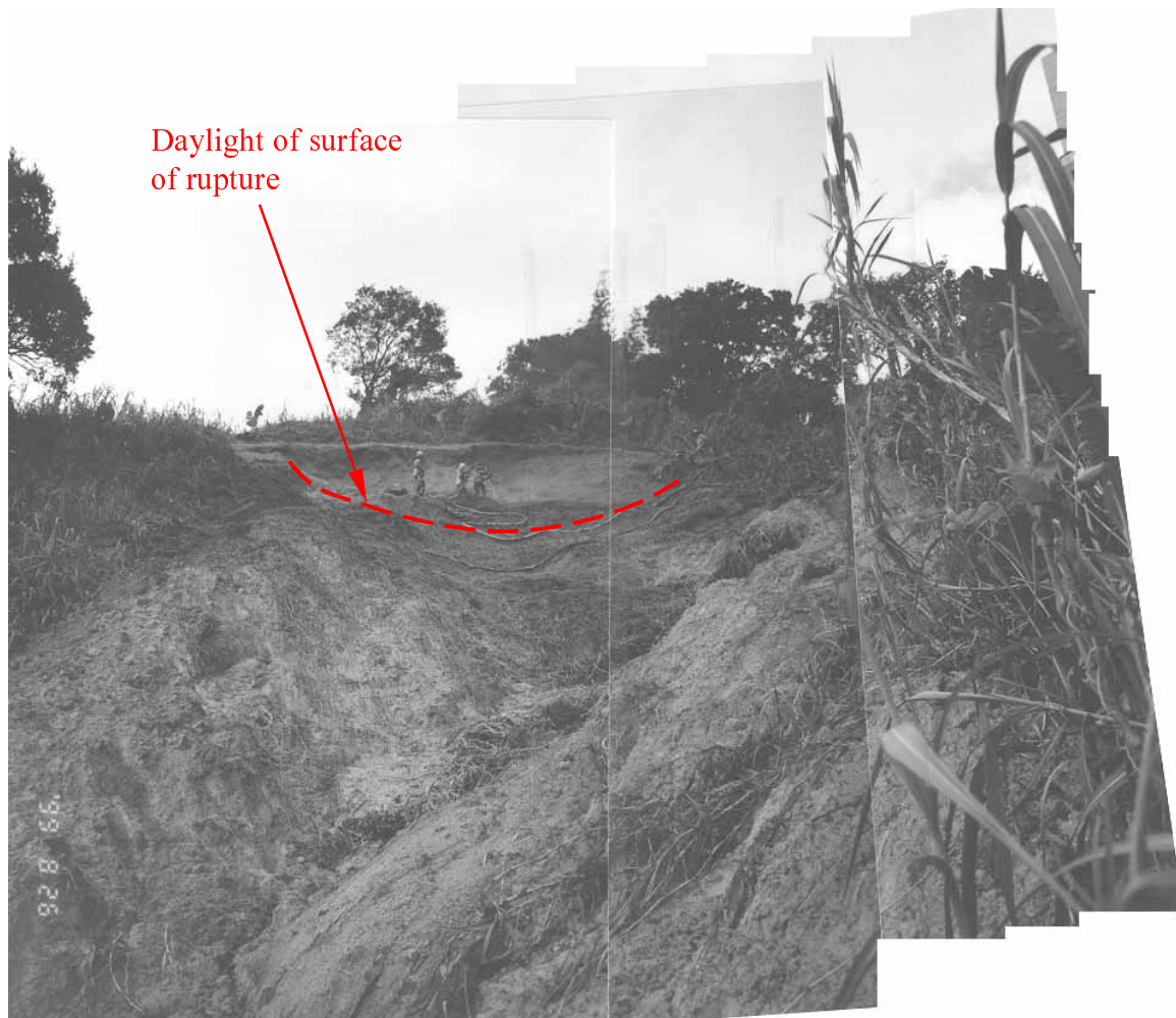
Plate 14 – View North up Landslide B from above Point of Confluence. Shotcreting Works Underway. Note Overhang of Main Scarp. Intact Vegetation in Scar in Foreground Suggests Source Area Largely Confined to Portion Already Shotcreted (Estimated Daylight Indicated). Note also Erosion Gully in Base of Drainage Line Traversing Scar in Foreground (Photograph Taken on 26 August 1999)
