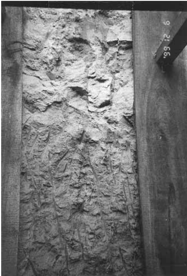
Plate 22 – Trial Pit TP1: General View Showing Relic Joints in Grade IV Tuff Infilled with Grade V Material (Photograph Taken on 6 December 1999)
