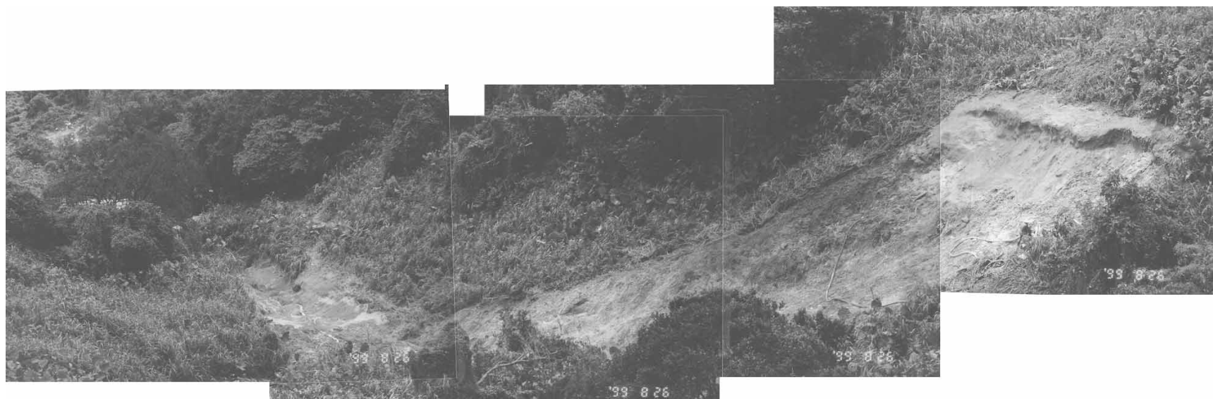
Plate 13 – View West across Landslide B from VTC Building. Shotcreting Works in Progress. Note Apparent Layer Separation in Main Scarp Producing Overhang. Note also Darker Superficial Material Remaining in Scar (Photograph Taken on 26 August 1999)
