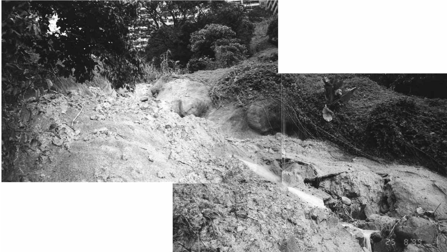
Plate 11 – View North-East up Landslide Scar from above Crest of Slope No. 11SW-C/C531 Exposing Previous Application of Shotcrete to Ephemeral Stream Course and Drainage Line No. 4 above Victoria Road (Photograph Taken on 25 August 1999)
