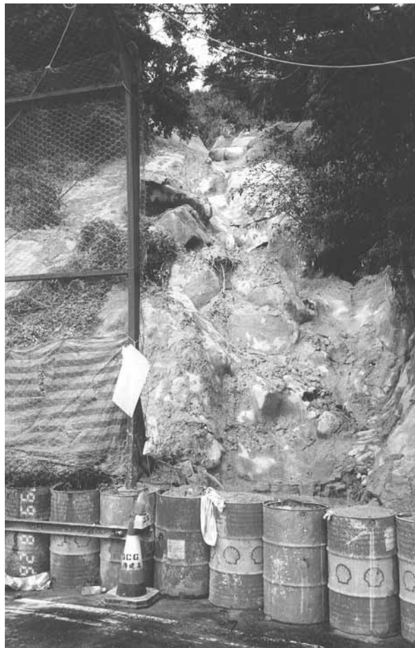
Plate 10 – View North–East up Landslide Scar from Victoria Road. Slope No. 11SW-C/C531 in Foreground. Note Random Orientation of Large Blocks in Slope to Suggest Previous Instability (Photograph Taken on 26 August 1999)
