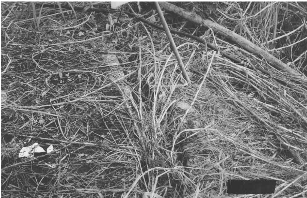
Plate 17 – 250 mm U-Channel Located above Main Scarp of Landslide A Overgrown and Blocked by Vegetation (Photograph taken on 25 August 1999)
