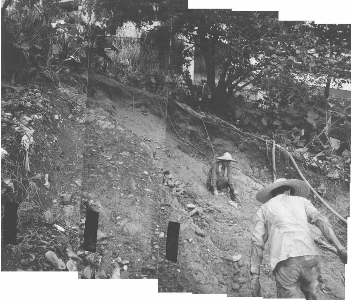
Plate 5 – View East across Main Scarp and Southern Flank of Landslide A. Note Definition of Scarp and Flank, Exposed Fill in Flanks and Clear Line of Interface with Natural Ground Below. Note also Refuse Content of Fill (Photograph Taken on 26 August 1999)
