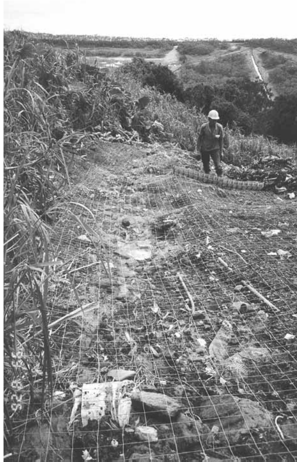
Plate 8 – View South-West down Landslide A. Note Shallow Sectional Geometry of Scar and Exposure of Natural Ground on Left of Frame (Photograph Taken on 26 August 1999)
