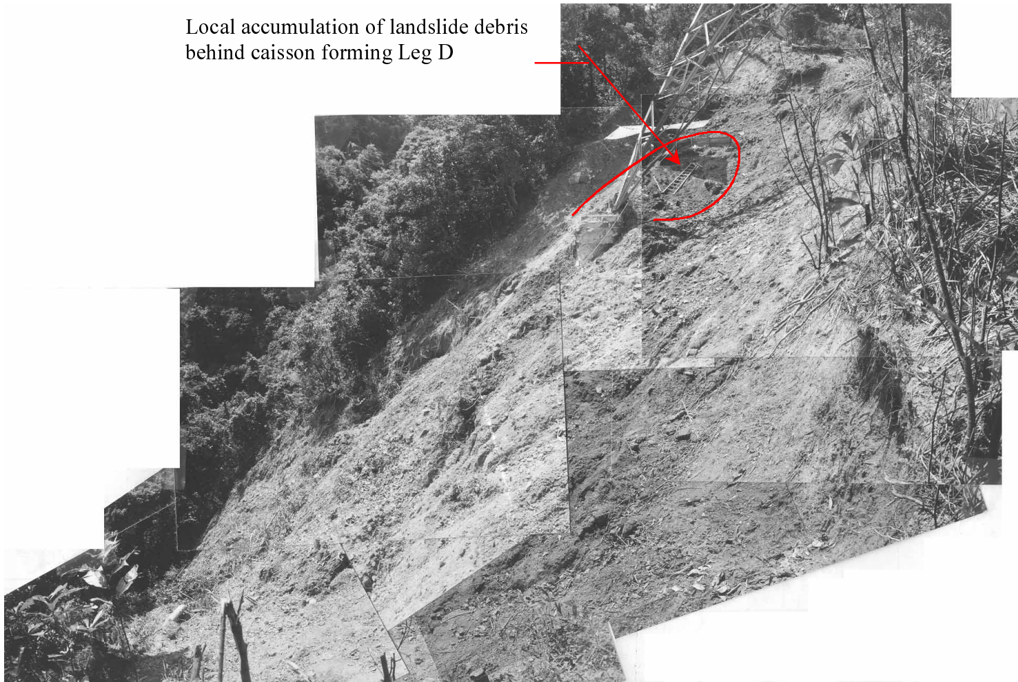
Plate 5 – General View of the Upper Portion of the Landslide Looking South (Photograph Taken on 23 September 1999)
