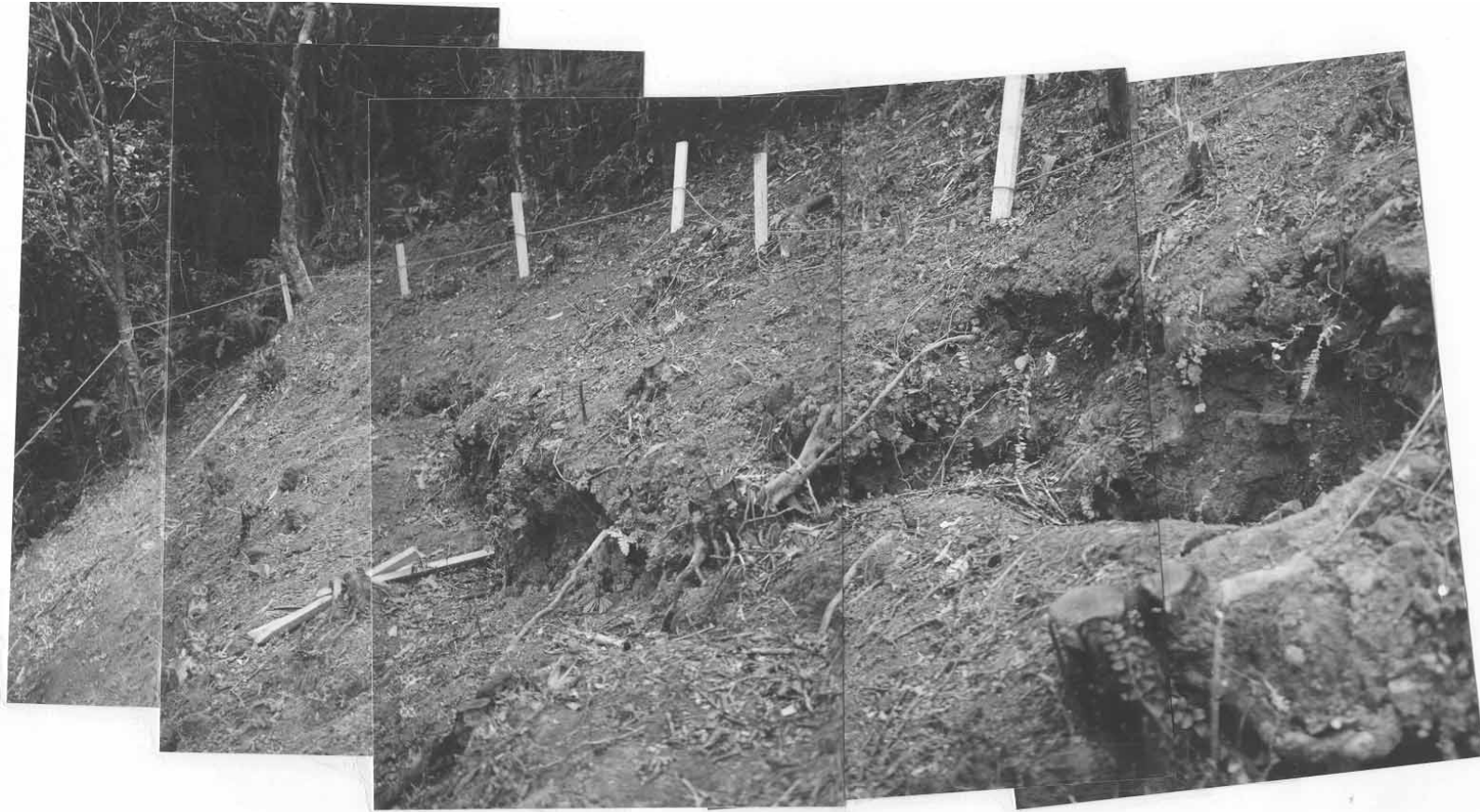
Plate 8 – Pre-existing Tension Crack Located on the Slope above the Crest of the Landslide Scar (Photograph Taken on 8 September 1999. See Figure 11 for Location)
