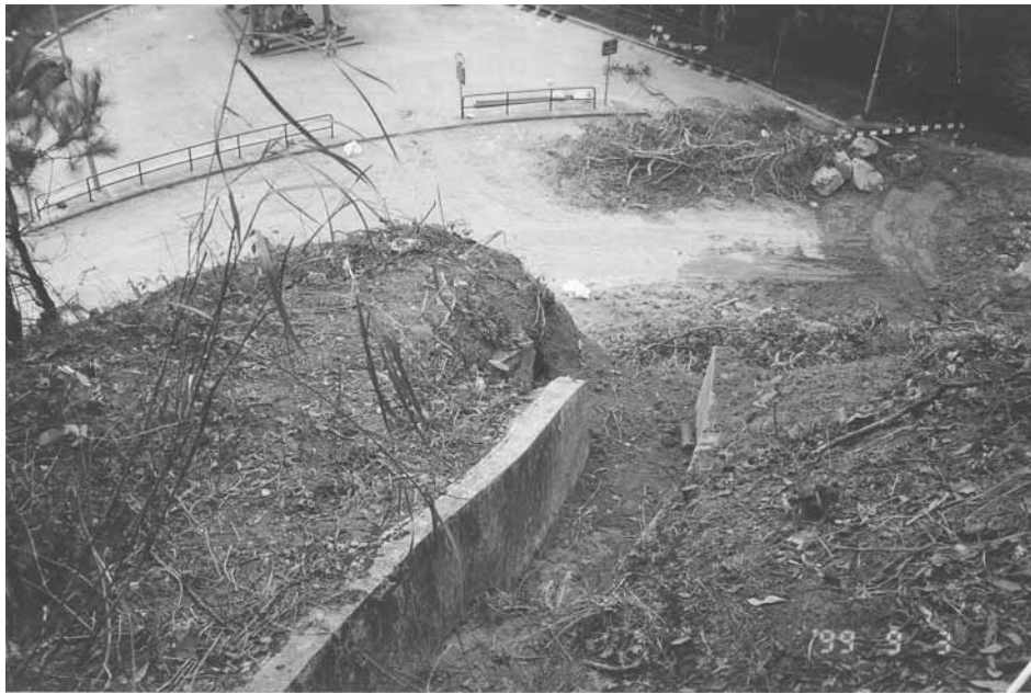
Plate 4 – Dislocated Trapezoidal Drainage Channel above the Western Flank of the Main Scarp (Photograph Taken on 3 September 1999. See Figure 11 for Location)
