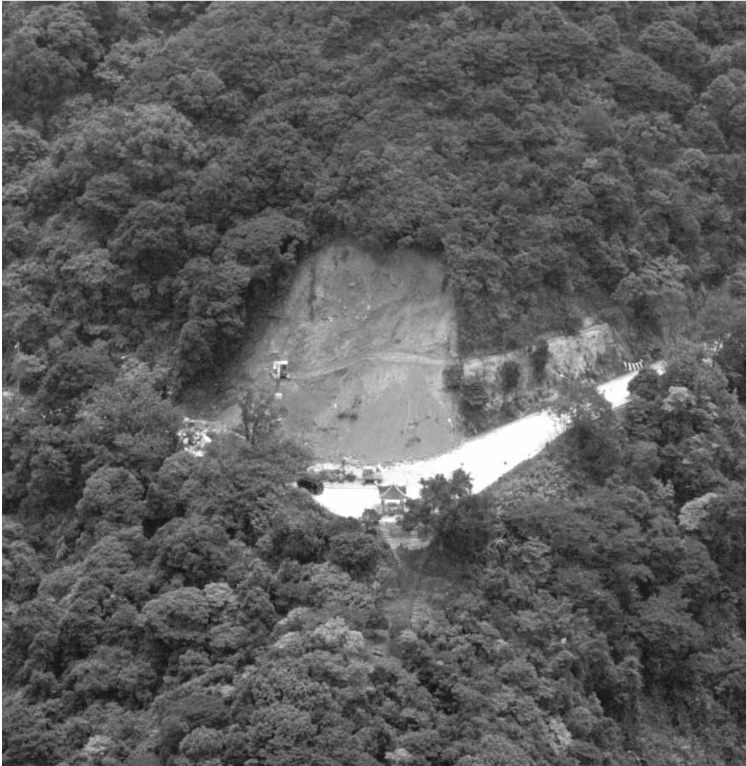
Plate 1 – Oblique Aerial View of the Landslide Site (Photograph Taken on 1 September 1999)
