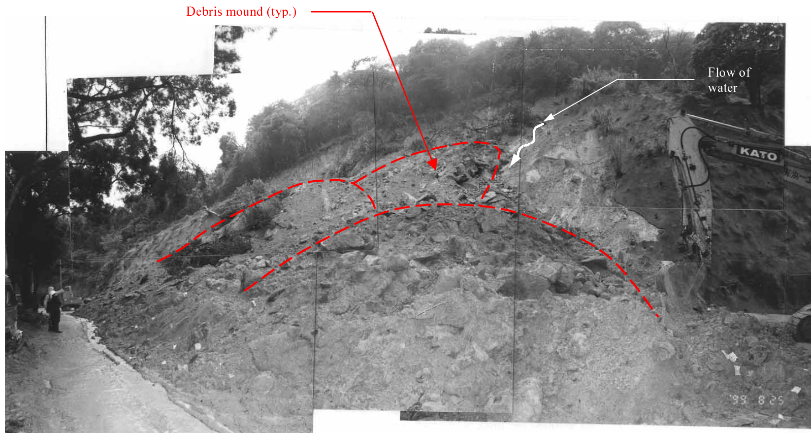
Plate 7 – General View South-East towards Landslide Scar. Note Form of Debris as a Number of Semi-Discrete Mounds (Indicated). Flow of Water Into Scar at Location Indicated. South Lantau Road Footpath Has Been Cleared of Debris (Photograph Taken on 25 August 1999)
