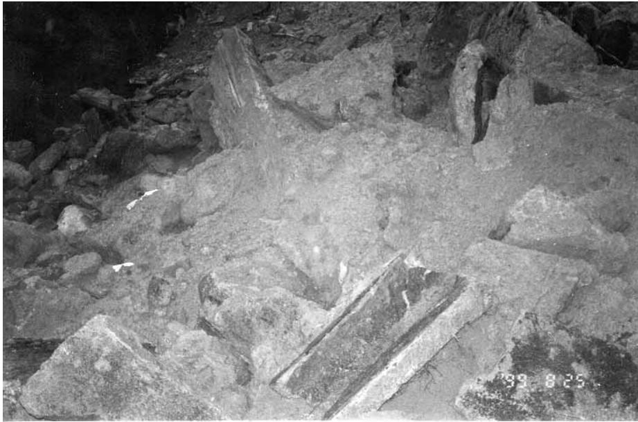
Plate 13 - Close-up of Debris at Eastern End of Mound Showing Broken Sections of U-Channel and Hard Surfacing (Photograph Taken on 25 August 1999)
