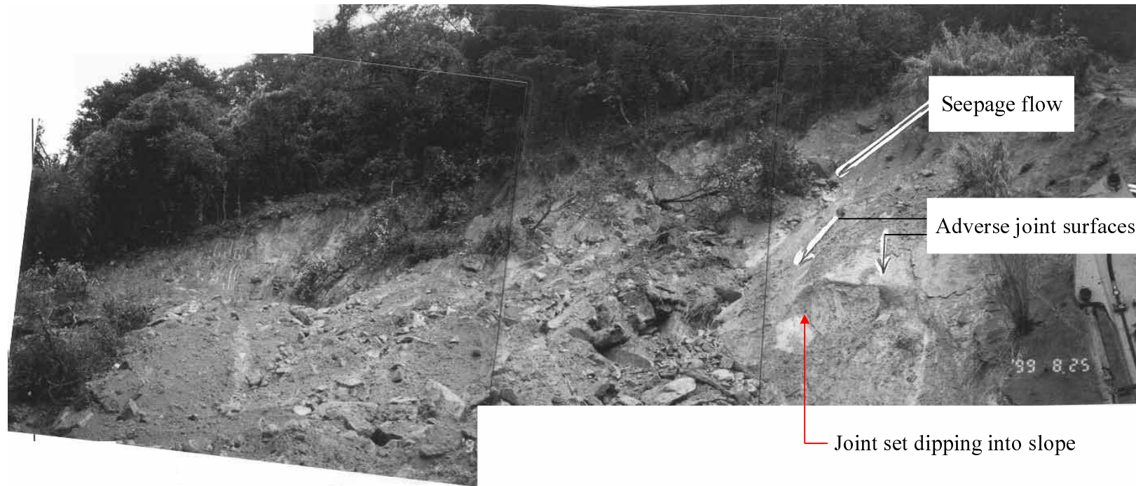
Plate 11 – View South-East towards Upper Portion of Landslide Scar and Main Scarp. Note Adverse Joint Surfaces on Corestone Exposed beneath Shotcrete on Right of Frame. Note also Joint Set Dipping into Slope Face Providing Release Plane. Flow of Water into Scar at Location Indicated (Photograph Taken on 25 August 1999)
