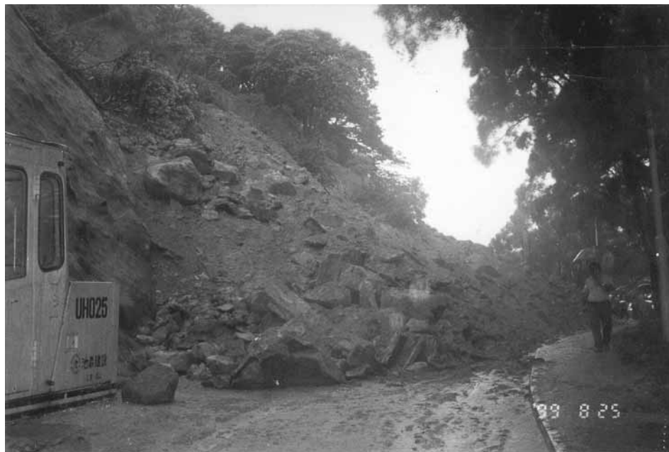
Plate 6 - View West along South Lantau Road. Debris Reposed at Approximately 20^{\circ} to 25^{\circ} (Photograph Taken on 25 August 1999)
