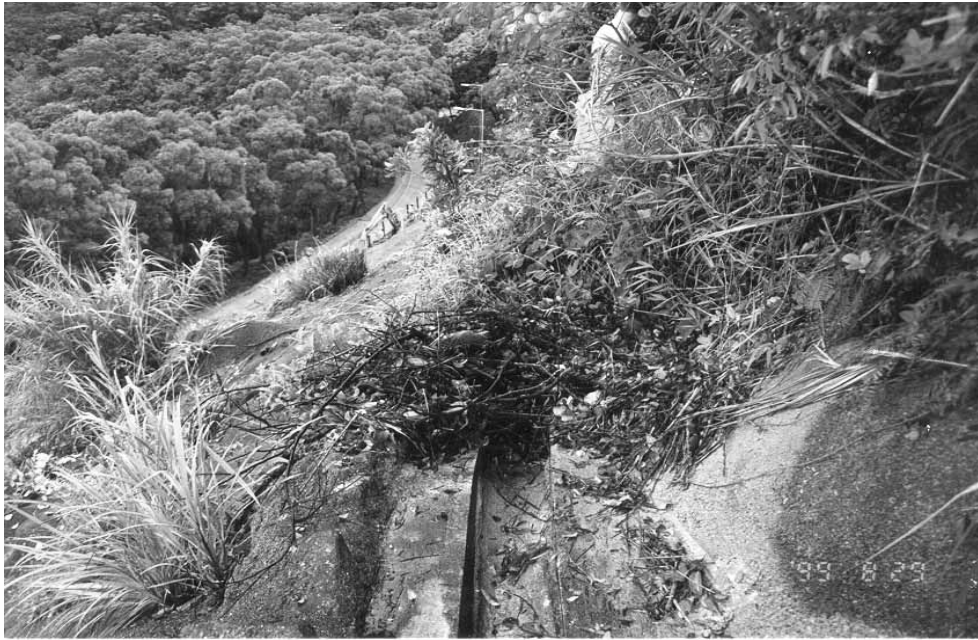
Plate 22 - Vegetation Blocking Crest U-Channel beyond Western Flank of Scar. Fall of Channel is away from Camera (Photograph Taken on 29 August 1999)
