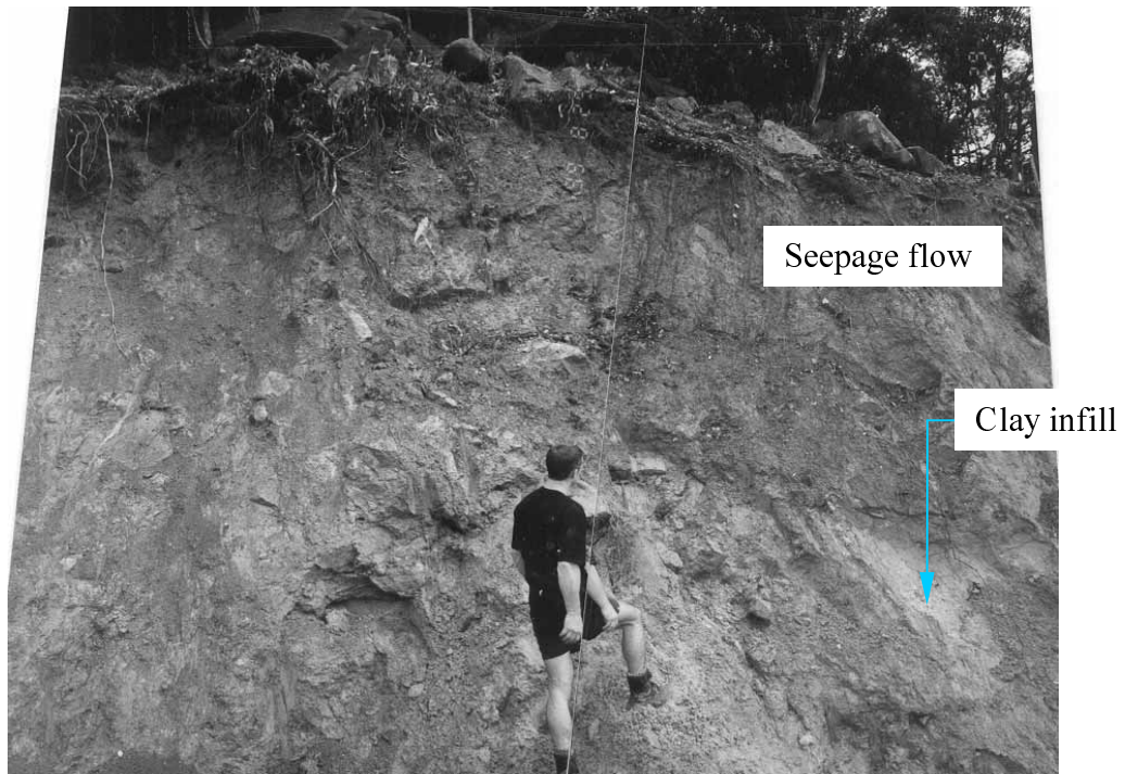
Plate 14 - View of Central Portion of Main Scarp. Seepage at Location Indicated. Clay Infilled Joint Visible on Right of Frame (Photograph Taken on 29 August 1999)
