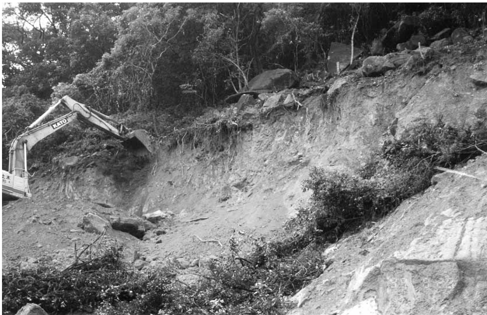
Plate 25 - View of Trimming Works in Eastern Portion of Scar. Note Large Number of Boulders Exposed on Hillside above (Photograph Taken on 29 August 1999)
