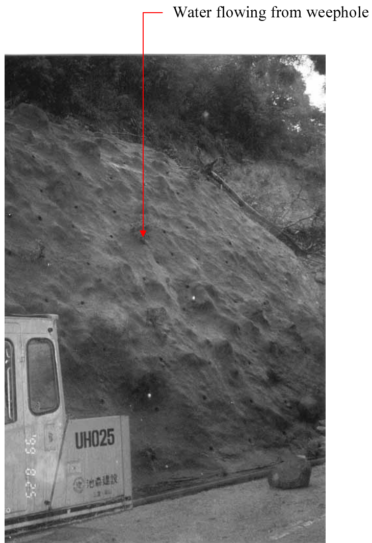
Plate 10 - Intact Portion of Shotcreted Slope beyond Eastern Flank of Scar. Note Muddy Water Flowing from Weephole (Indicated) (Photograph Taken on 25 August 1999)
