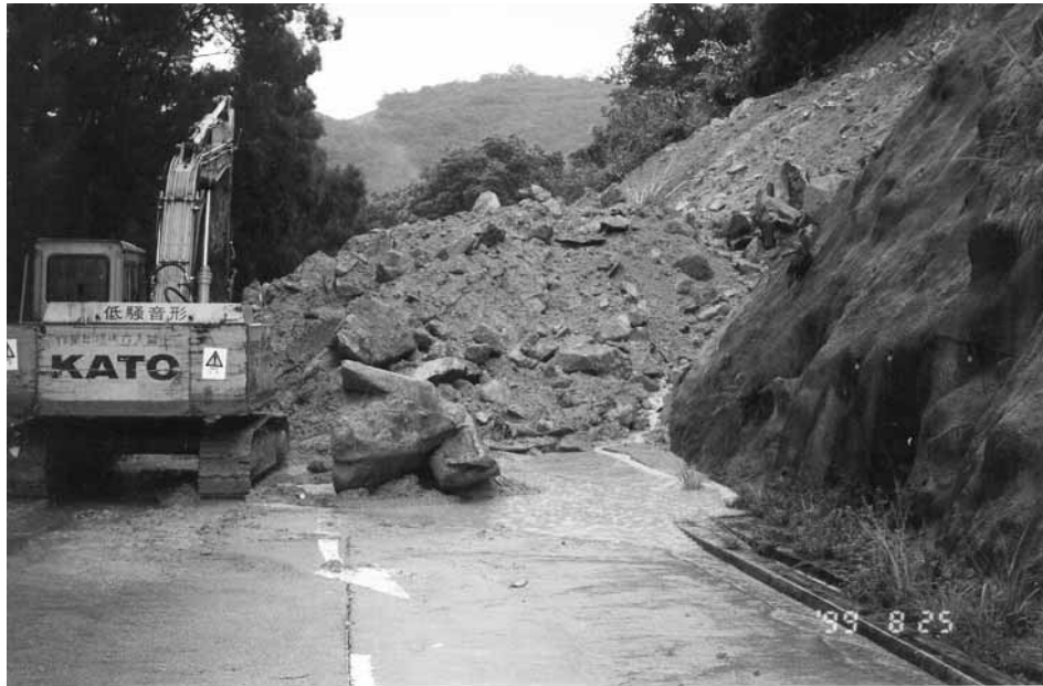
Plate 5 - View East along South Lantau Road towards Debris Mound. Note Boulder and Cobble Content of Debris and Angle of Repose ( 20^{\circ} to 25^{\circ} ) (Photograph Taken on 25 August 1999)
