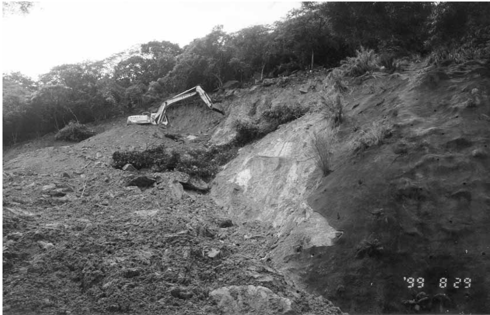
Plate 24 - View South-East along Western Flank of Scar. Adverse Joint Orientations Coincident with Previous Scar Visible in Centre-Right of Frame (Photograph Taken on 29 August 1999)
