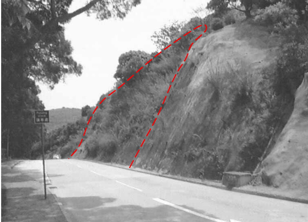
Plate 3 - View South-East across Western Portion of Slope No. 10SW-C/C20 on 26 April 1995. 1999 Landslide Site Indicated. Note Vegetation Growing through Hard Surfacing (Photograph Taken by FMR Consultant)
