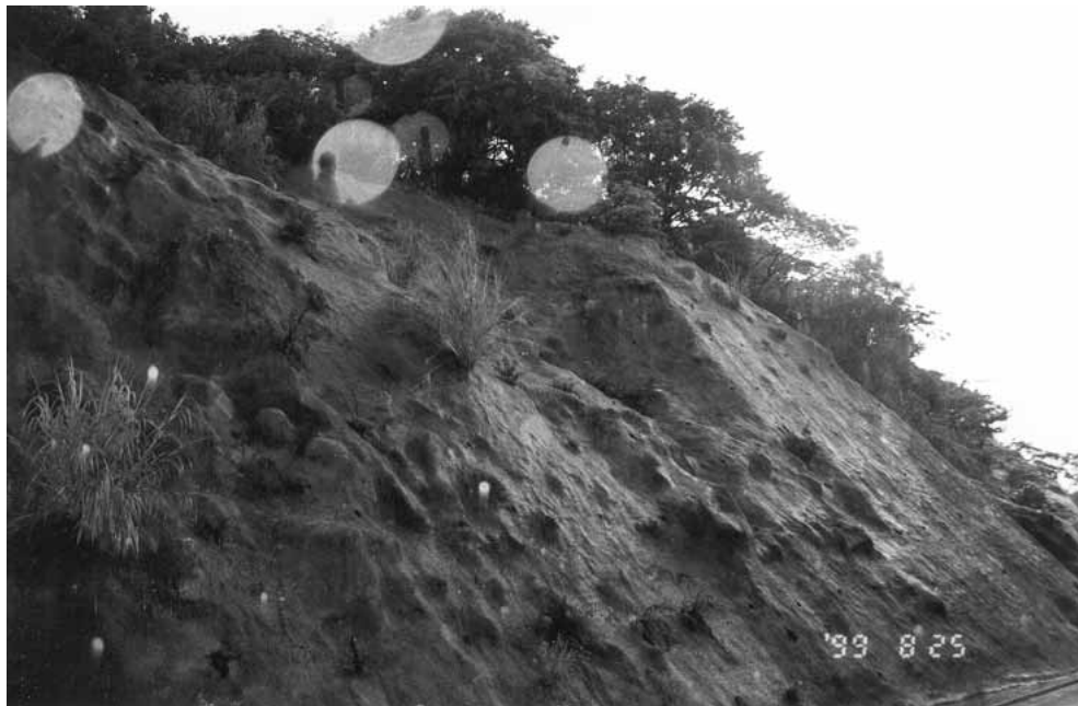
Plate 23 - View South-West towards Pre-Existing Wedge-Shaped Landslide Scar in Slope West of Present Failure. Note also Boulders and Cobbles Visible in Shotcreted Slope Face (Photograph Taken on 25 August 1999)
