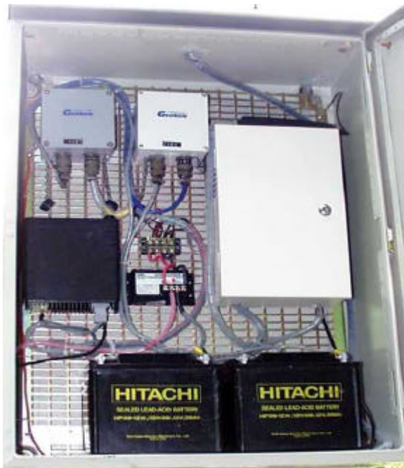
Plate C3 - Details of the Po Shan Mansion Site Subscriber Unit
