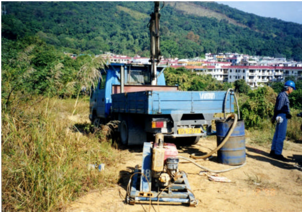
Plate 2 - Diesel Water Pump and Service Water Barrel to Support Drilling Operation
