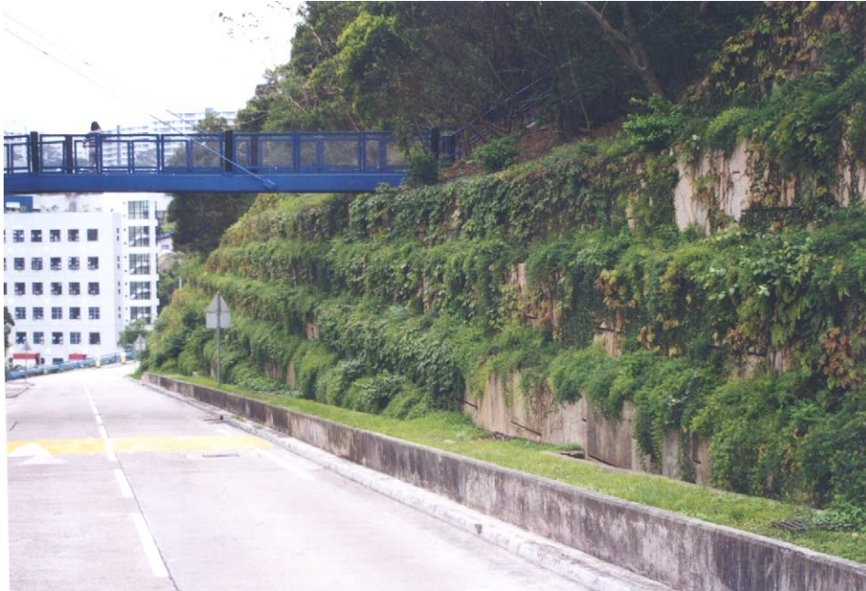
(a) The creative use of a series of small terrace reduces the apparent size and scale of the slope and allows introduction of valuable greenery into the surrounding landscape
