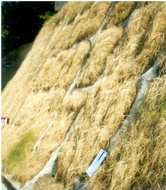
(k) Recently completed slope using “Creat” and General Toyo-Mulching
