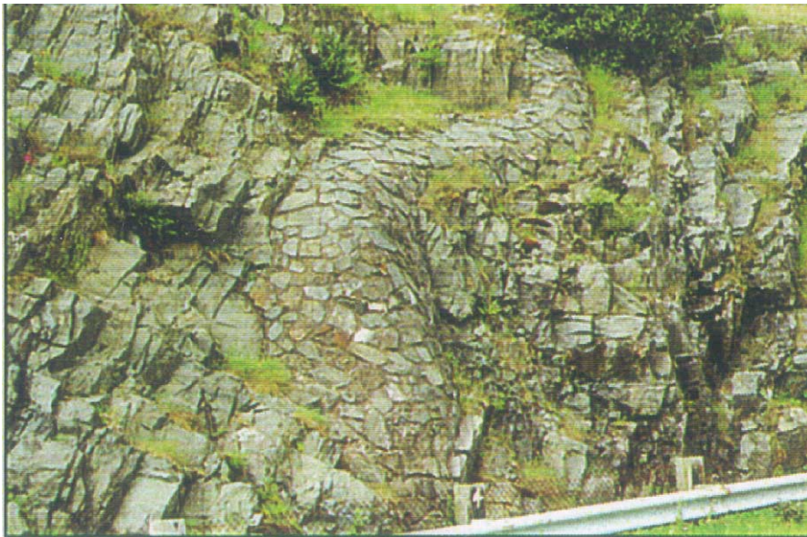
(b) Good practice. Concrete within the outcrops has been clad in local stone. M6 Motorway UK
