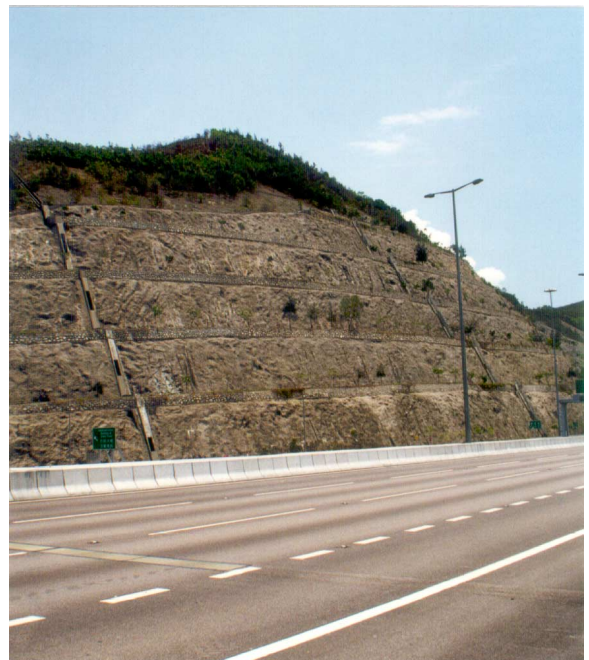
(p) Berm planters on rock slope
