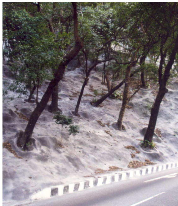
(aa) Tree rings on hard surfaced slope
