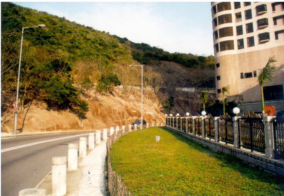
(h) Natural profiles under the pale brown sprayed shotcrete create a pattern which reduces the monotone effect of a single colour.
