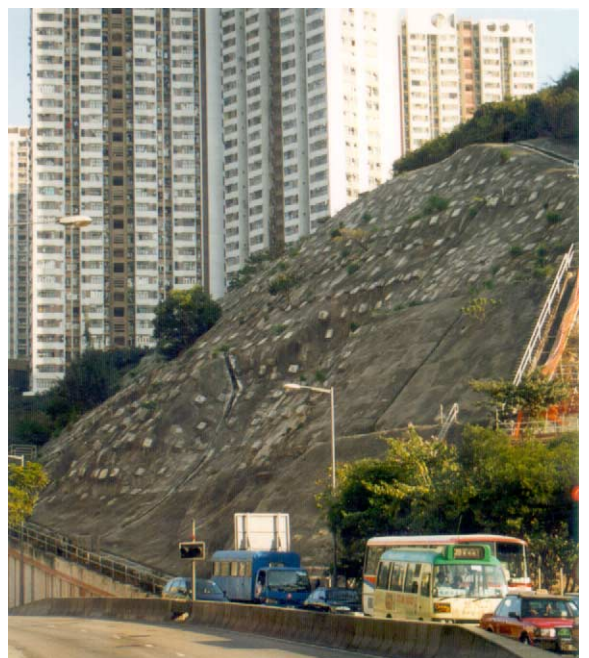
(l) Countersunk nail head detail on a hard surfaced slope
