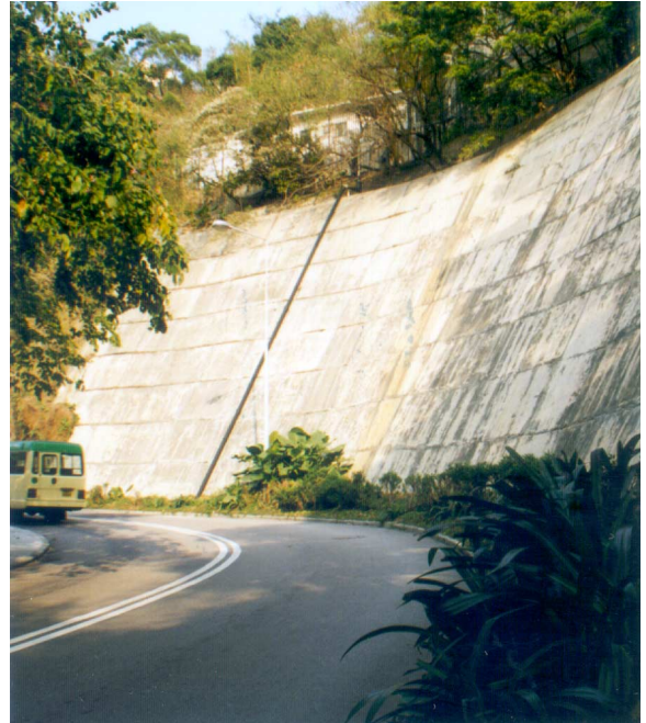
(j) Large-scale block pattern surface cladding
