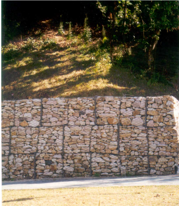
(m) Layered rock infill pattern in gabion basket
