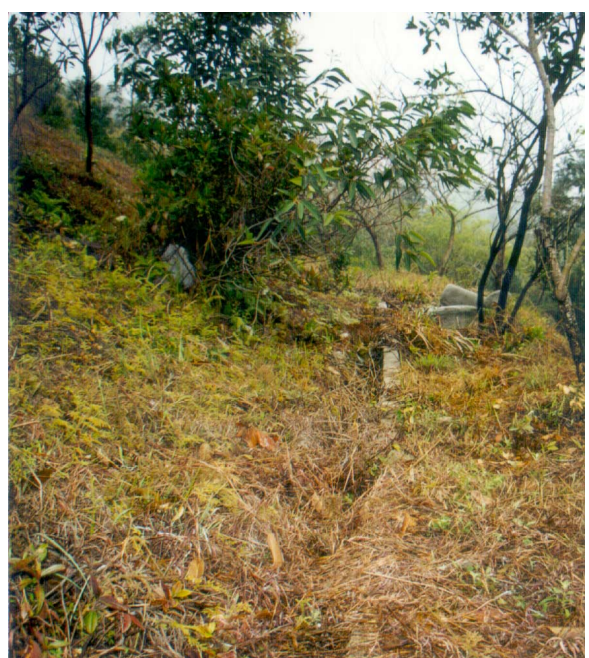
(d) Blockage of drainage channel by uncontrolled grass growth
