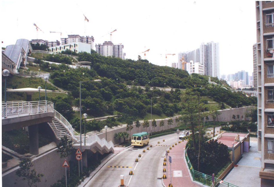
(a) Planting at the toe, top of retaining wall and soil slopes above successfully create a unified appearance for the whole slope and help to blend it into the surrounding landscape
