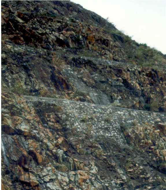
(i) Masonry block used as infill on rock slope
