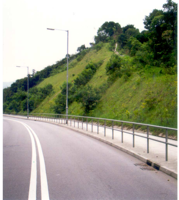
(b) Hydroseeding with grass and mixed tree planting on 40° soil cut slope
