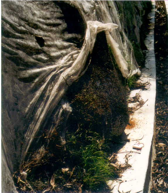
(a) Accumulation of eroded soil behind erosion control mat
