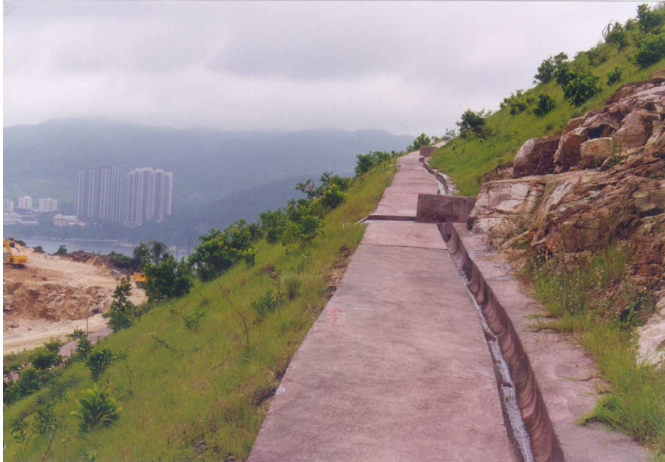
(a) Use of pigments to tone with adjacent rock features helps to integrate the drainage infrastructure
