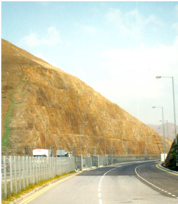
(c) Sprayed concrete with naturalistic colouring and patterning
