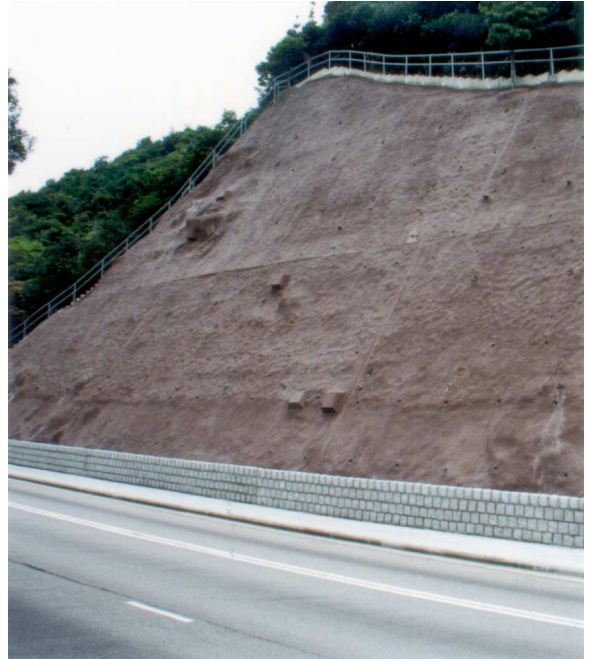
(b) Sprayed concrete with colour pigment
