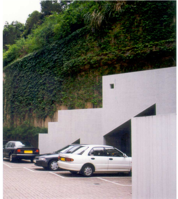
(r) Hanging planter on medium-height retaining wall (right upper side)
