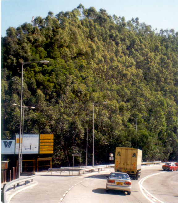
(e) Mature hydroseeded grass and tree seed on 50° soil cut slope
