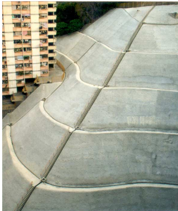
(b) Bad practice - this slope has almost no features dividing it up resulting in a scale out of proportion with its setting
