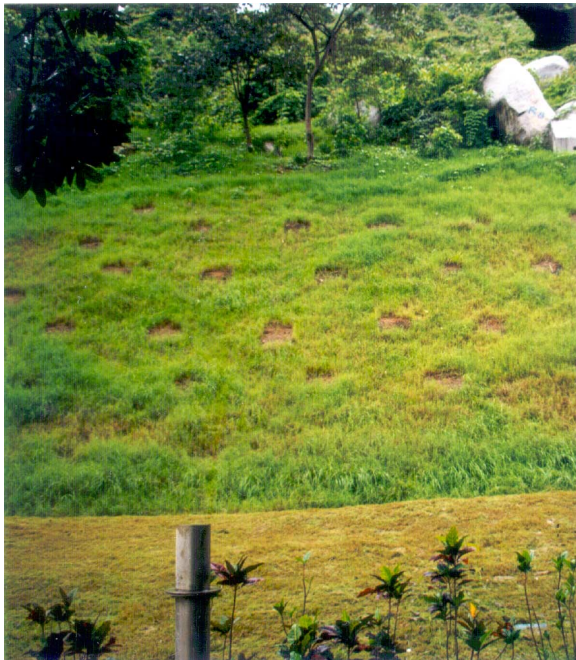
(g) Soil nail heads exposed beneath recently hydroseeded 45° cut slope
