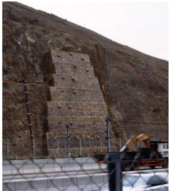
(t) Buttress is coloured to suit landscape and has been given a random stonework finish.
