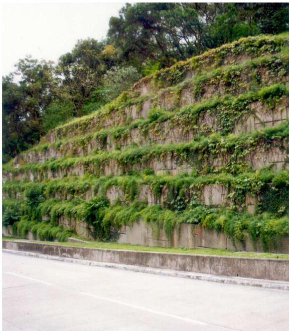
(o) Stepped-back reinforced fill structure with facing panels
