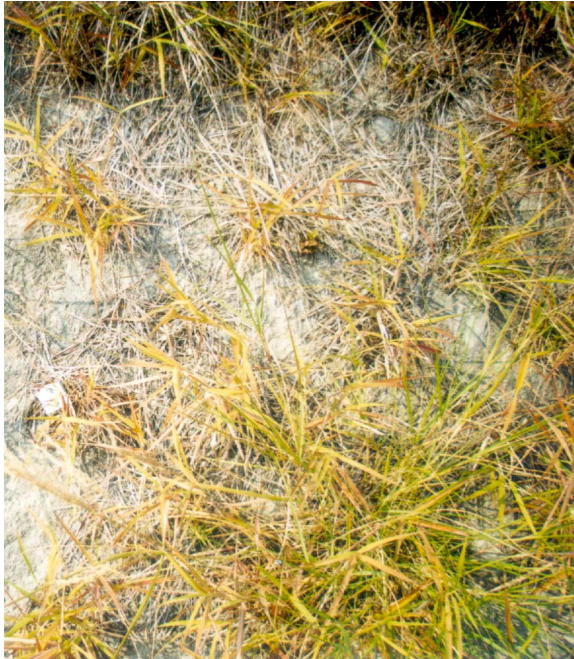
(i) Close-up view of “Grasscrete” surface layer
