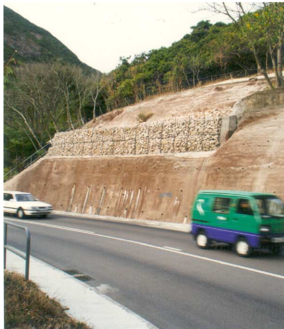
(b) Bad practice - the juxtaposition of materials of different visual characteristics in this case shotcrete and gabions
