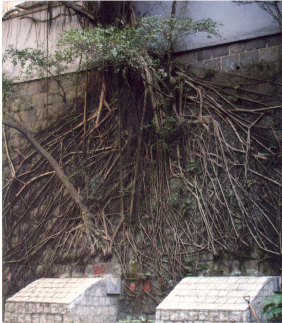
(y) Toe buttress upgrading works preserving wall trees
