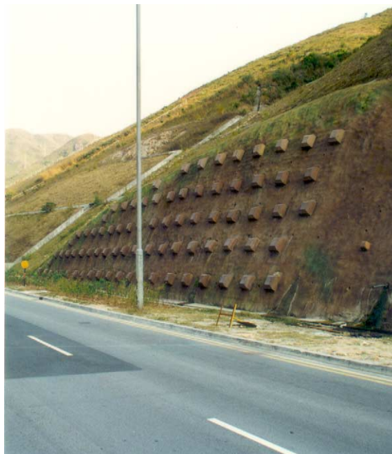
(u) Geometric pattern of anchorage heads gives a reasonable visual appearance
