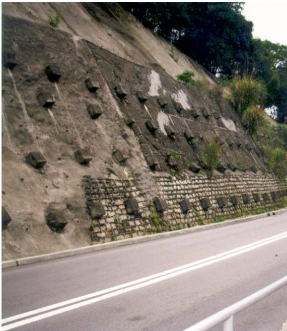
(k) Raised nail head detail on a hard surfaced slope
