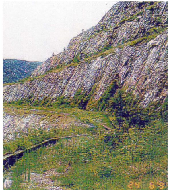
(v) Lam Tei Quarry - An attempt to "green" Lam Tei Quarry by planting of berms between rock slopes with tree whips, shrubs and climbers.
