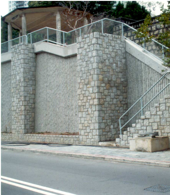
(o) Co-ordinated materials and textures on a retaining wall
