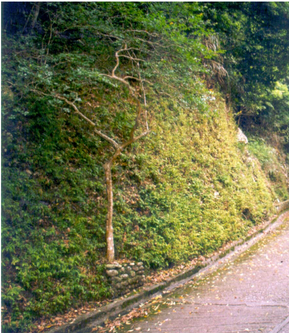
(c) Self-seeded grasses and groundcover plants on 70° soil cut slope
