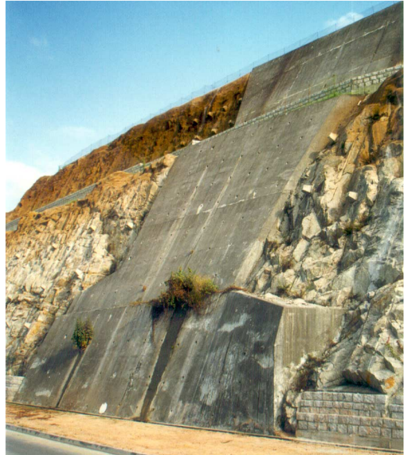
(r) Visually intrusive rock buttress contrasts with the texture and scale of the slope
