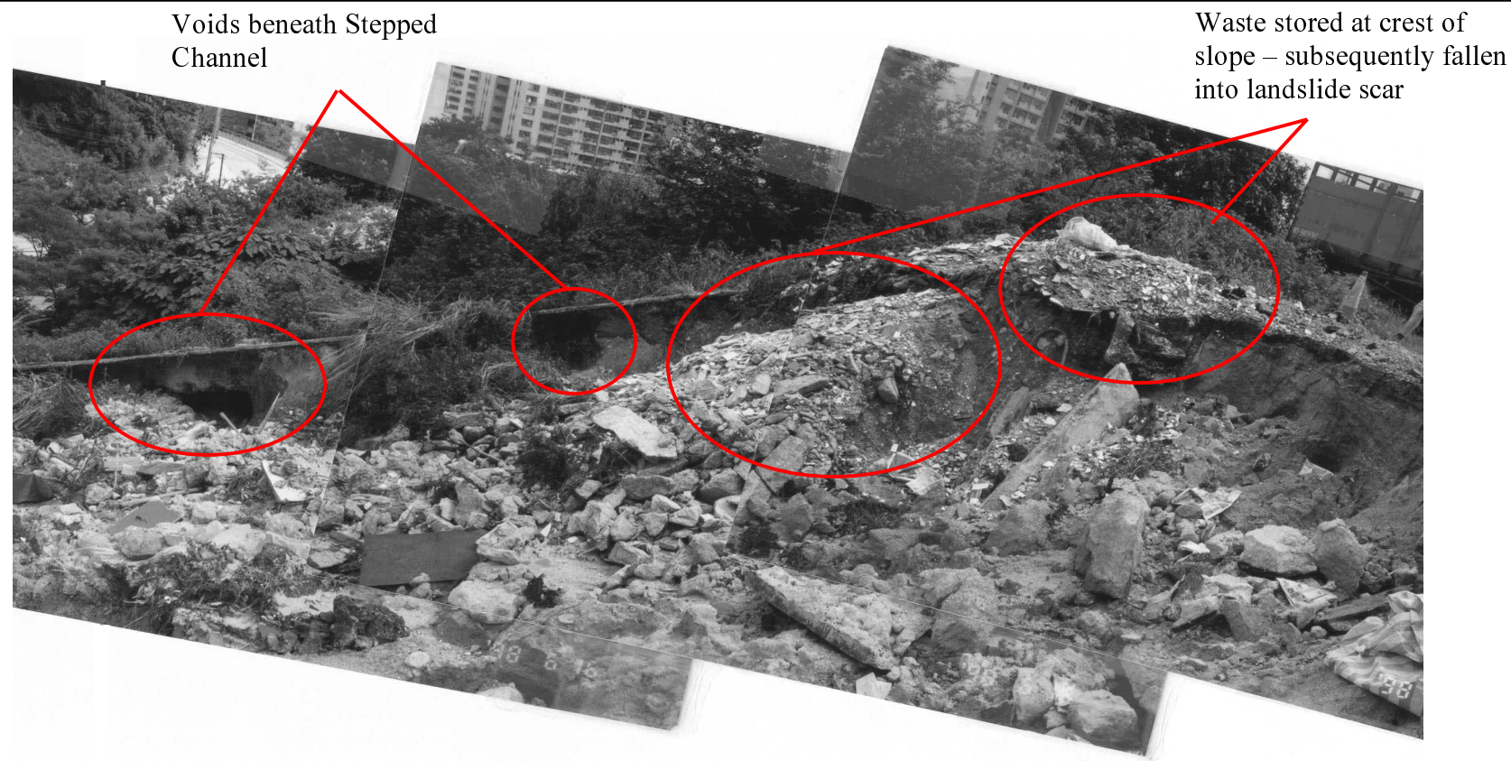
Plate 12 – General View looking across and down the Landslide Scar. Undermining of the Stepped Channel clearly evident. Note the Nature of the Material within the Landslide Scar – Heterogeneous Construction Waste and a Fill Capping. Layering of Capping clearly evident. Construction Waste also appears to have been stored at the Crest of the Slope adjacent to the Stepped Channel. Some of this Waste appears to have subsequently fallen into the Landslide Scar (Photographs taken on 16 June 1998)
