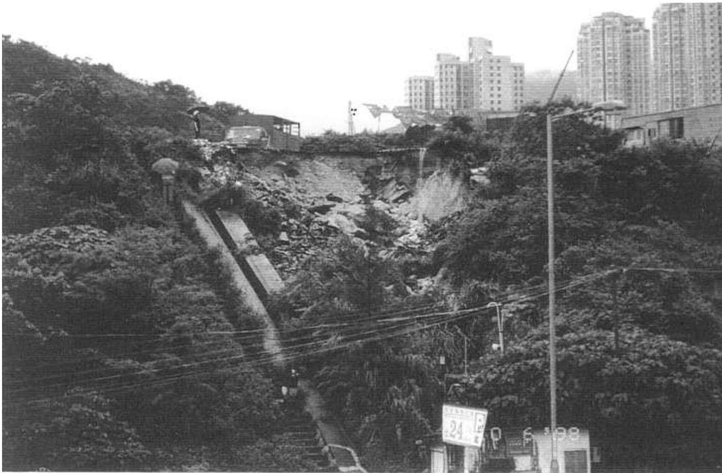
Plate 2 – View of Landslide Scar. Note Water still Discharging into Landslide Scar (Photograph taken on 10 June 1998)
