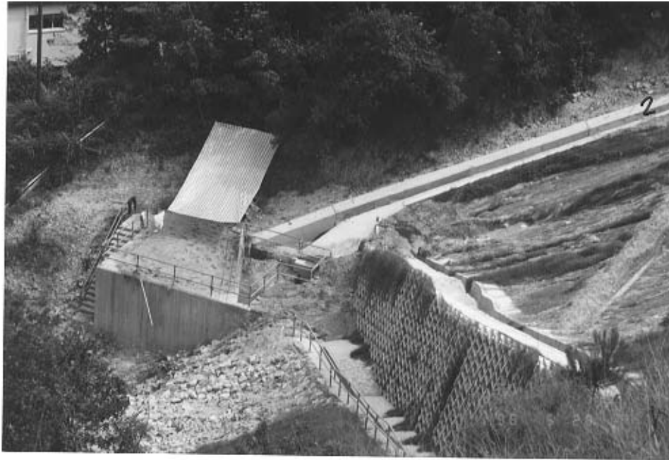
Plate 20 – Event No. 2: 24 May 1998. View South Towards Toe of Slope A Indicating Debris Deposition on Slope Face, with Over-spill onto Concrete Apron at Toe of Crib Wall and Reservoir Structure. (Photograph Taken on 28 May 1998)
