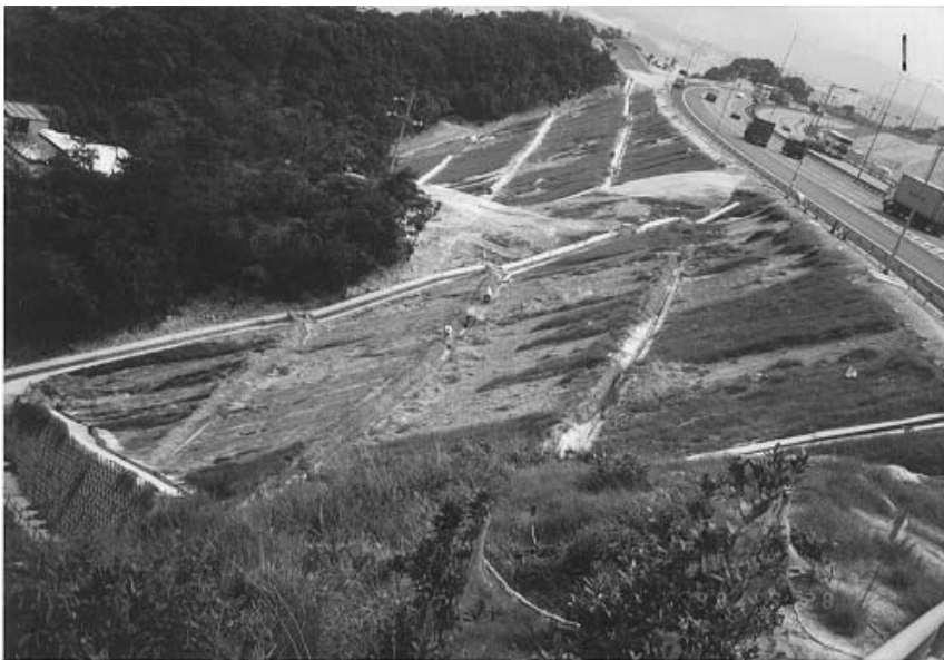
Plate 19 – Event No. 2: 24 May 1998. View South-West Across Slope A and Slope B, Indicating Extensive Failure in Upper Two Batters of Slope A, with Runout of Debris and Additional Failures on Third and Fourth Batters (Below 64.5 mPD and 58 mPD Berms, Respectively). Clearance of Berm Drainage Channels Underway. Note Stockpiling of Debris on Berm Aprons. Note Also Little Change to Appearance of Slope B Since 8 May 1998 (Refer Plate 15). (Photograph Taken on 28 May 1998)
