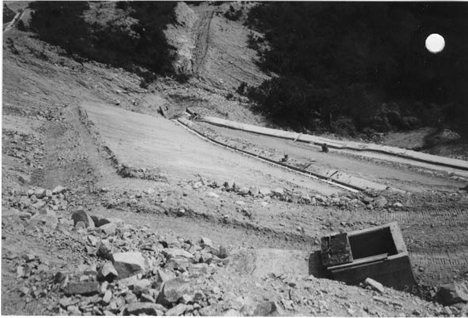
Plate 55 – View North-East Across Slope A From 64.50 mPD Berm Indicating Placement of DG Fill Over Rock Fill on Batter Between 64.50 mPD and 58 mPD, and Landscaping Fill on Batter Between 58 mPD and Crest of Crib Wall. (Photograph taken on 26 November 1997)
