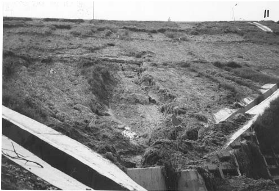
Plate 20 – Event No. 2: 24 May 1998. View South Towards Toe of Slope A Indicating Debris Deposition on Slope Face, with Over-spill onto Concrete Apron at Toe of Crib Wall and Reservoir Structure. (Photograph Taken on 28 May 1998)
