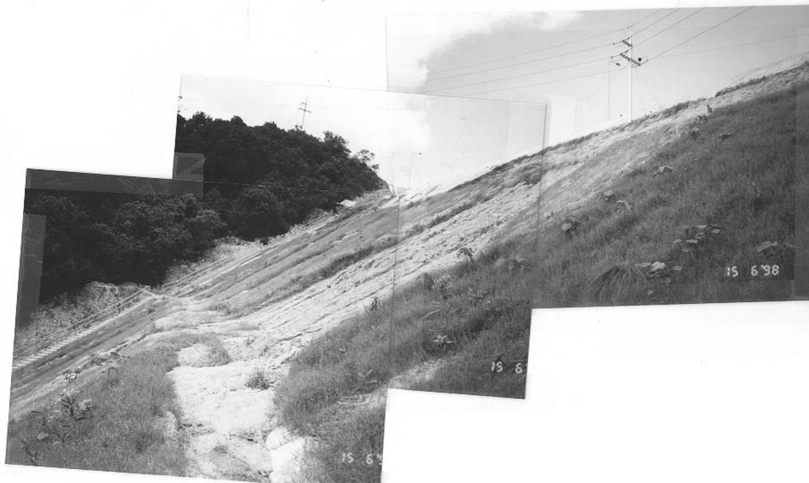
Plate 25 – Event No. 3: 9 June 1998. View South-West Along 45 mPD Berm on Slope B Indicating New Failures in Slope B Affecting Batter Above 52.5 mPD Berm (Right of Frame). Note Debris Over-Spill onto Batter Below 45 mPD Berm and Blockage of Berm Drainage. (Photograph Taken on 15 June 1998)
