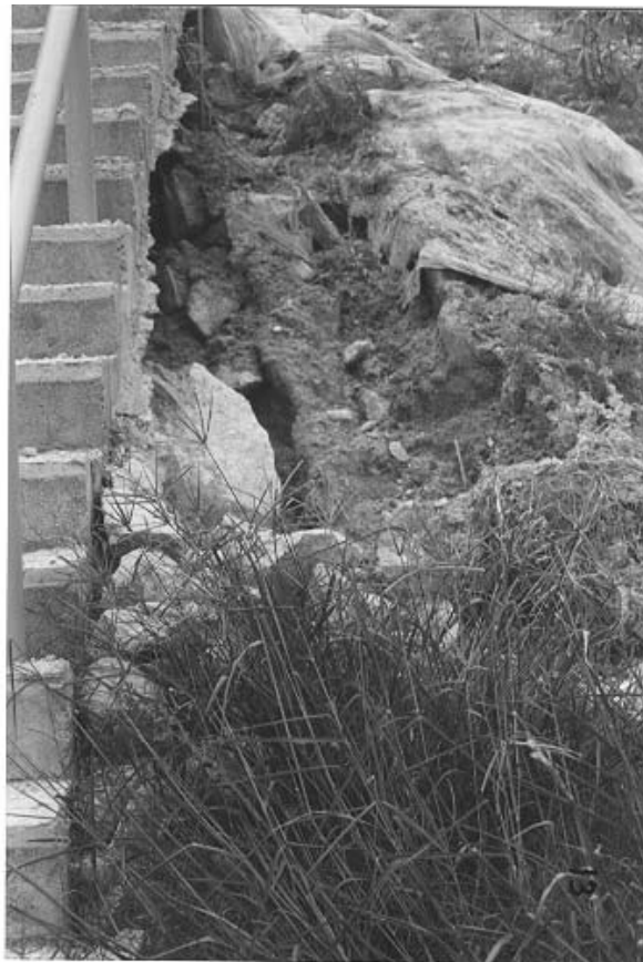
Plate 23 – Event No. 2: 24 May 1998. Close-up of Access stairway Below Crib Wall Indicating Washout of Fill Material and Undermining of Stairs. (Photograph Taken on 28 May 1998)
