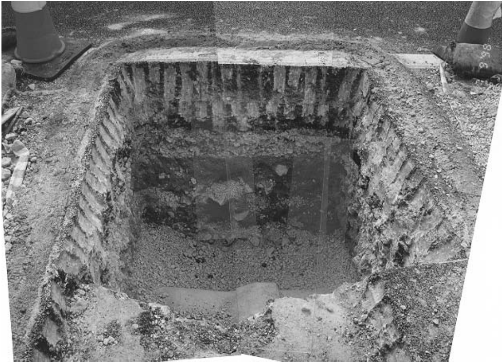
Plate 38 – Trial Pit ATP1 Excavation at Crest of Slope A. Note Line of Cracking Across Far Side of Pit Indicated by Yellow Foam on Either Side. Pavement Layers and Stormwater Drain Exposed in Pit. (Photograph Taken on 9 July 1998).
