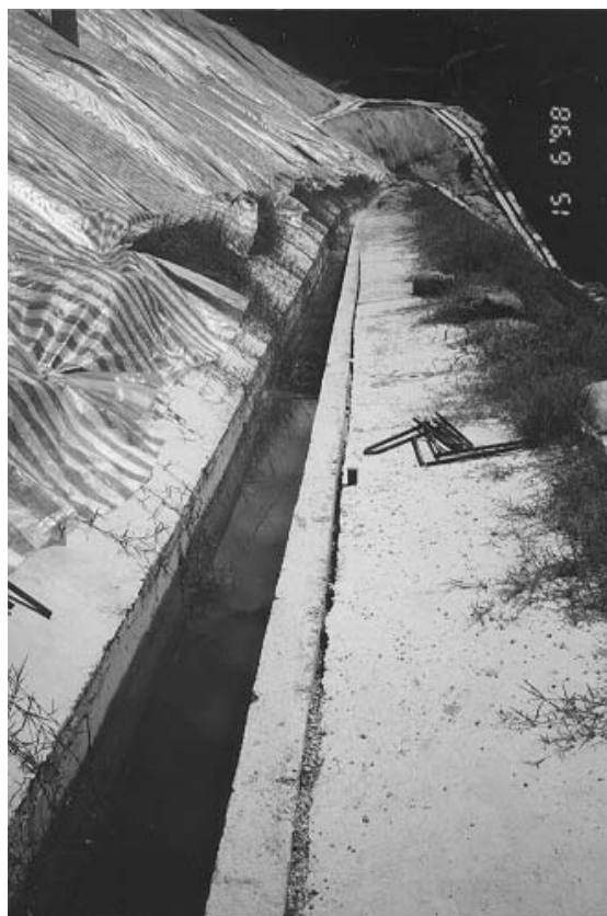
Plate 35 – Event No. 3: 9 June 1998. View North-East Along 60 mPD Berm on Slope B Indicating Separation of Berm Apron Slab from Berm U-Channel. Also Note Standing Water in U-Channel. (Photograph Taken on 15 June 1998)
