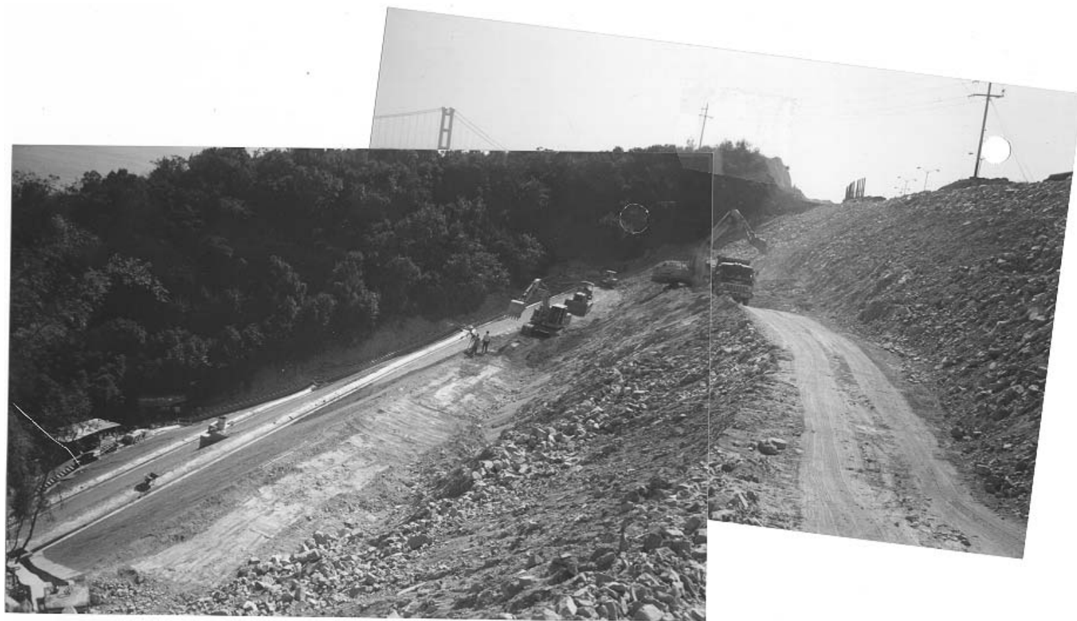
Plate 52 – View South Across Slope B indicating Placement of Landscaping Fill Over DG Layer Between 52.5 mPD and 45 mPD. Note Finished Slope Face Now Flush With Drainage Channel Above 45 mPD Berm. (Photograph Taken on 5 November 1997)
