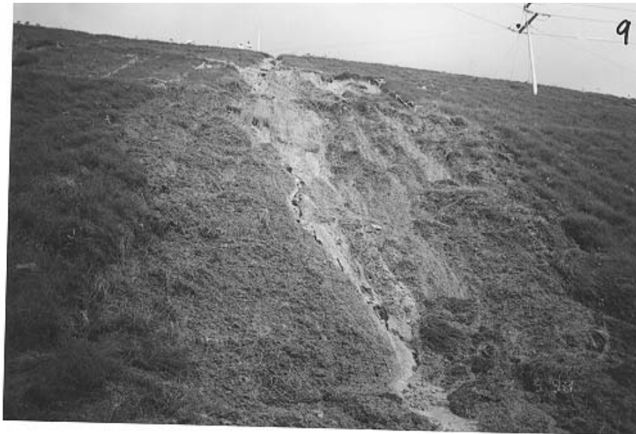
Plate 13 – Event No. 1: 4 May 1998. View North-West Towards Crest of Slope B from 45 mPD Berm up Succession of Landslide Scars Below Road Drainage Outlet Above 67.5 mPD Berm at CH 1000 Note Washout of Scars and Accumulation of Debris on Batter Above 45 mPD Berm in Foreground. (Photograph Taken on 4 May 1998)
