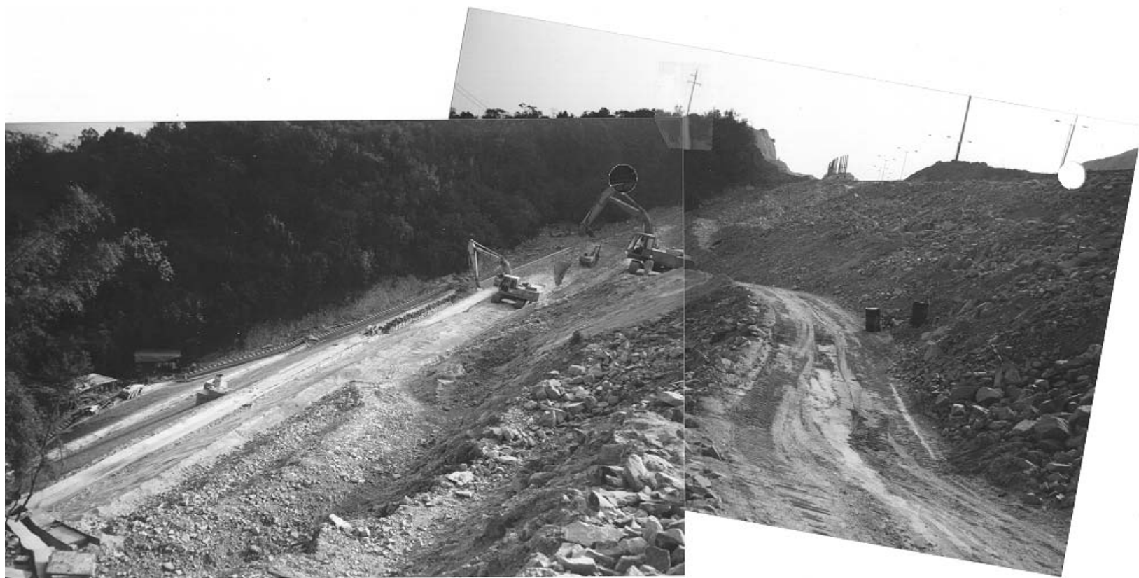
Plate 50 – View South Across Slope B Construction. Note Placement and Compaction of DG Fill Over Rock Fill in Centre of Frame on Batter Between 52.5 mPD and 45 mPD Berms (Small Roller Visible Behind Lower of two Large Excavators). Note Also Drainage Works in Progress Below Filling Operations, Upstand Remaining on Channel Structure on Left of Frame to Receive Landscaping Fill Layer and Planar Face on DG Fill. (Photograph Taken on 29 October 1997)
