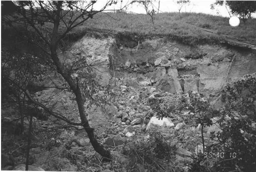
Plate 4 – View North-West Across Landslide Scar Towards Main Scarp. Horizontal Layering Visible in Exposed Fill. (Photograph Taken on 10 October 1995)
