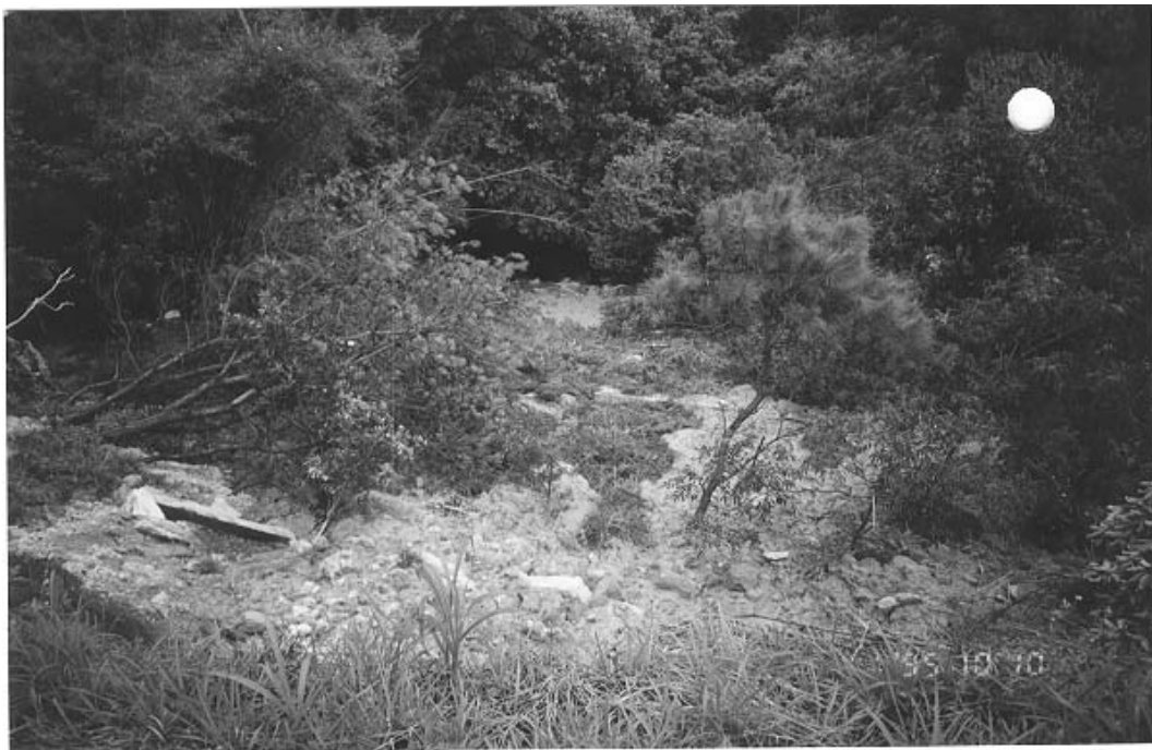
Plate 3 – View South-East Over Landslide Scar Indicating Debris Runout. Concrete Structure Visible in Debris on Left. Reservoir Filled With Debris Visible in Centre Background. (Photograph Taken on 10 October 1995)
