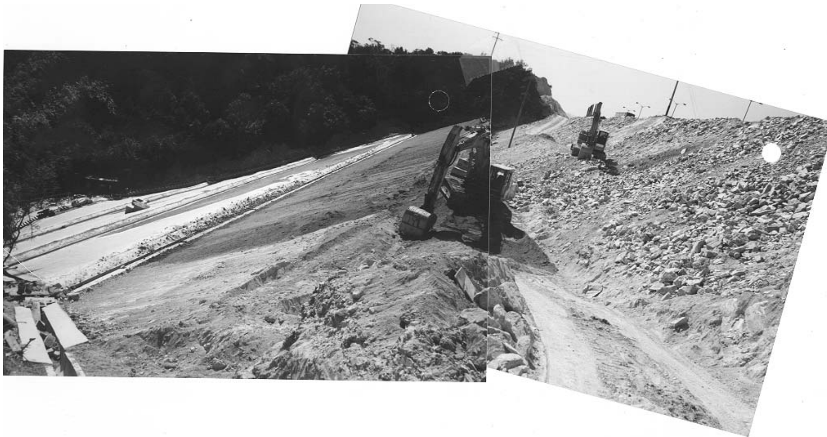
Plate 54 – View South Across Slope B Indicating Placement of Landscaping Fill Over DG Fill Between 60 mPD and 52.5 mPD. Note ‘Loose-Tipping’ Approach and Impressions on Upper Half of Slope Face Suggesting Tamping by The Backhole Bucket. (Photograph Taken on 9 November 1997)
