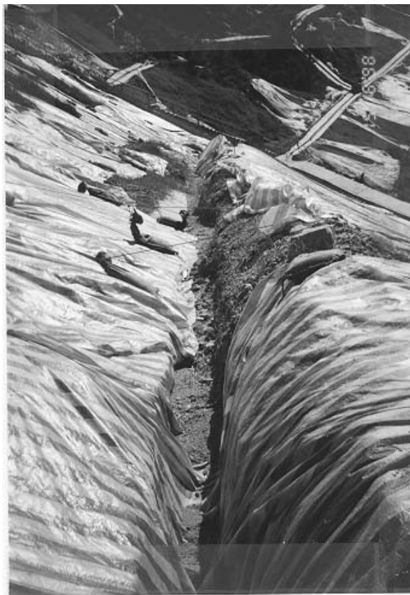
Plate 31 – Event No. 3: 9 June 1998. View North-East Along 64.5 mPD Berm on Slope A Indicating Debris Previously Stockpiled on Berms Washed into Surface Drainage. (Photograph Taken on 15 June 1998)
