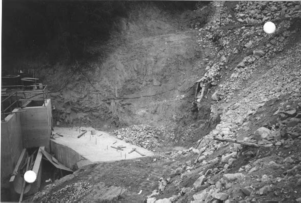
Plate 40 – View South-West from Toe of Slope No. 6SE-C/FR13. New Reservoir Structure on Left of Frame. Crib Wall Footing Adjacent to Reservoir Insitu Profile Exposed Beneath Previous Fill and Rockfill. (Photograph Taken on 7 April 1997)
