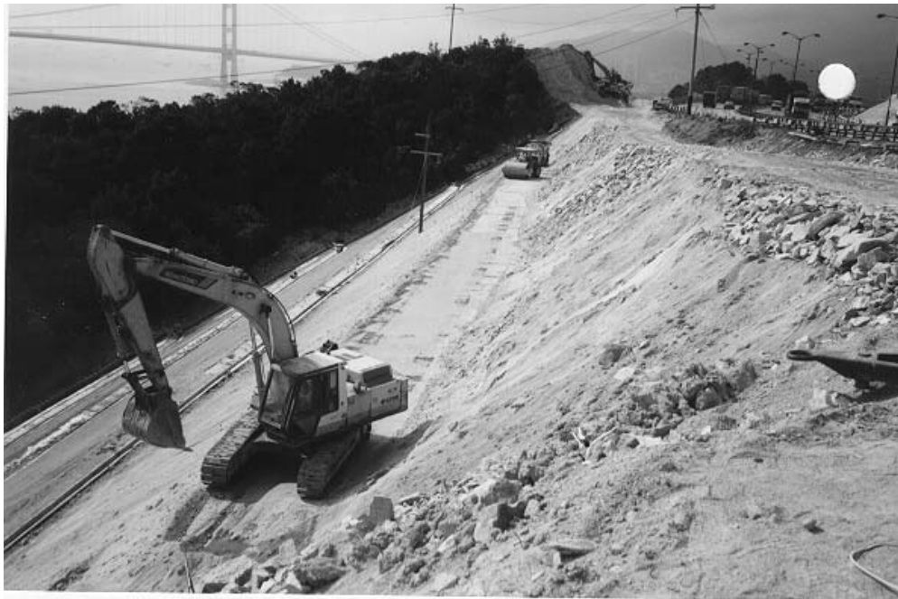
Plate 56 – View South Across Slope B Indicating Placement of DG Fill Over Rock Fill on Batter Between 67.5 mPD and 60 mPD. Note Planar Face to DG Fill and Apparently Minor Trimming of Slope Face Following Compaction. (Photograph Taken on 26 November 1997)
