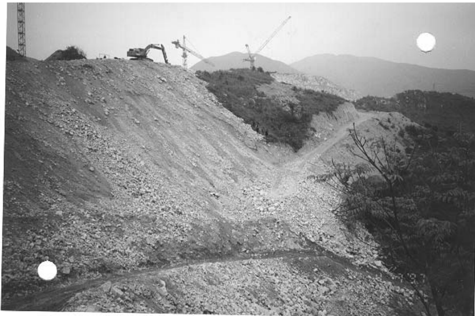
Plate 41 – View North-East Across Upper Portion of Slope No. 6SE-C/FR13 Indicating Haul Road in Natural Slope to North-East and Rock Fill Material (This Rock Fill Apparently Did Not Meet Specification Due to High Fines Content). (Photograph Taken on 7 April 1997)
