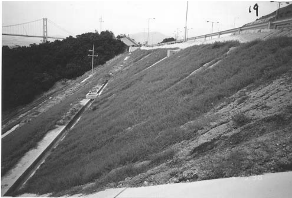
Plate 7 – Event No. 1: 4 May 1998. View South-West Along Upper Batter of Slope B and 67.5 mPD Berm from Northern End. Note Road Drainage Discharge into Slope Drainage in Middle-Ground and Debris from Landslides Blocking Berm Drainage Channel on Either Side of Catchpit. (Photograph taken on 4 May 1998)
