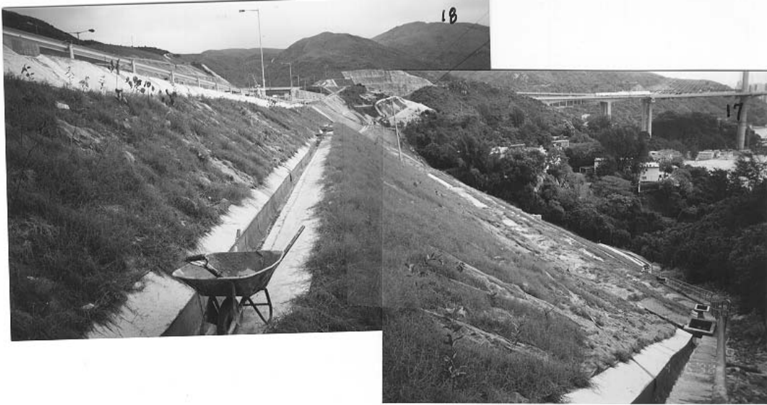
Plate 6 – Event No. 1: 4 May 1998. View North-East Along 67.5 mPD (Uppermost) Berm of Slope B and Lower Batters from Southern End of Slope. Note Extensive Blockage of 67.5 mPD Berm Drainage and Failed Areas of Slope on Right of Frame. (Photograph Taken on 4 May 1995)
