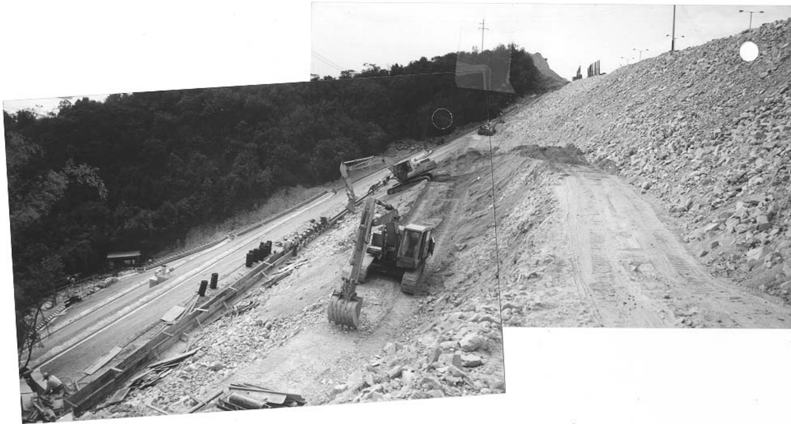
Plate 53 – View South Across Slope B Indicating Placement of DG Fill Over Rock Fill on Batter Between 60 mPD and 52.5 mPD. Note Shallow Depth of DG Fill, Apparently Minimal Benching in Rock Fill and Compaction of Fill by Vibrating Plate Compactor on Slope Face (Beneath Arm of Far Excavator) to Produce Planar Face. (Photograph Taken on 12 November 1997)
