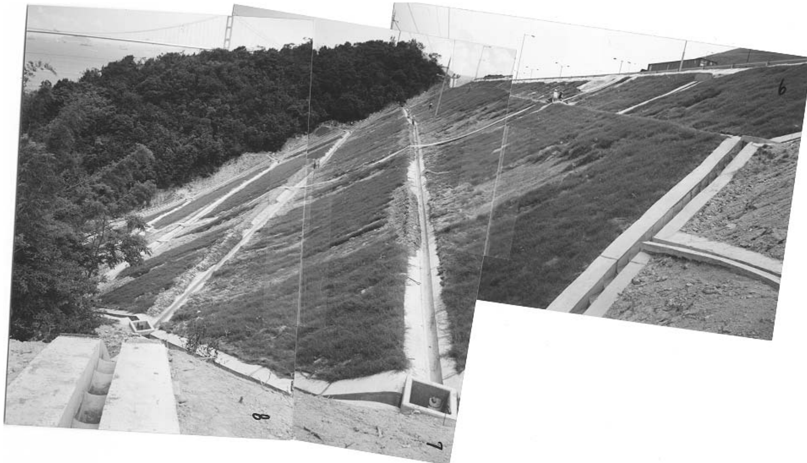
Plate 15 – Event No. 1: 4 May 1998. View South-West Across Slope B from Natural Spur Separating Slopes A and B. 60 mPD Berm in Centre of Frame. Note Extent of Scars in Slope Face. Note also Clearance of Berm Channels and Stock piling of Debris on Berm Apron. (Photographs Taken on 8 May 1998)
