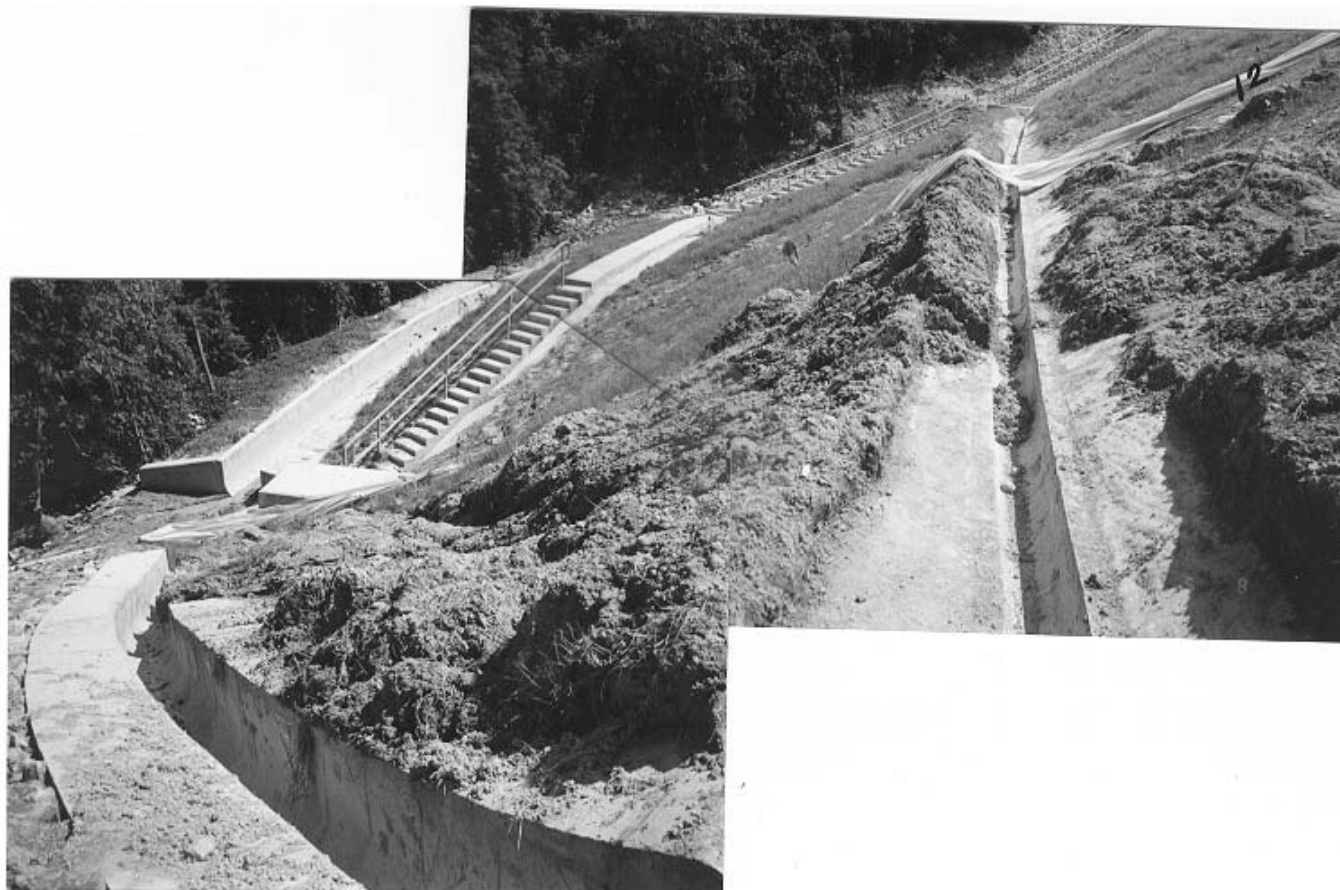
Plate 17 - Event No. 1: 4 May 1998. View South-West Along 37.5 mPD Berm Towards South End of Slope B Indicating Debris Deposition on Slope Face. Clearance of Berm Drainage in Progress. Note Also Apparent Runout Over Batter Below Berm in Middle Distance Indicated by Flattened Hydroseeding. Outlet for Culvert P043 Visible at Toe of Slope on Left of Frame. (Photograph Taken on 8 May 1998)
