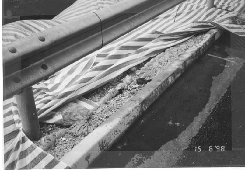
Plate 36 – Event No. 3: 9 June 1998. Close-up of Filled Cracking Behind Kerb Beam Approximately Mid-Way Along Crest of Slope A. Note Also, Separation of Kerb Beam from Pavement. (Photograph Taken on 15 June 1998)
