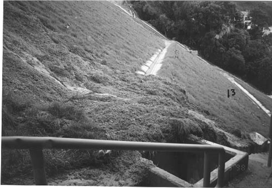
Plate 12 – Event No. 1: 4 May 1998. View North-East Along 45 mPD Berm from South End of Slope B. Accumulated Debris on Berm in Foreground. Note Also Debris on Same Berm in Distance Beyond Manhole on Slope Face, and Debris Deposition on 37.5 mPD Berm Below on Right of Frame. (Photograph Taken on 4 May 1998)
