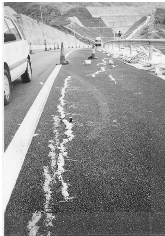
Plate 37 – Event No. 3: 9 June 1998. View North-East Along Hard Shoulder at Crest of Slope A Approximately 35 m from North End Indicating Cracking in Pavement. Cracking Filled with Expanding Foam. (Photograph Taken on 15 June 1998)
