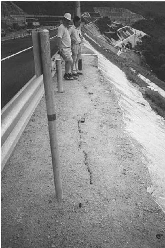
Plate 5 - Event No. 1: 4 May 1998. View North-East Along Crest of Slope B Indicating Tension Cracking South of Road Drainage Outlet on Slope (Outlet Visible on Right of Frame). (Photograph Taken on 4 May 1998)
