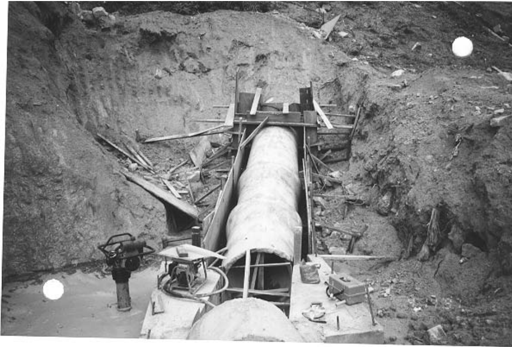
Plate 43 – View North-West from Toe of Slope No. 6SE-C/F14 Indicating New Drainage Works as Extension of Existing Culvert P043 to the Toe of Slope B. (Photograph Taken on 14 April 1998)
