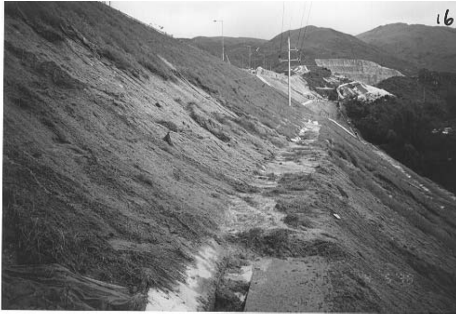
Plate 8 – Event No. 1: 4 May 1998. View North-East Along 60 mPD Berm from South End of Slope B Indicating Scar on Batter Above and Runout of Debris on Batter Below. (Photograph Taken on 4 May 1998)
