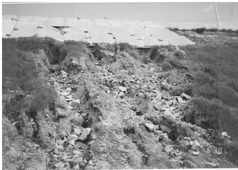
Plate 34 – Event No. 3: 9 June 1998. View Towards Crest of Slope B From 45 mPD Berm Indicating Secondary Washout of Existing Scar. Note Plastic Sheetting on Slope Above and Thin Layer of Rock Fill Exposed Beneath DG Fill, with Existing Fill Visible Behind Rock Fill. (Photograph Taken on 15 June 1998)
