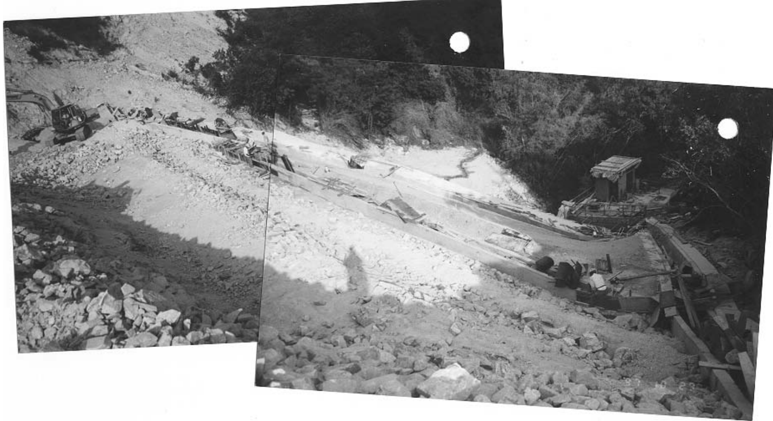
Plate 48 – View East Towards Toe of Slope A from Berm Elevation at 64.5 mPD. Note Rock Fill in Foreground, Channel for 58 mPD Berm Formed and Landscaping Fill Over DG Fill on Lower Batter. (Photograph Taken on 29 October 1997)
