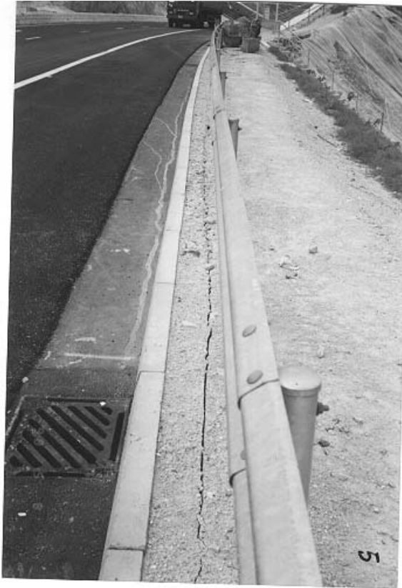
Plate 18 – Event No. 1: 4 May 1998. View North-East Along Crest of Slope A Indicating Cracking Behind Kerb Beam. (Photograph Taken on 8 May 1998)
