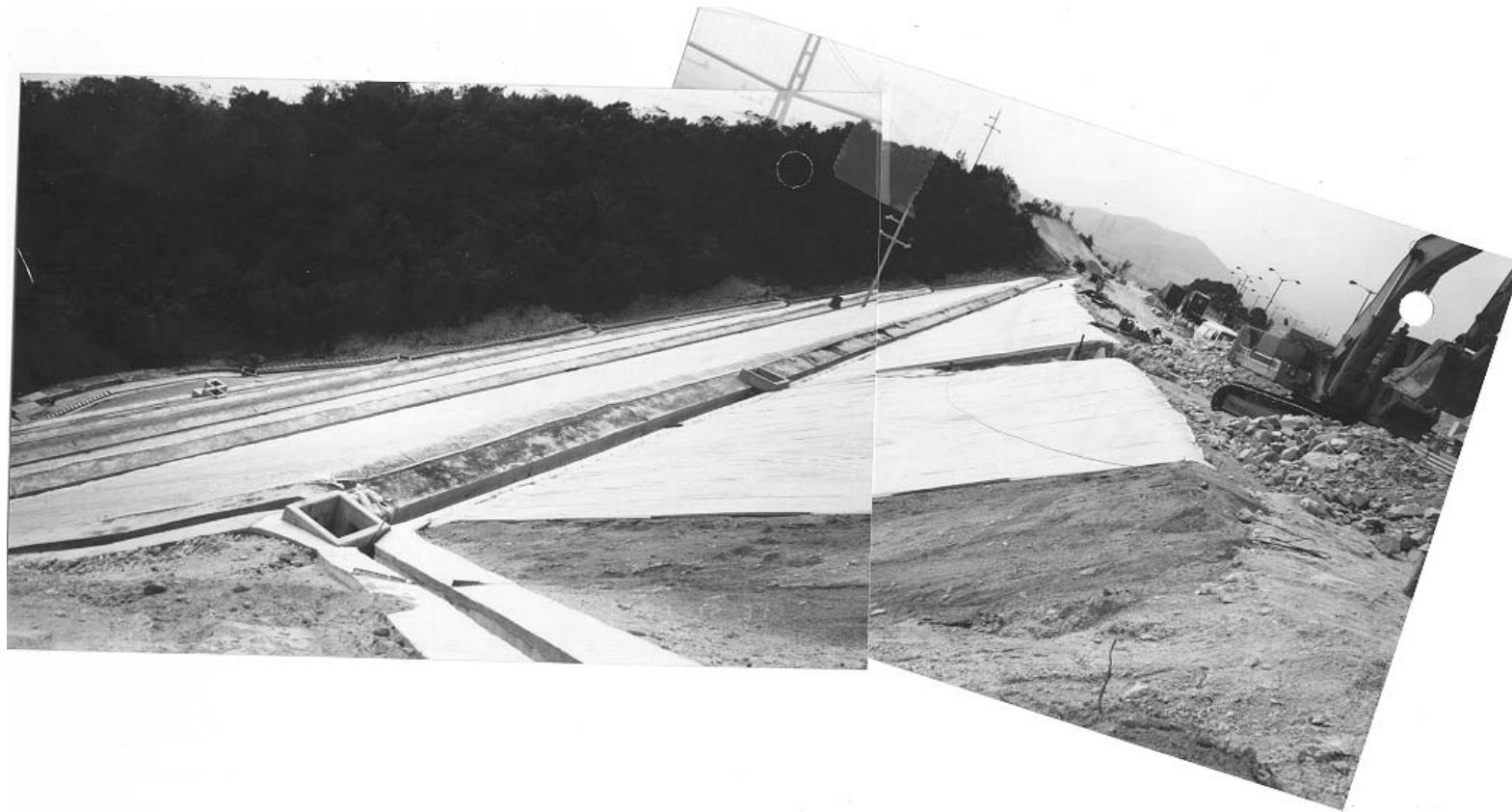
Plate 58 – View South Across Slope B Indicating Essentially Completed Slope Works. Drainage Works in Progress on Upper Batter. Similar Comment Regarding Exposed Horizontal Face of Landscaping Fill at Berm Level as for Plate 57. (Photograph Taken on 31 December 1997)
