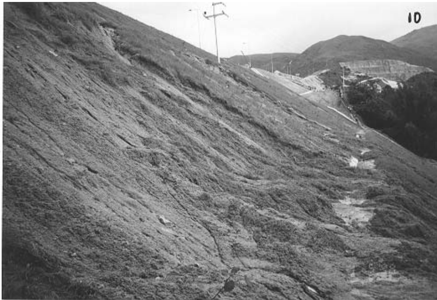
Plate 9 – Event No. 1: 4 May 1998. View North-East Along 52.5 mPD Berm from South End of Slope B Indicating Scars on Batter Above and Debris Deposition on Berm and Batter Below. (Photograph Taken on 4 May 1998)
