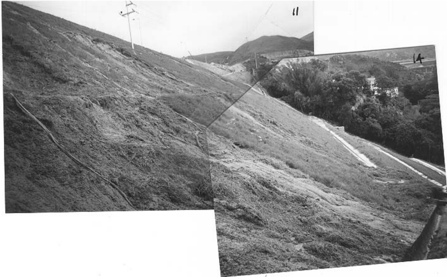
Plate 11 – Event No. 1: 4 May 1998. View North-East Along Batter Between 45 mPD and 52.5 mPD Berms from South End of Slope B. Note accumulated Debris in Foreground, with Scar Extending from Batter Above 52.5 mPD Berm to 45 mPD Berm and Debris Accumulation on Berm. (Photograph Taken on 4 May 1998)
