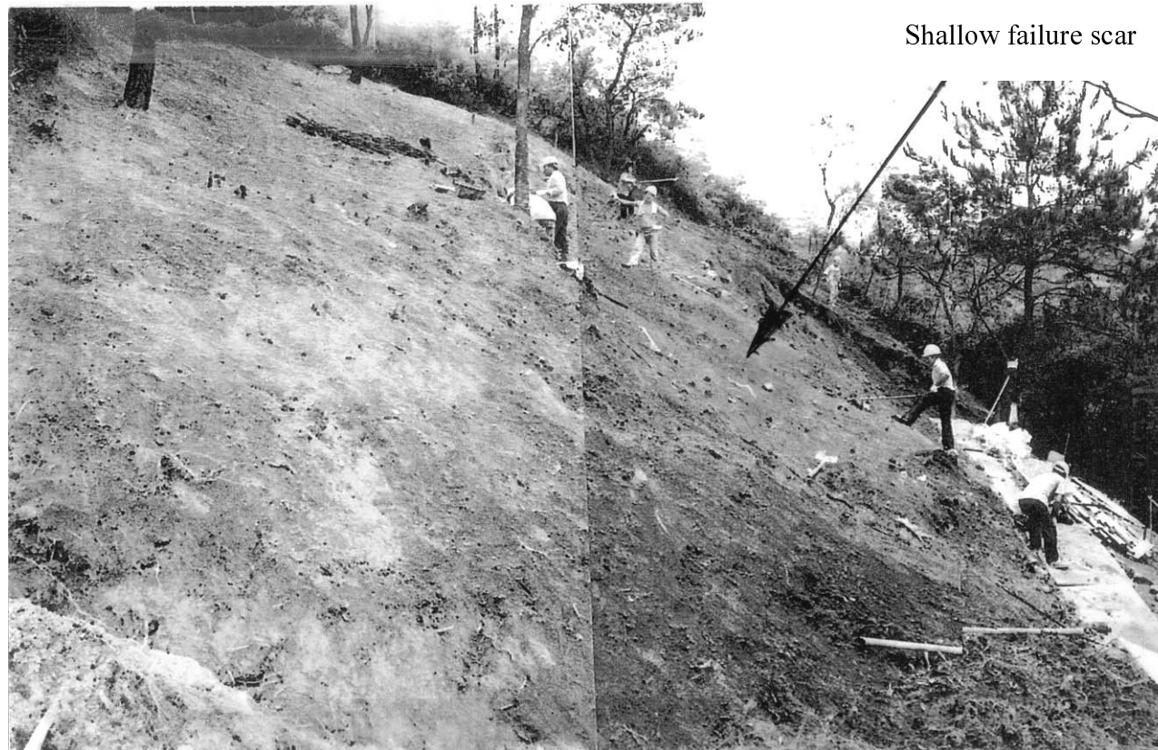
Plate 3 – View of Shallow Failure Scar Identified in the Hillside above Block 13 (Photographs taken on 29 April 1998)
